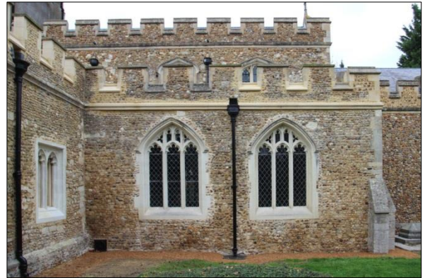
Plate 34: Finished works, south aisle (69)
