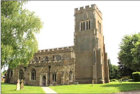
Plate 1: Initial survey, north elevation and tower (1)
