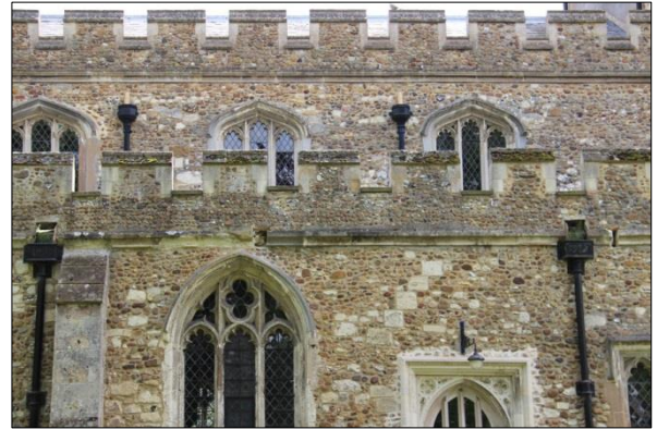
Plate 4: Initial survey, north aisle string course and parapets (4)
