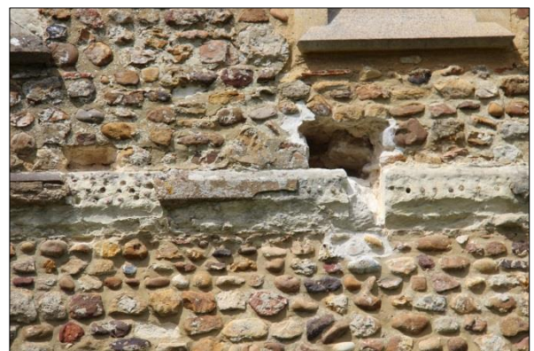
Plate 12: Initial survey, south aisle string course (28)
