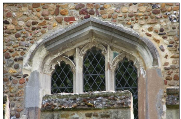
Plate 6: Initial survey, northeast clerestory window (9)
