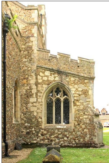
Plate 3: Initial survey, east elevation of north aisle (33)
