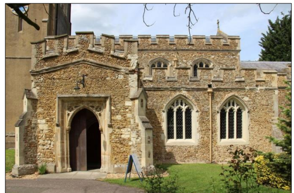
Plate 10: Initial survey, south aisle and porch (23)
