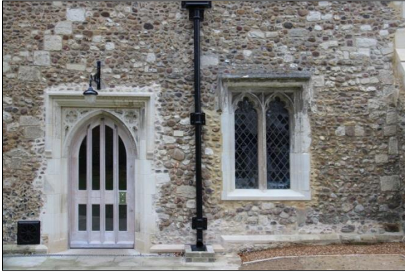
Plate 31: Finished works, repairs to doorway and window surround in north aisle (63)
