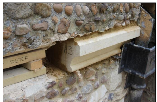
Plate 18: Watching brief, new Clipsham stone in north aisle string course (46)
