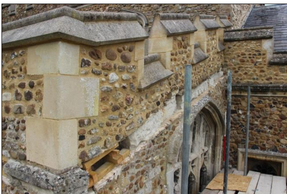
Plate 23: Watching brief, south aisle string course (57)
