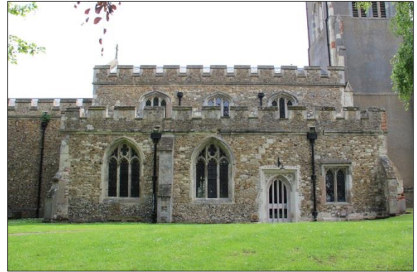
Plate 2: Initial survey, north elevation (2)
