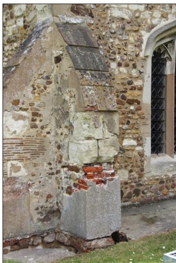
Plate 5: Initial survey, west buttresses of north aisle (11)
