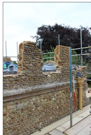
Plate 24: Watching brief, south porch stripped parapet wall (51)
