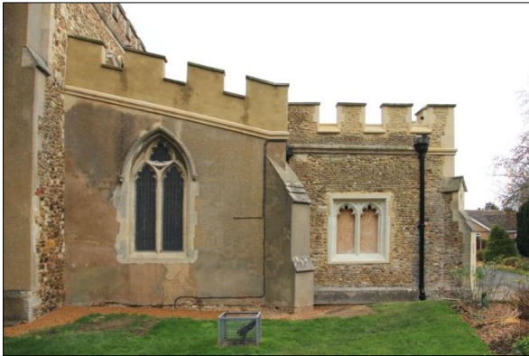
Plate 33: Finished works, west elevation of south aisle and porch (67)
