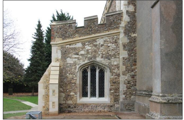
Plate 32: Finished works, west elevation of north aisle (65)
