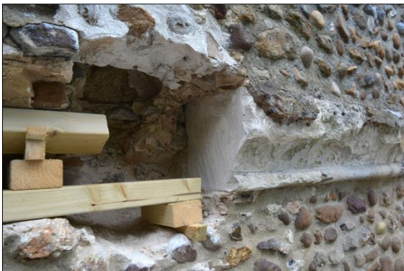
Plate 15: Watching brief, exposed clunch in north aisle string course (36)
