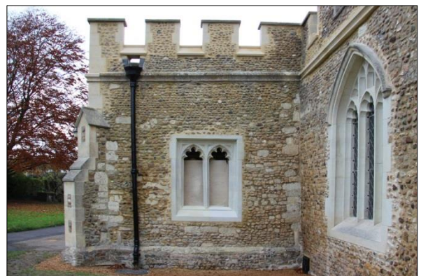
Plate 36: Finished works, east elevation of south porch (68)
