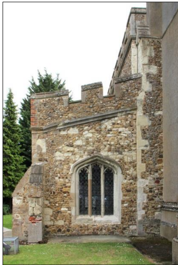
Plate 7: Initial survey, west elevation of north aisle (13)
