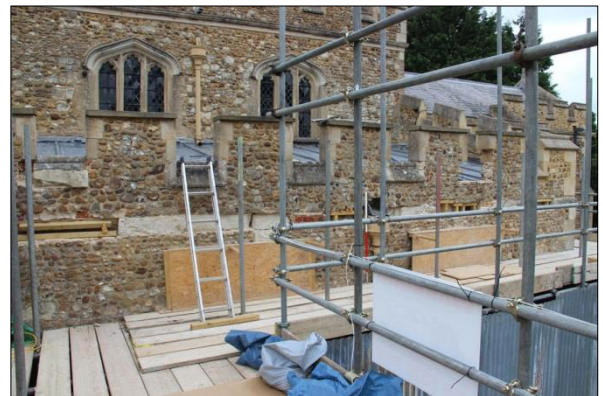
Plate 22: Watching brief, south aisle string course (56)
