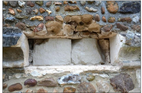
Plate 14: Watching brief, exposed clunch in north aisle string course (39)
