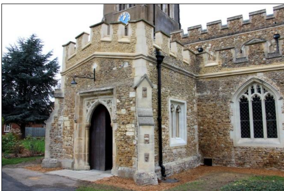
Plate 35: Finished works, south porch (70)
