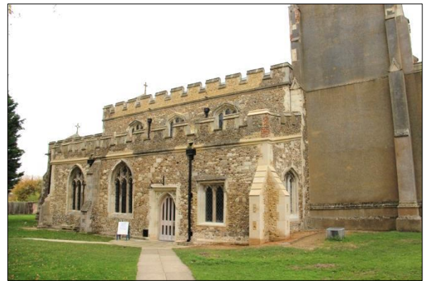
Plate 28: Finished works, north elevation (60)
