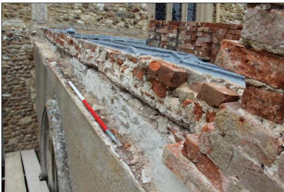
Plate 21: Watching brief, south aisle parapet wall removed (50)
