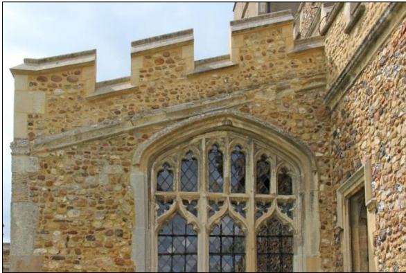
Plate 13: Initial survey, east elevation of south aisle (32)
