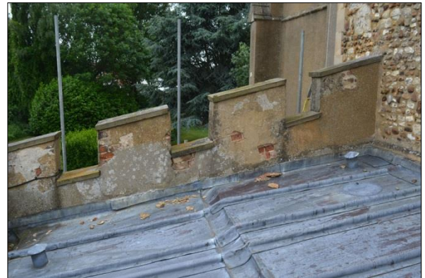
Plate 20: Watching brief, south aisle parapet wall (42)
