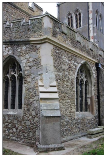
Plate 30: Finished works, east buttress of north aisle (73)
