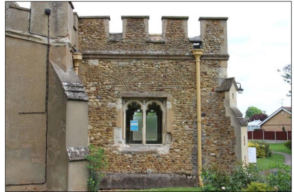
Plate 8: Initial survey, west elevation of south porch (16)
