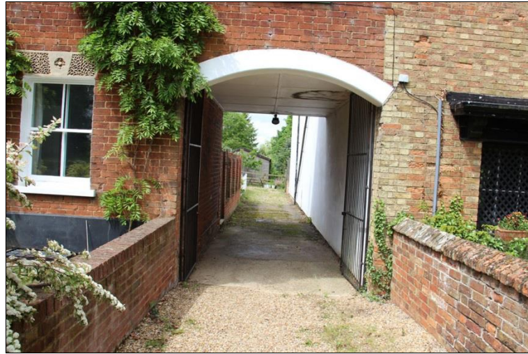
Plate 5: Carriageway and access to the proposed development site
