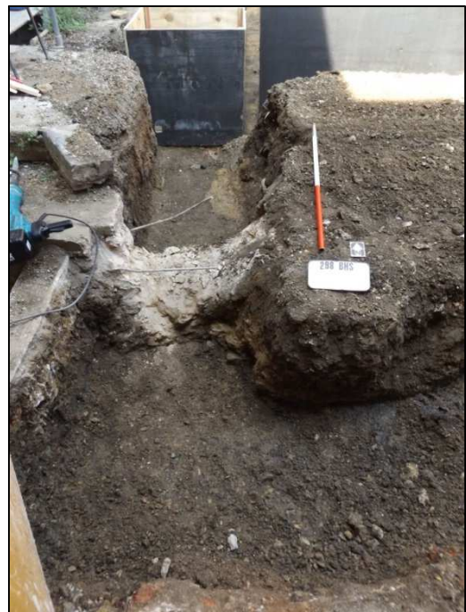
Plate 14: Western side of footing trench, looking N (1m scale)
