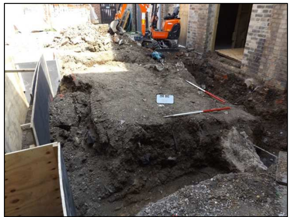
Plate 12: Footing trench, looking ESE (2x1m scale)
