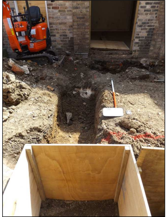
Plate 16: Eastern side of footing trench, looking S (1m scale)
