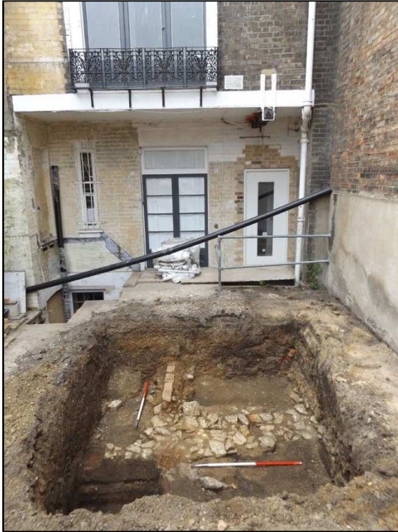
Plate 1: General shot of trench in relation to surrounding building, looking W (2x1m scale)
