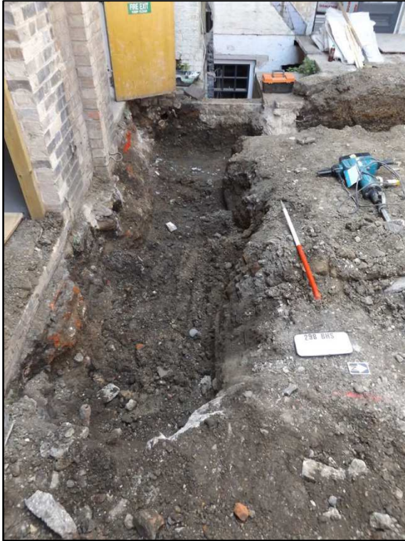
Plate 15: Southern side of footing trench, looking W (1m scale)
