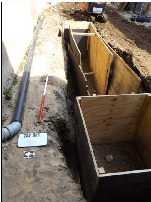
Plate 13: Northern side of footing trench, looking E (1m scale)
