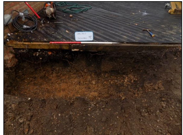
Plate 2: Northeast footing trench, facing northeast
