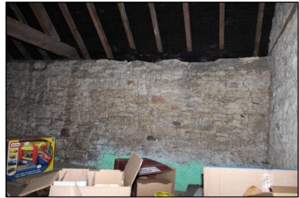
Plate 40: Shot 22. F1, west wall
