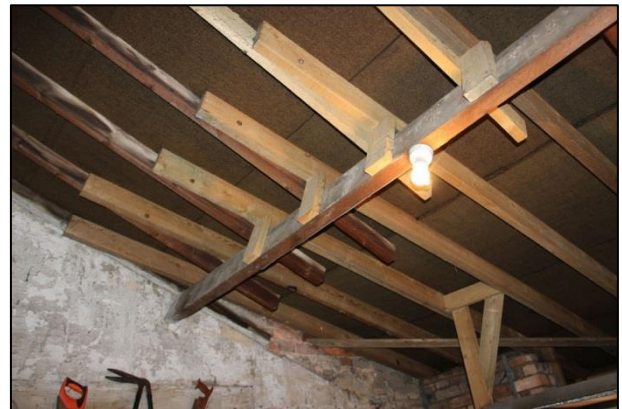
Plate 33: Shot 33. G2 roof detail
