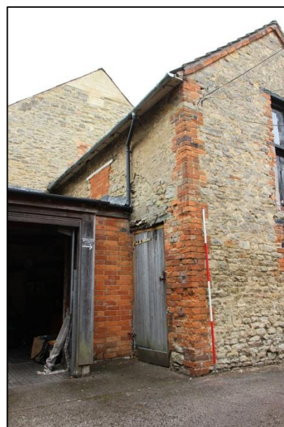
Plate 9: Shot 2. North elevation, door detail
