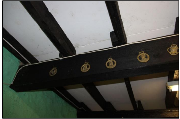
Plate 23: Shot 16. G1 beam detail
