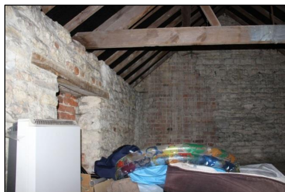
Plate 38: Shot 20. F1, northeast corner
