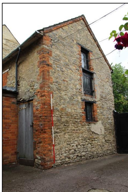
Plate 8: Shot 1. North elevation
