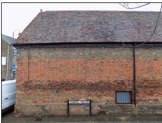
Plate 5: Old Maltings west elevation- south end
