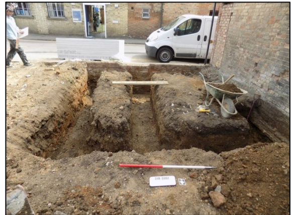
Plate 17: Building Foundation Trenches looking south
