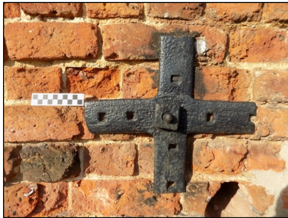
Plate 12: Cross anchor plate
