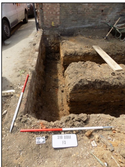
Plate 18: Building Foundation Trench 3 looking west
