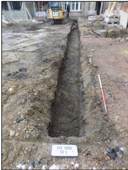
Plate 14: Wall Footing 1 looking north
