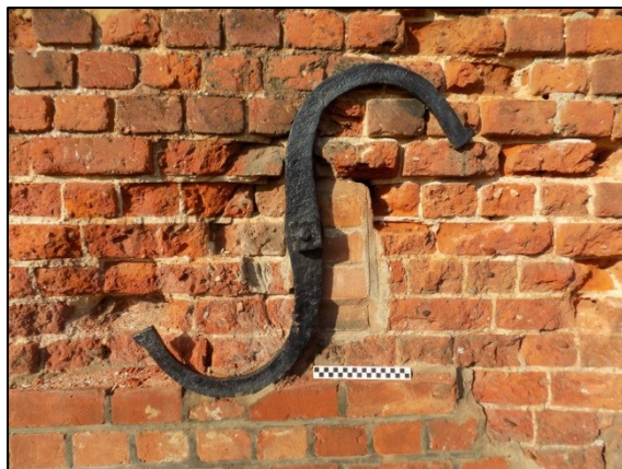
Plate 11: S Anchor plate
