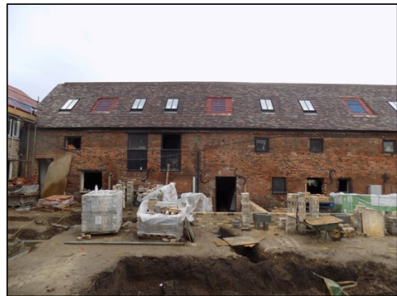
Plate 2: Old Maltings east elevation- north end
