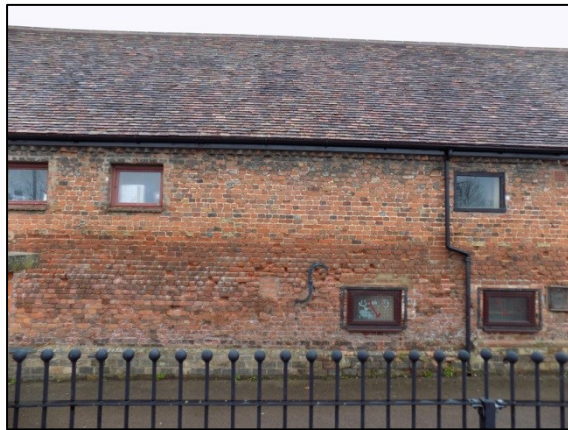
Plate 7: Old Maltings west elevation- south end moving north
