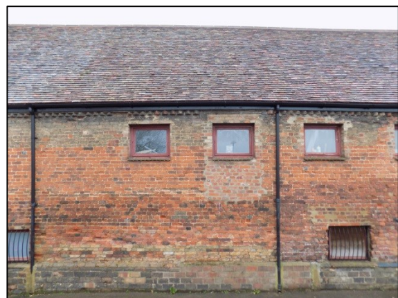
Plate 6: Old Maltings west elevation- south end moving north
