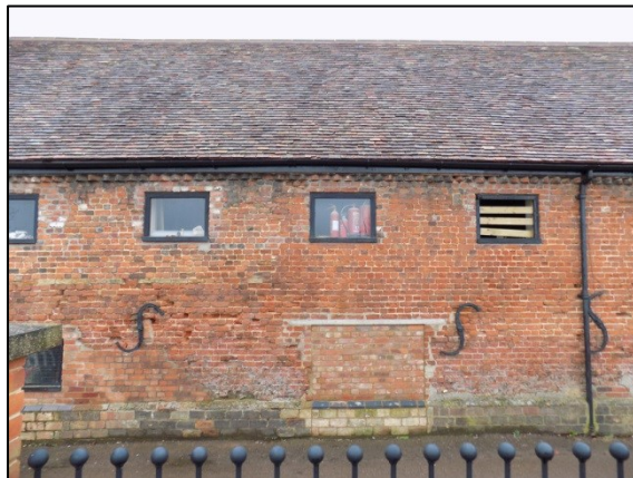
Plate 9: Old Maltings west elevation- north end moving north
