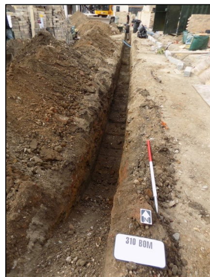
Plate 19: Service Trench 3 looking north
