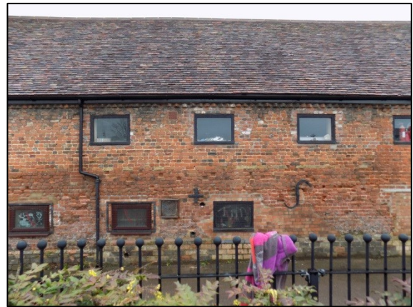
Plate 8: Old Maltings west elevation- middle section
