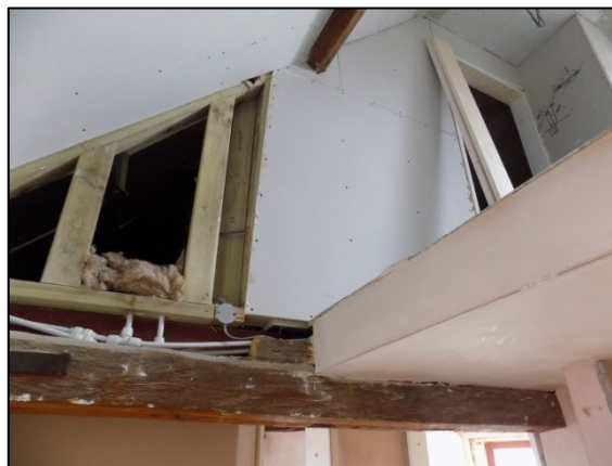
Plate 13: Tiebeam with newly added upper floor, looking northeast
