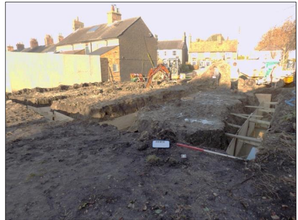
Plate 14: Overall shot of footing trenches, view north-northeast
