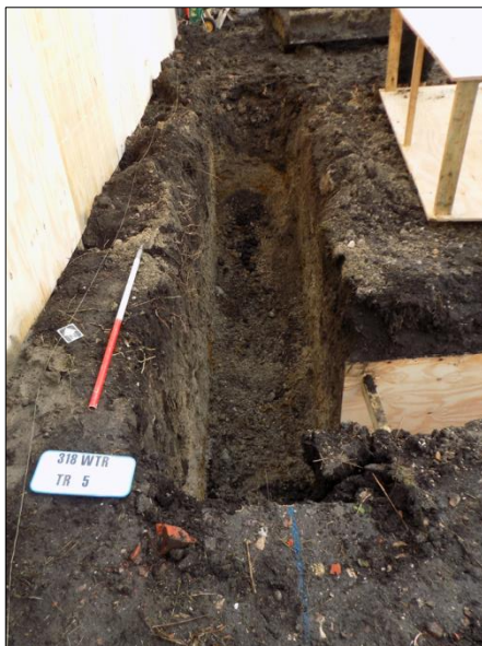
Plate 9: Trench 5, view northeast
