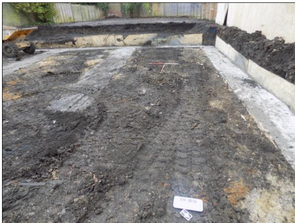
Plate 15: Footprint with footings present and ground levelled, view southwest
