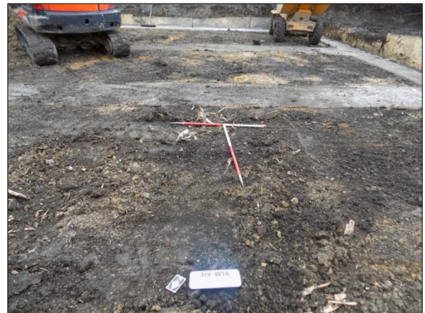
Plate 16: Footprint with footings present and ground levelled, view southeast
