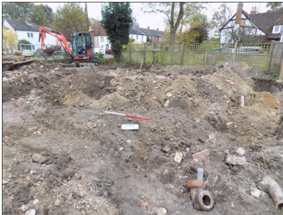
Plate 1: Overall shot during removal of original footings
