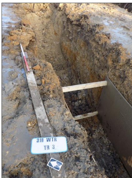
Plate 5: Trench 3, view east-northeast
