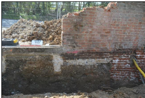
Plate 6: West wall foundation, looking west
