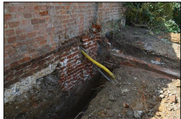
Plate 7: West wall foundation showing return, Looking northwest
