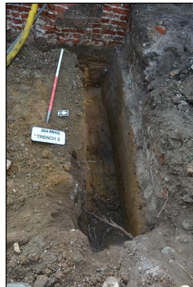
Plate 2: Footing 2, looking west
