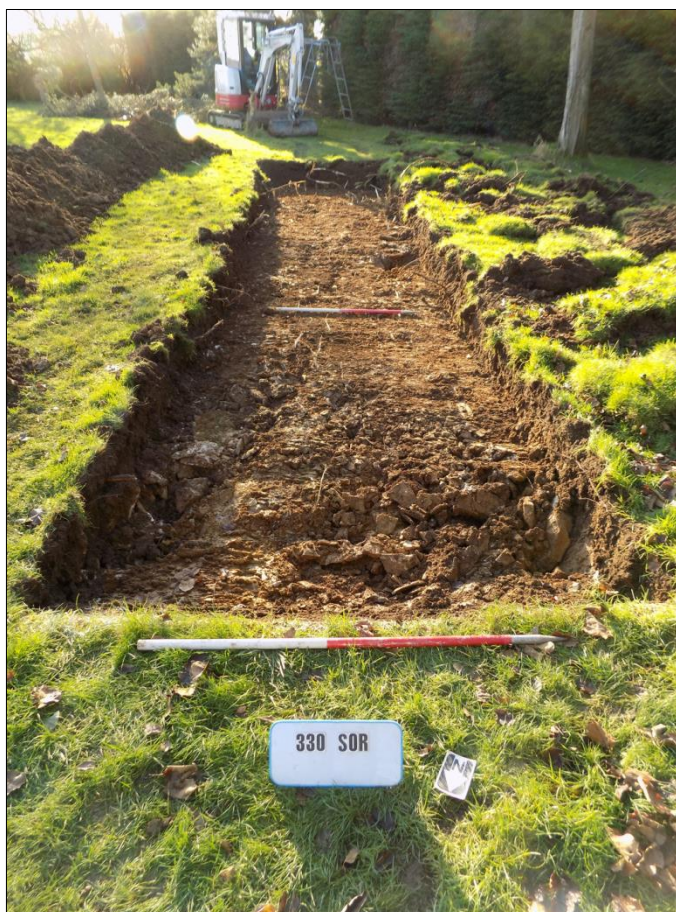
Plate 1: Overall trench shot, facing south
