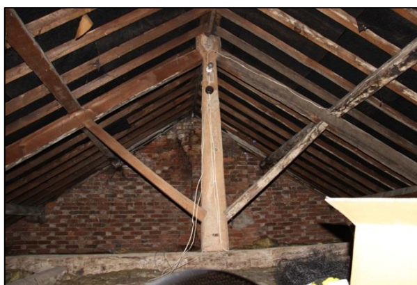
Plate 60: Shot 58. King posts in loft, looking north
