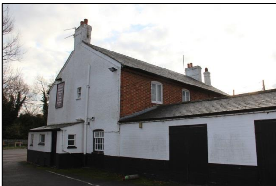
Plate 8: Shot 9: North & west elevations, main building
