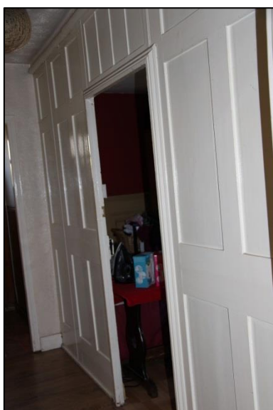
Plate 48: Shot 46. F6 corridor, partition wall
