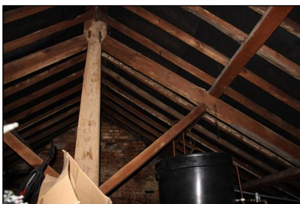
Plate 58: Shot 56. King posts in loft, looking south
