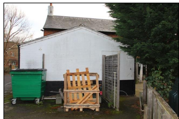
Plate 9: Shot 6. West elevation of extension
