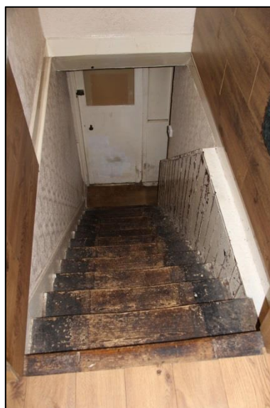
Plate 35: Shot 55. F1 Staircase, looking east
