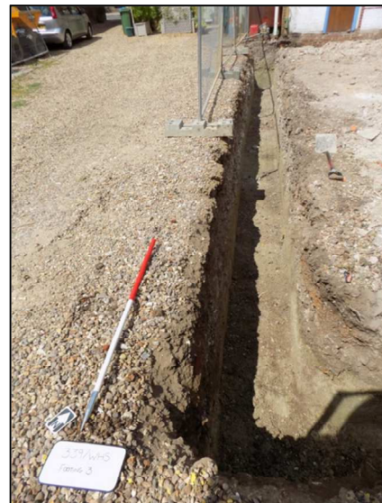
Plate 4: Footing 3, looking NNW
