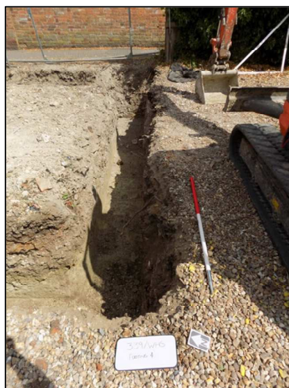
Plate 5: Footing 4, looking ENE
