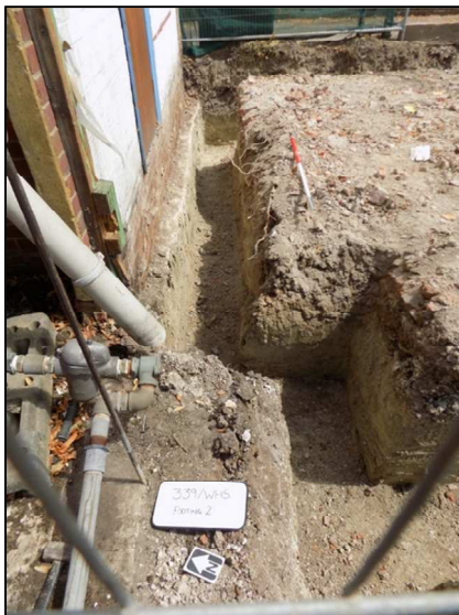
Plate 3: Footing 2, looking ENE
