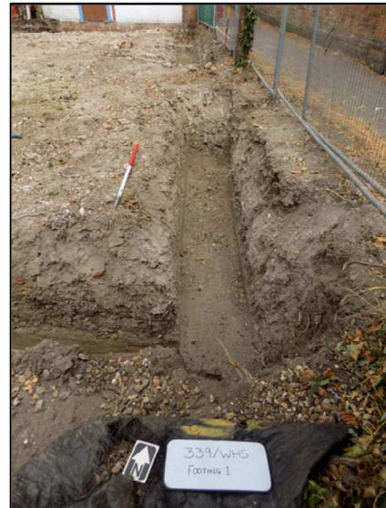
Plate 2: Footing 1, looking NNW
