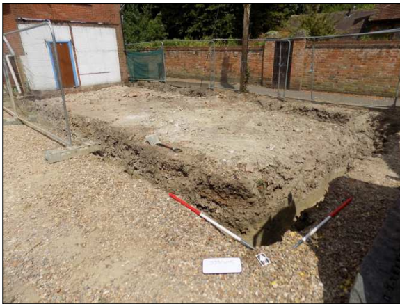
Plate 1: Completed footings, looking NNE
