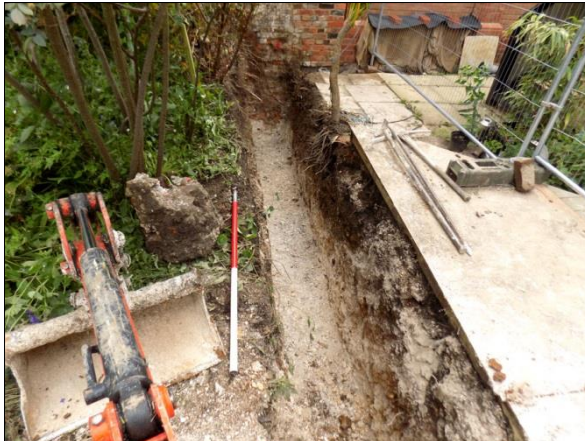
Plate 1: Wall footing trench, view N
