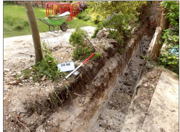
Plate 2: Wall footing trench, view SE
