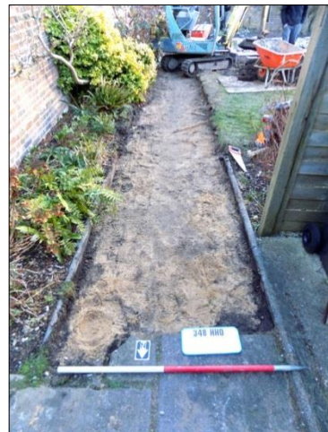
Plate 8: Path slab removal, view SSE
