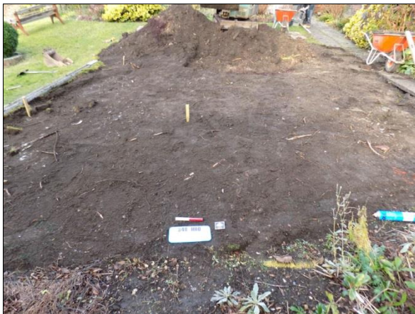
Plate 7: Patio ground reduction, view NNW
