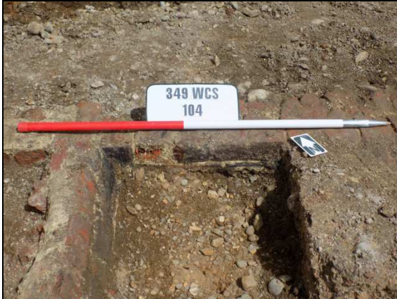
Plate 13: Southwest facing section of [104] northeast wall
