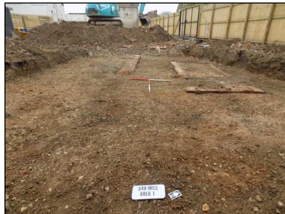
Plate 2: Area 1 looking northwest
