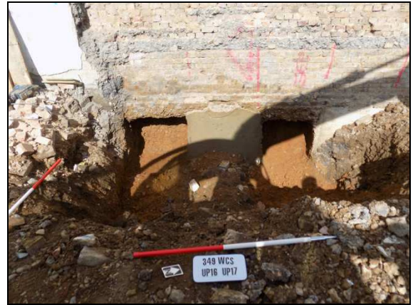
Plate 44: Underpinning pits 16 and 17 looking west northwest
