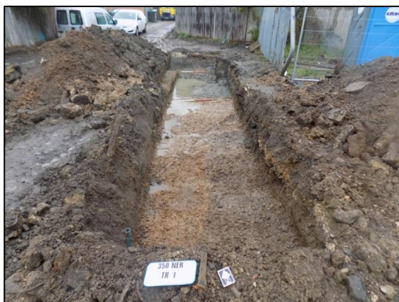
Plate 3: Trench 1 looking north northeast
