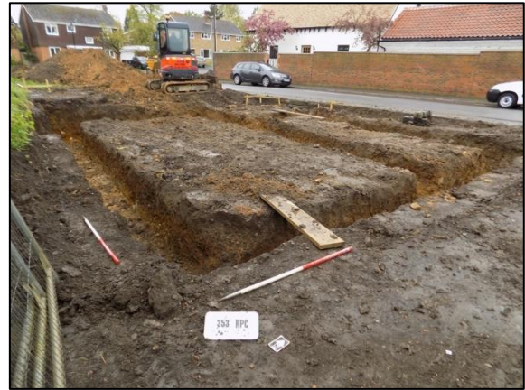
Plate 2: Footing trenches, general shot, looking WNW (2x1m scale)
