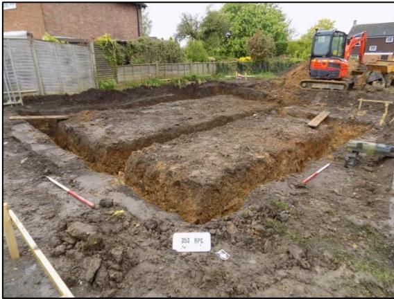
Plate 1: Footing trenches, general shot, looking SSW (2x1m scale)
