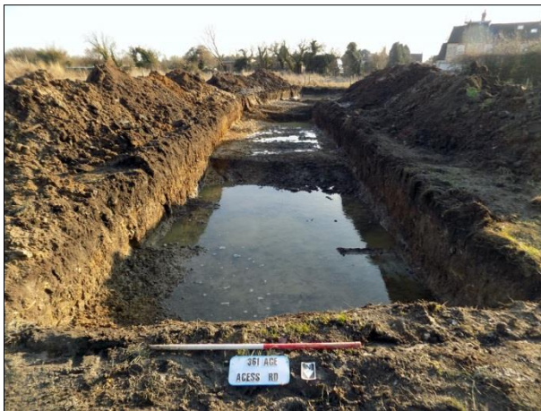
Plate 1: Access Road trench, facing south
