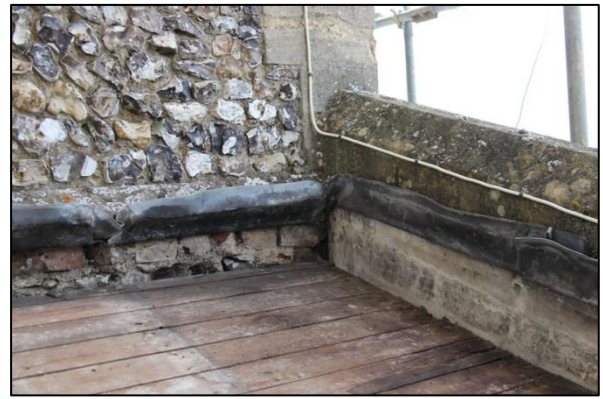
Plate 14: Brickwork in the nave wall over the north aisle roof
