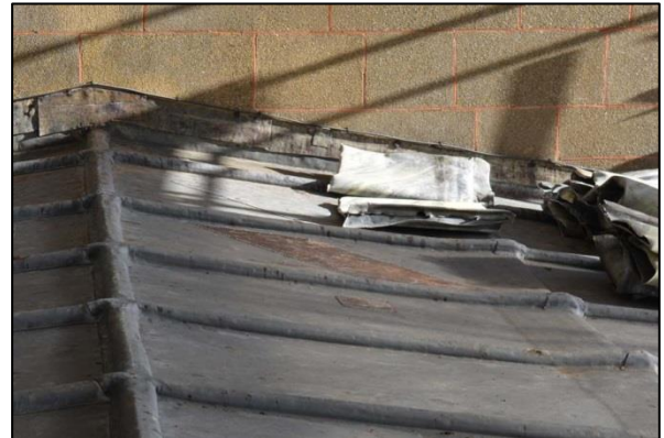
Plate 8: Example of a historic roof repair
