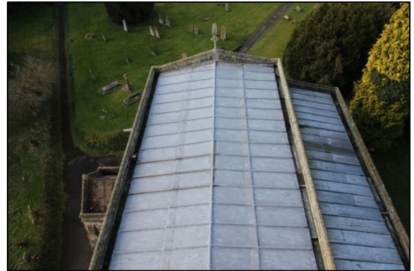
Plate 2: Nave and north aisle roofs from the east
