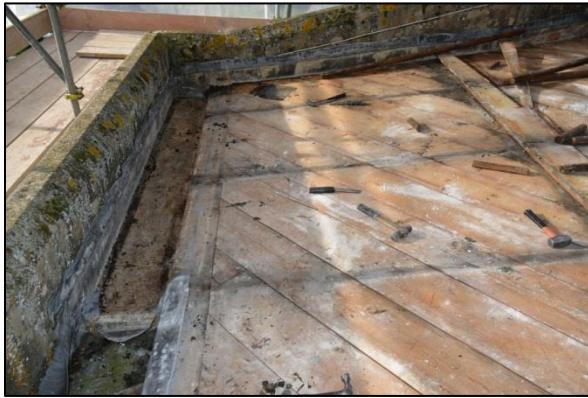
Plate 7: Nave roof timbers and valley gutter detail
