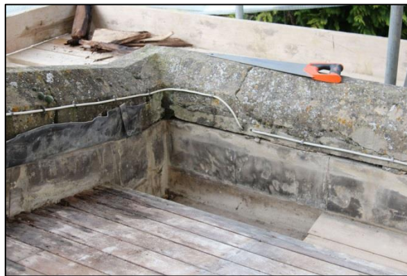
Plate 15: Blockwork in the south and west walls of the north aisle
