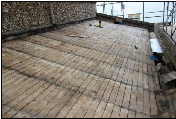
Plate 13: North aisle roof timbers looking west
