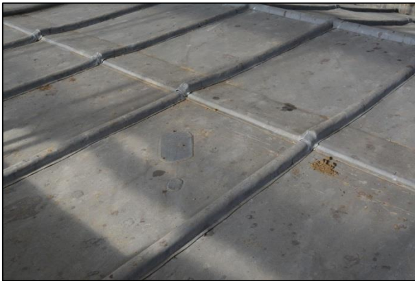
Plate 9: Patch repair at the eastern end of the nave roof
