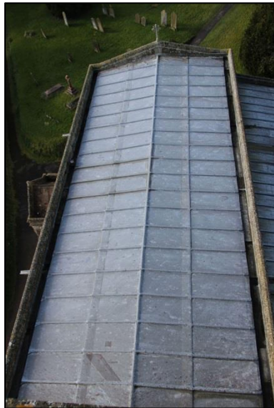
Plate 3: Nave roof before works commenced
