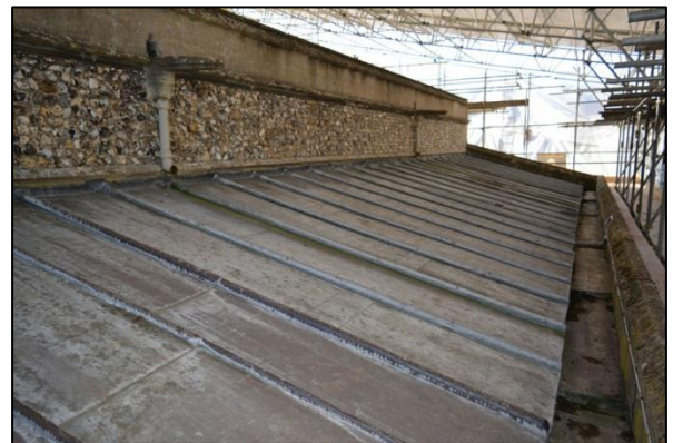
Plate 4: North aisle roof from the northeast before works commenced
