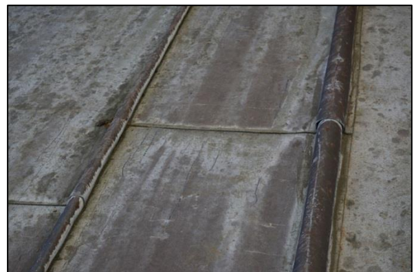
Plate 6: Hollow roll to the left of a timber roll joint
