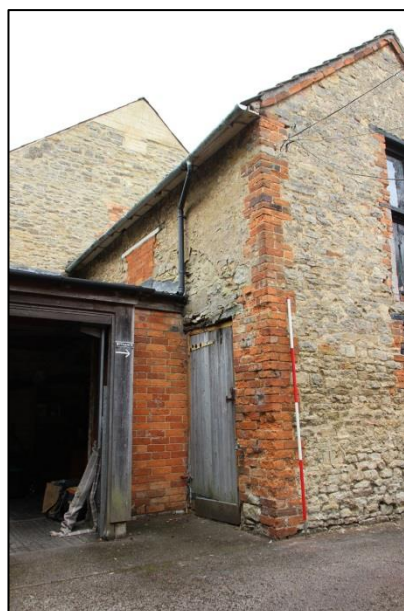
Plate 9: Shot 2. North elevation, door detail
