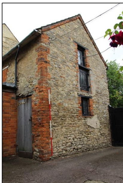
Plate 8: Shot 1. North elevation
