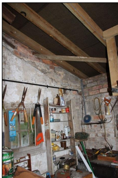
Plate 34: Shot 34. G2, northwest corner showing garage heightening
