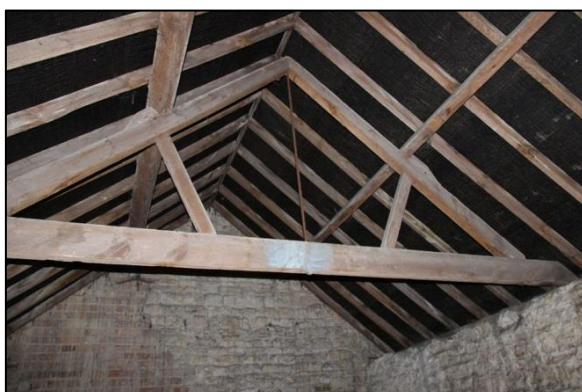
Plate 35: Shot 17. F1, Roof detail
