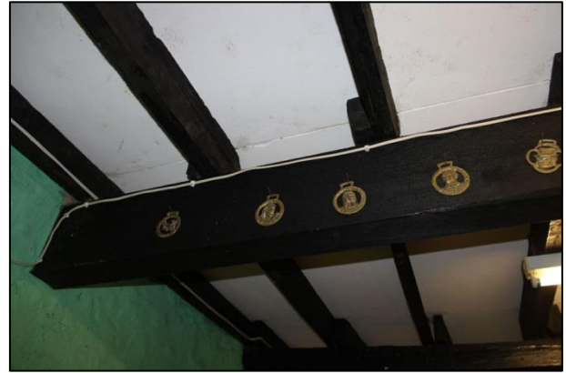
Plate 23: Shot 16. G1 beam detail
