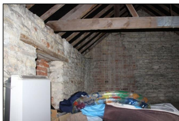
Plate 38: Shot 20. F1, northeast corner
