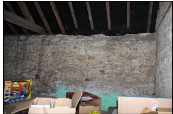
Plate 40: Shot 22. F1, west wall
