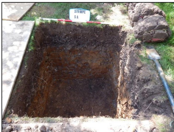
Plate 5: Soakaway, looking south southeast
