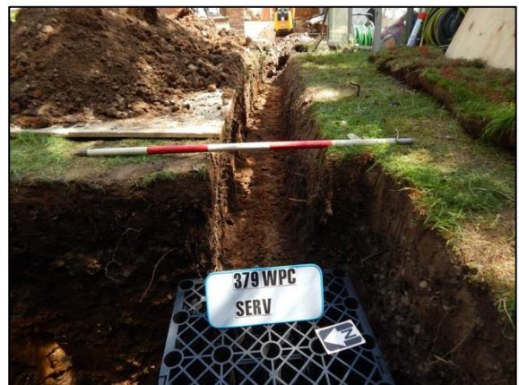
Plate 6: Service trench, looking east southeast
