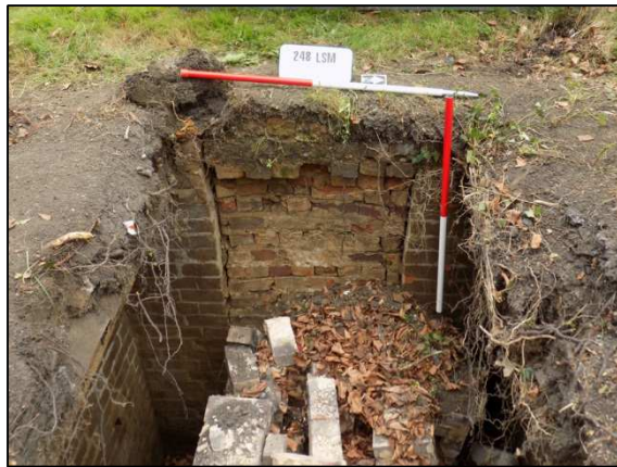
Plate 13: Bricked up vault entrance looking west
