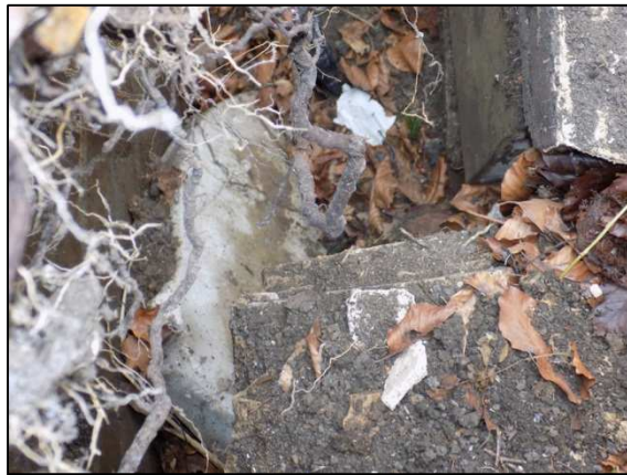
Plate 15: Displaced gravestone close up looking east
