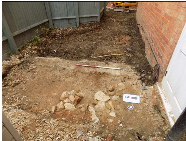
Plate 1: Ground reduction, looking NW (1m scale)
