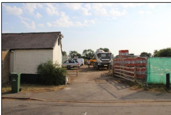
Plate 4: Access from Hartwell Road into current building site, looking northeast
