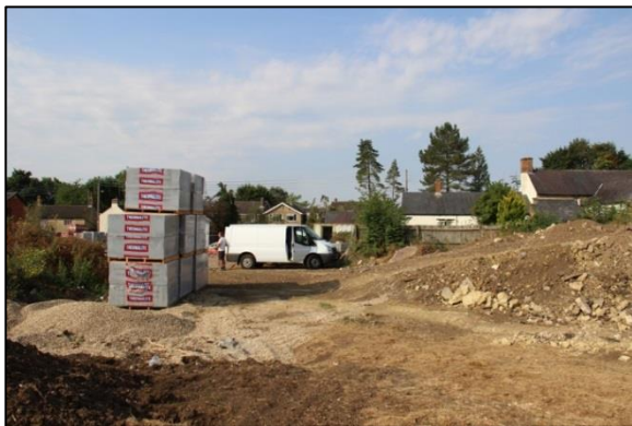
Plate 6: Proposed access road looking southwest
