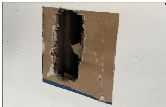
Plate 21: Ceiling to the rear of the shop
