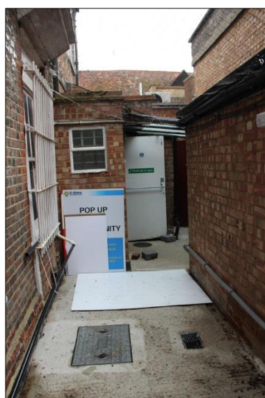
Plate 4: View into the yard from the passage
