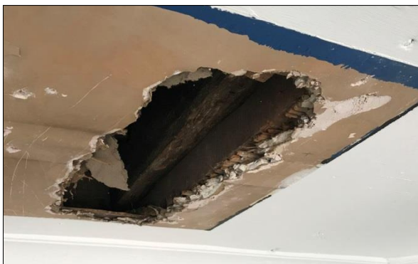
Plate 20: Ceiling to the front of the shop
