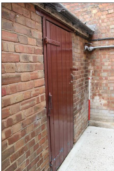
Plate 16: WC in the rear yard
