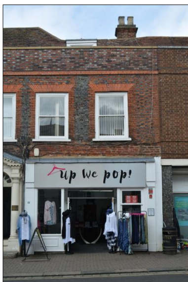
Plate 2: Detail of shop frontage
