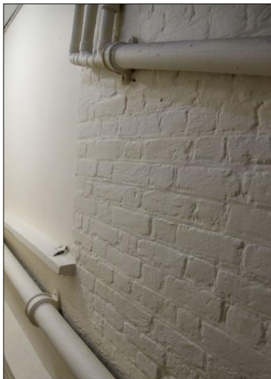
Plate 14: Blocked window detail
