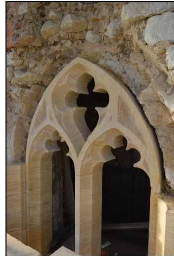
Shot 68: East elevation Stage 4 new window
