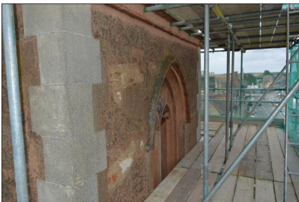
Shot 35: North elevation Stage 4
