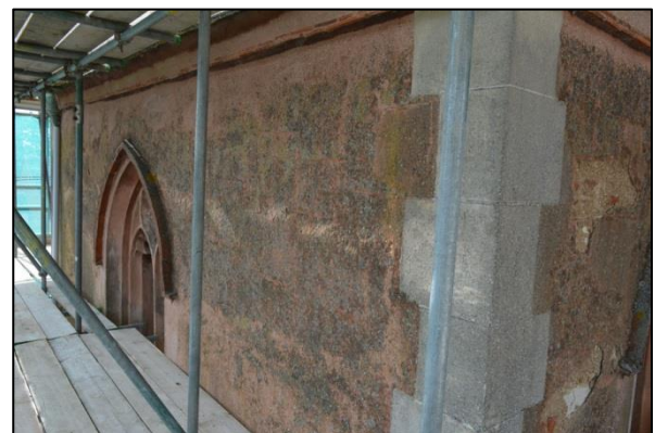
Shot 28: East elevation Stage 4
