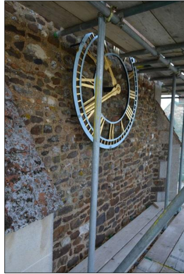
Shot 13: North elevation Stage 2
