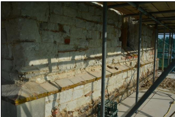
Shot 62: West elevation Stage 3
