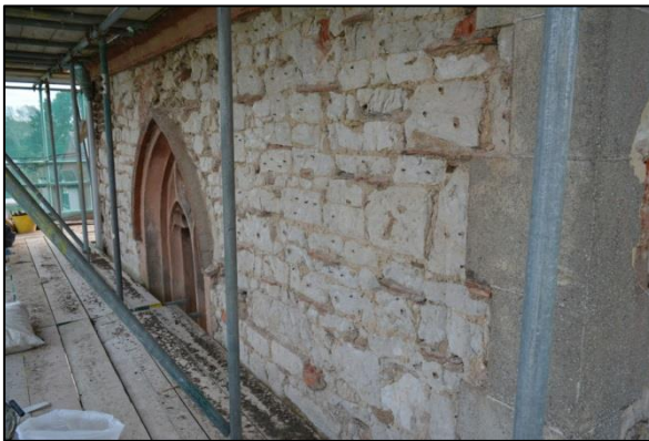
Shot 44: East elevation Stage 4
