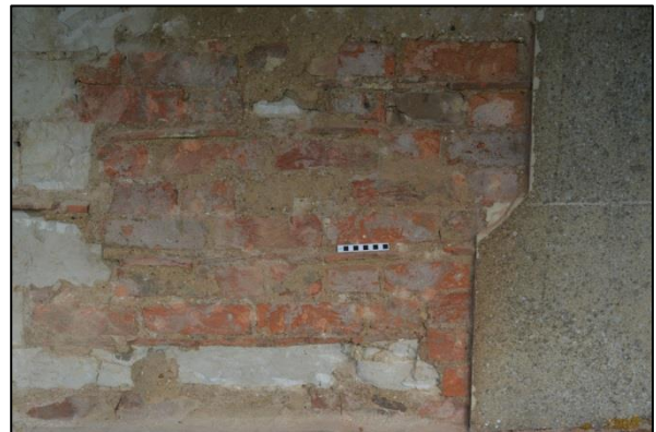
Shot 61: West elevation Stage 3, wall detail
