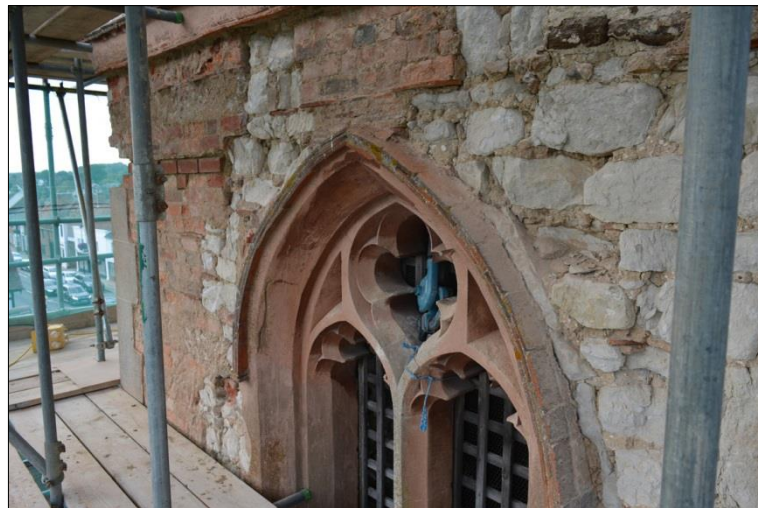
Plate 15: South elevation: upper level from the east
