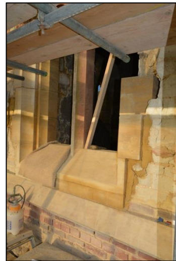
Shot 71: South elevation Stage 3
