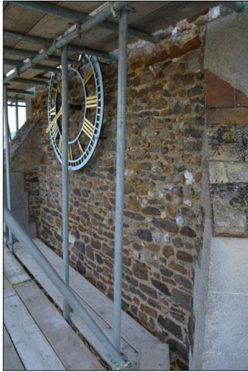
Shot 12: North elevation Stage 2
