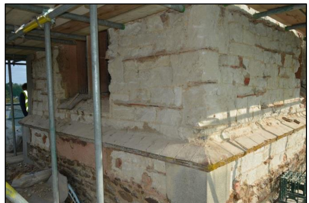
Shot 55: North elevation Stage 3
