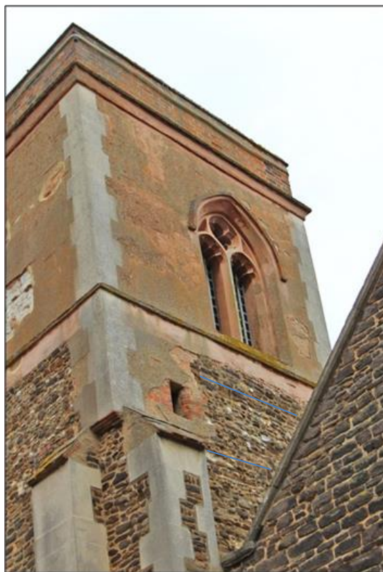
Plate 7: Repairs to the southwest corner
