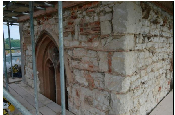
Shot 43: North elevation Stage 4
