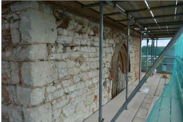
Plate 20: West elevation: upper level from the north
