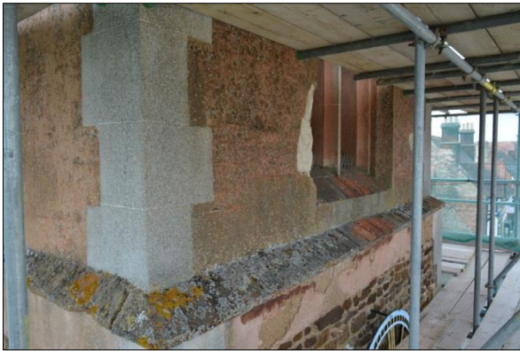
Shot 25: North elevation Stage 3
