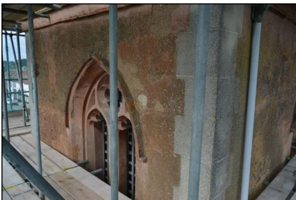
Shot 32: South elevation Stage 4
