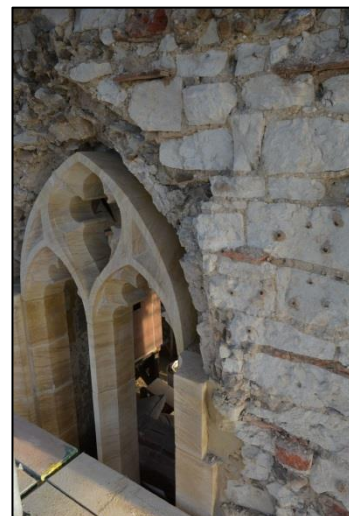
Shot 72: West elevation Stage 4
