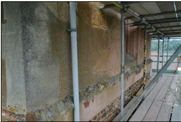
Shot 18: East elevation Stage 3
