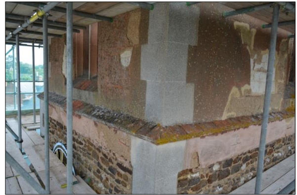
Shot 26: North elevation Stage 3
