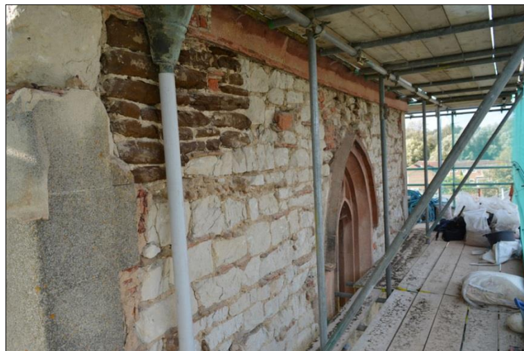
Plate 11: East elevation looking northwest
