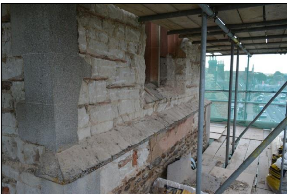
Shot 54: North elevation Stage 3
