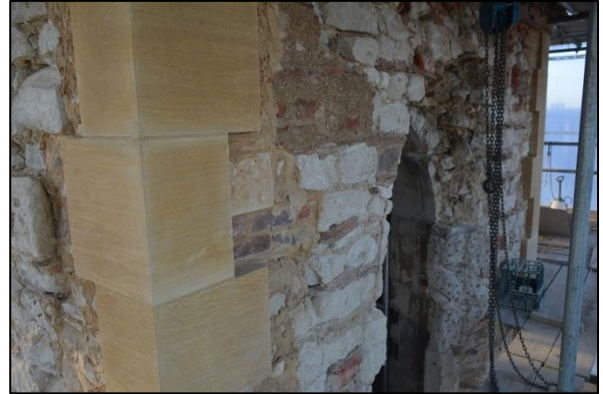
Shot 66: North elevation Stage 4, view to west
