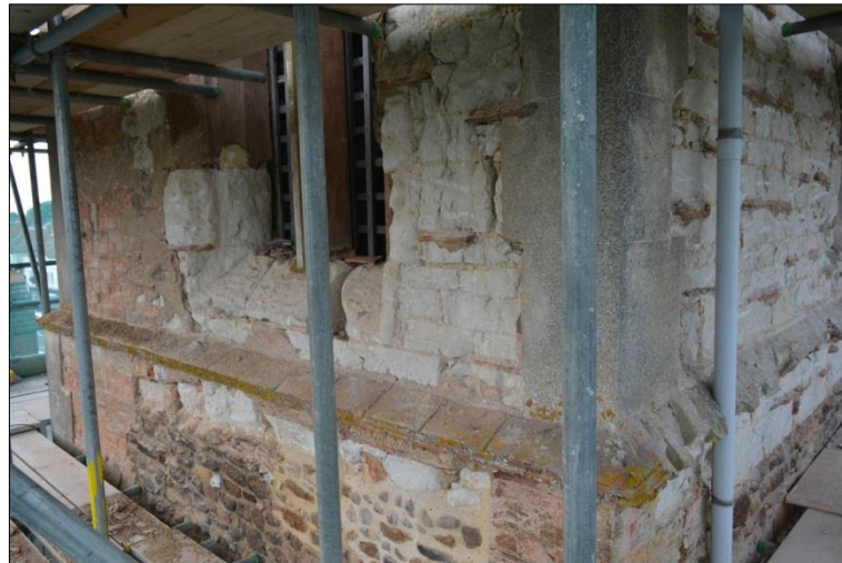
Plate 17: South elevation: lower level from the east
