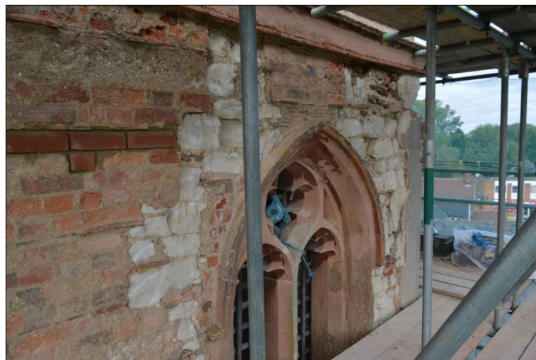
Plate 16: South elevation: upper level from the west
