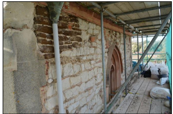
Shot 45: East elevation Stage 4
