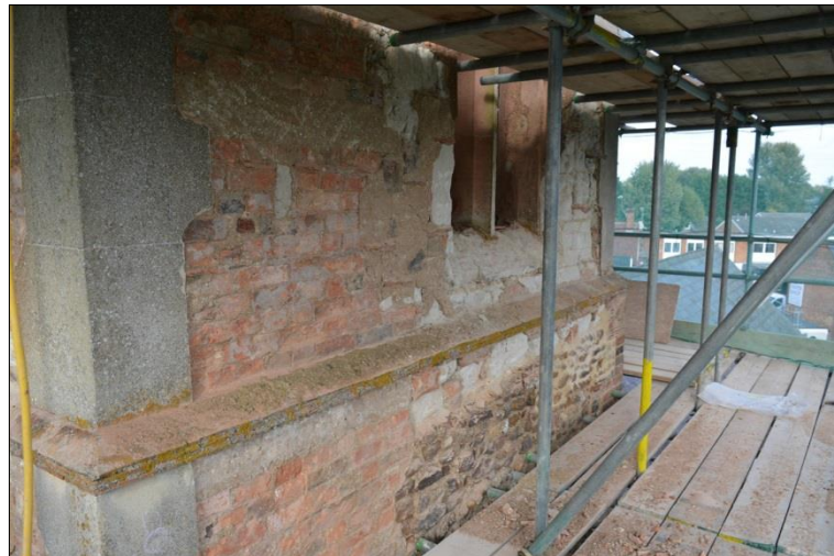
Plate 18: South elevation: lower level from the west
