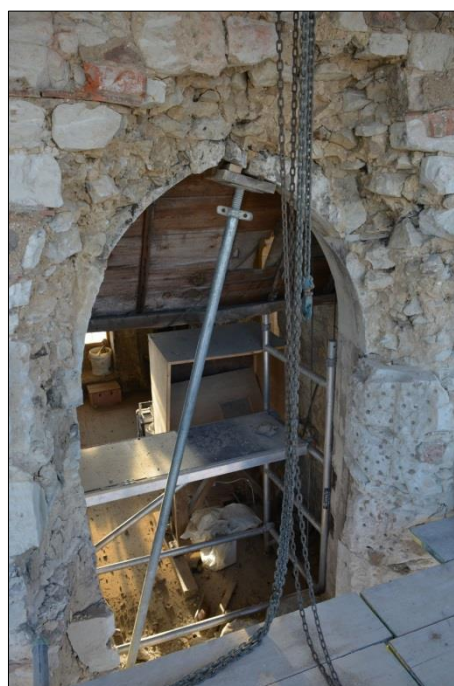
Plate 10: North window opening
