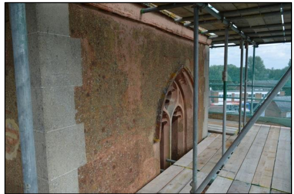
Shot 31: South elevation Stage 4
