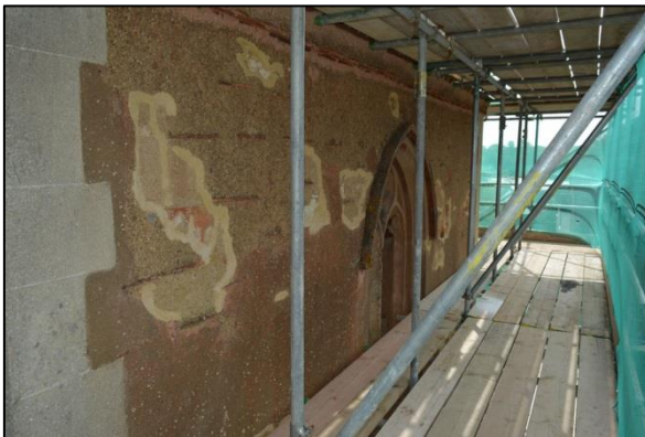
Shot 33: West elevation Stage 4
