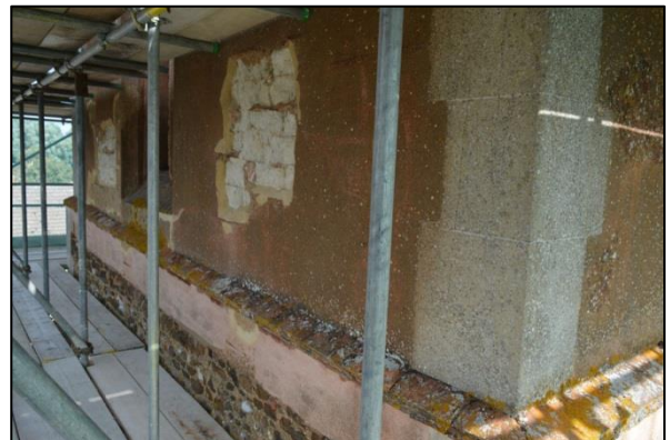
Shot 24: West elevation Stage 3
