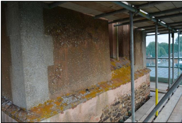
Shot 20: South elevation Stage 3
