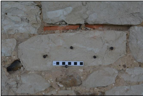
Shot 48: East elevation Stage 4, nails set into clunch
