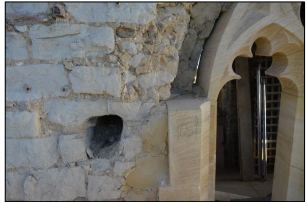
Shot 74: West elevation Stage 4, putlog hole
