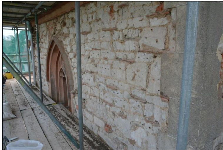
Plate 12: East elevation looking southwest
