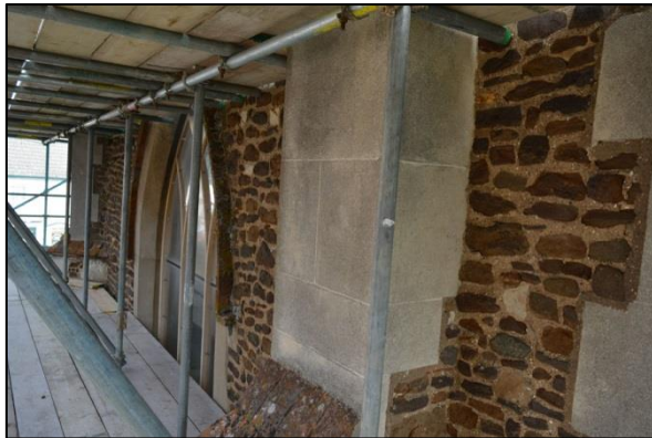
Shot 6: West elevation Stage 1
