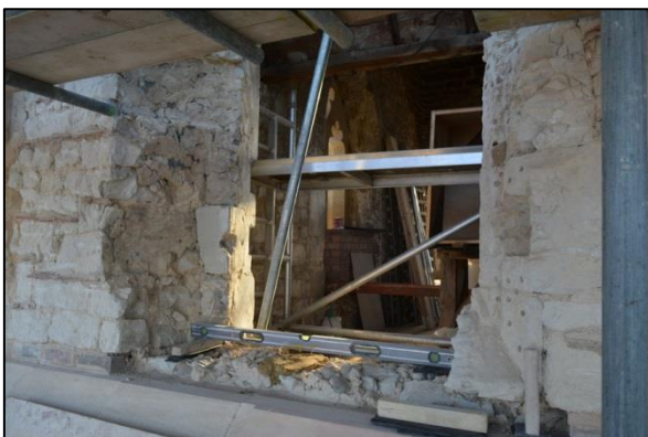
Shot 79: North elevation Stage 3, window detail
