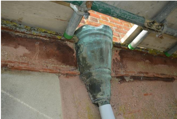
Shot 29: East elevation Stage 4, hopper & string course detail
