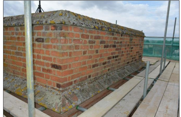
Shot 39: North elevation Stage 5, view to west
