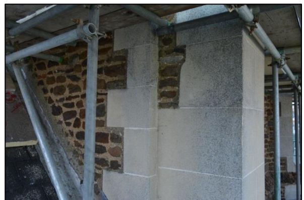
Shot 9: East elevation Stage 1
