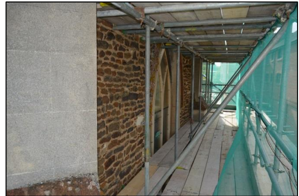
Shot 7: West elevation Stage 1
