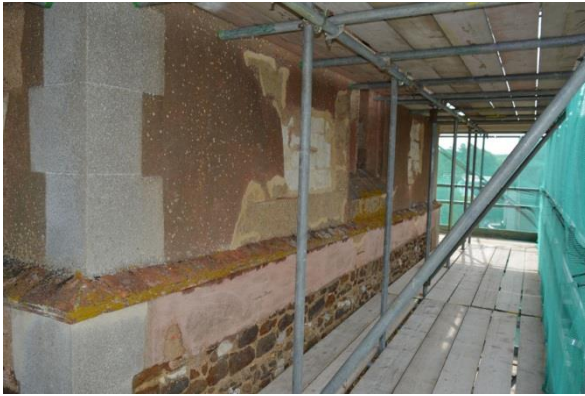
Shot 23: West elevation Stage 3
