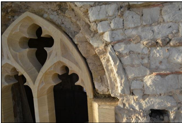
Shot 69: East elevation Stage 4, clunch hoodmould
