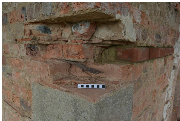
Plate 19: South elevation: iron work within southwest corner
