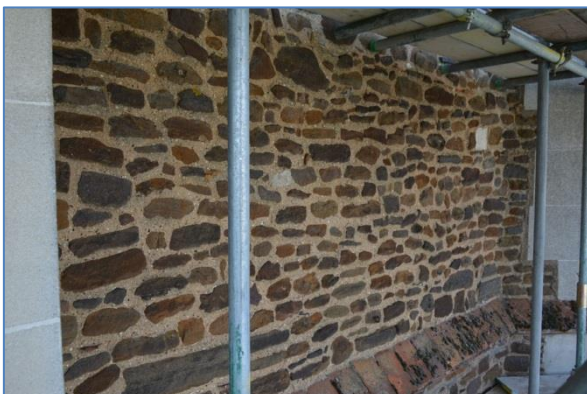
Shot 5: North elevation Stage 1
