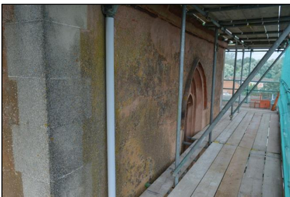
Shot 27: East elevation Stage 4
