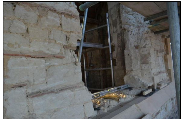
Shot 788: North elevation Stage 3, window detail
