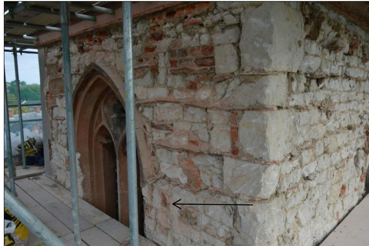
Plate 8: North and west elevations, upper level putlog hole indicated by arrow
