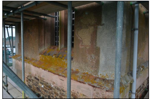
Shot 21: South elevation Stage 3
