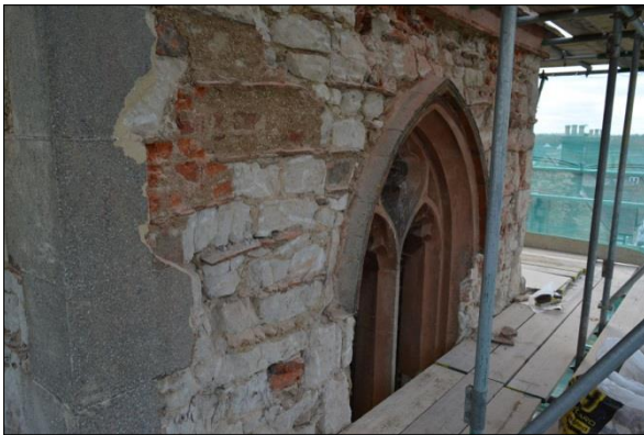
Shot 42: North elevation Stage 4
