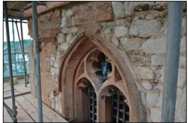
Shot 49: South elevation Stage 4
