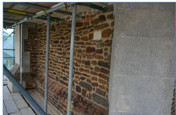
Shot 8: North elevation Stage 1
