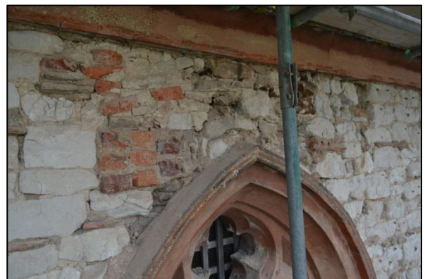
Shot 47: East elevation Stage 4, walling detail
