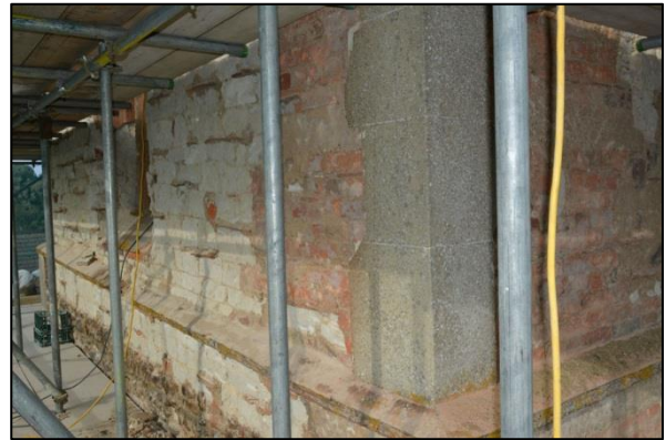
Shot 60: West elevation Stage 3
