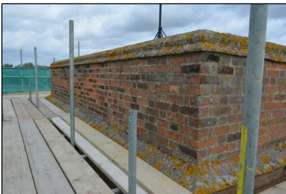
Shot 41: West elevation Stage 5
