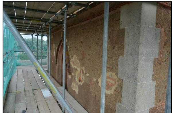
Shot 34: West elevation Stage 4
