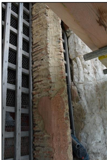
Shot 64: West elevation Stage 3 mullion detail
