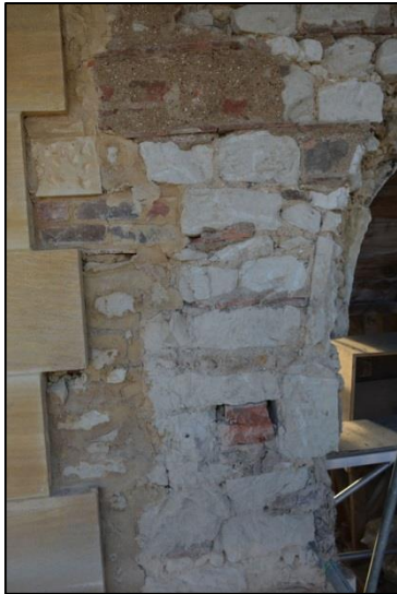
Shot 67: North elevation Stage 4, wall detail
