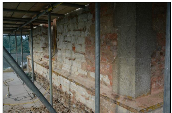
Shot 51: West elevation Stage 4
