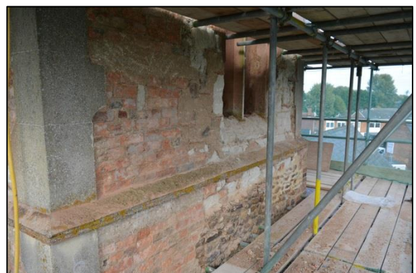
Shot 59: South elevation Stage 3
