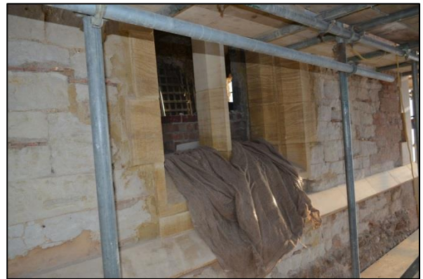
Shot 85: West elevation Stage 3
