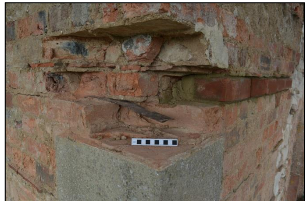
Shot 52: South west corner Stage 4 repair detail
