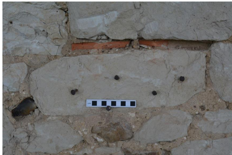
Plate 13: Detail of tile insert above and nails inside clunch piece
