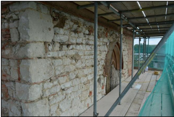
Shot 53: West elevation Stage 4
