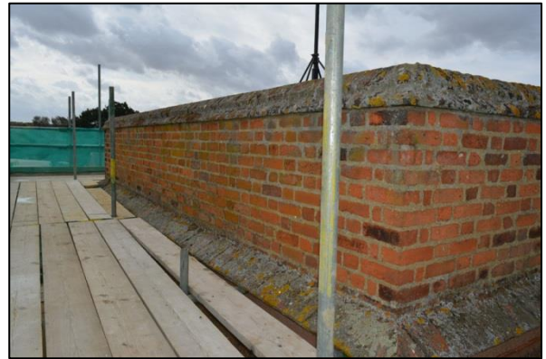
Shot 38: East elevation Stage 5
