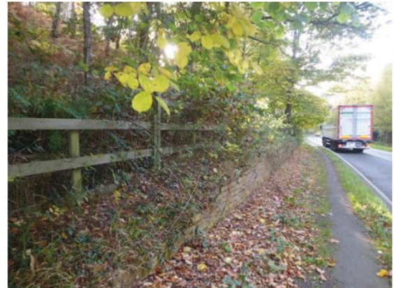
Figure 5 (right): An upstanding stretch of the remains of the wall in the combe
