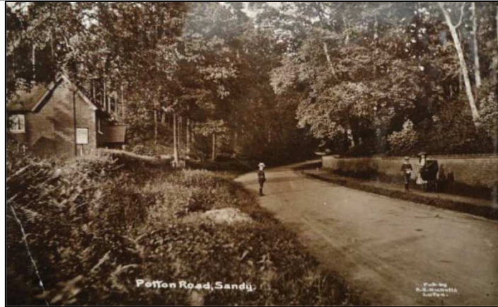
Figure 3: Postcard that includes the brick wall along the south side of the road to Potton
