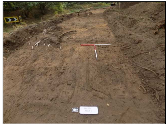
Plate 2: Area 2, looking east
