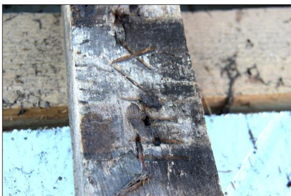
Plate 17: West range roof, east side: carpenters' marks (10)
