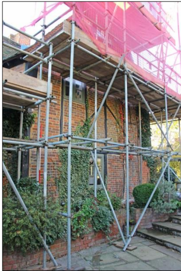
Plate 1: North elevation, west range (1)
