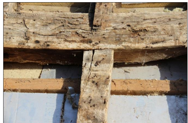
Plate 12: West range roof, west side: carpenters' marks (25)
