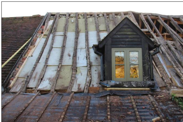
Plate 21: East range roof, north side (40)
