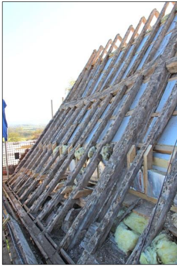
Plate 13: West range roof, east side (33)
