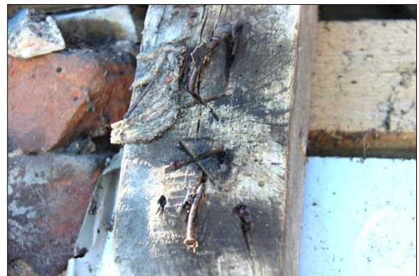
Plate 16: West range roof, east side: carpenters' marks (9)
