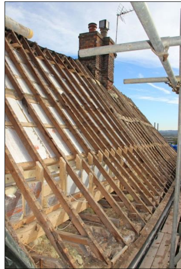
Plate 8: West range roof, west side (23)
