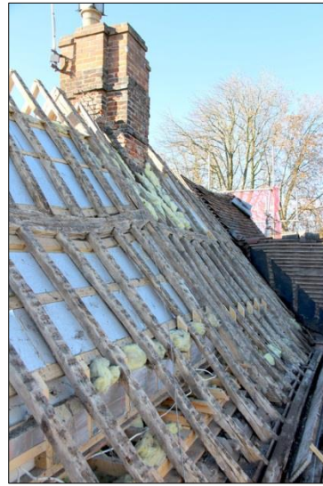
Plate 14: West range roof, east side (32)
