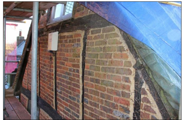
Plate 4: North elevation, west range, upper level (6)
