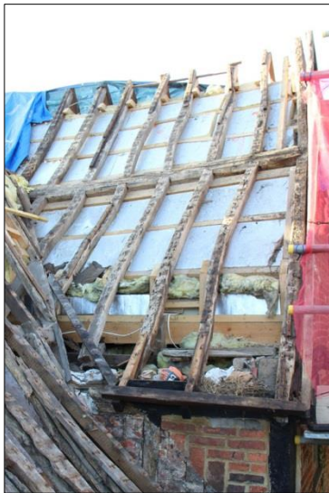
Plate 15: West range roof, east side (42)
