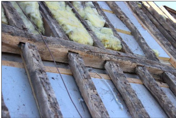
Plate 19: West range roof, east side: central tenon joints, one with a spurred face shoulder to the left, between purlin and common rafters (36)
