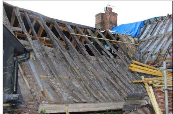
Plate 22: East range roof, north side (39)
