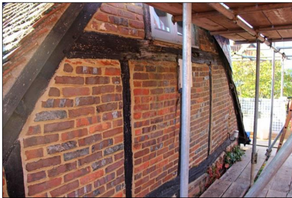
Plate 3: North elevation, west range, upper level (5)
