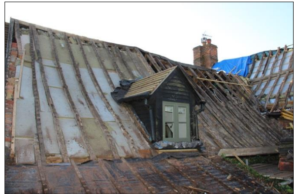
Plate 20: East range roof, north side (41)
