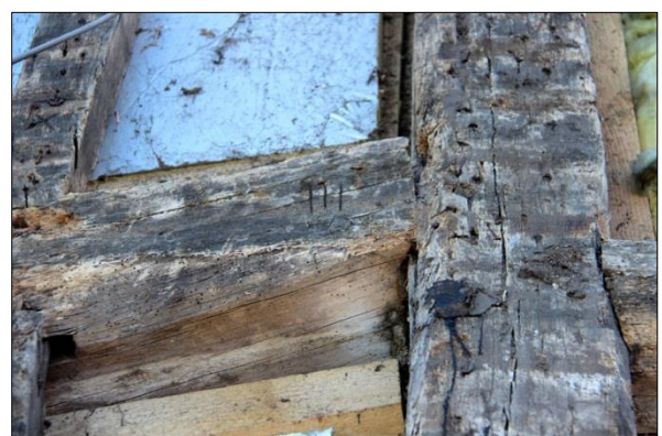
Plate 18: West range roof, east side: carpenters' marks (37)
