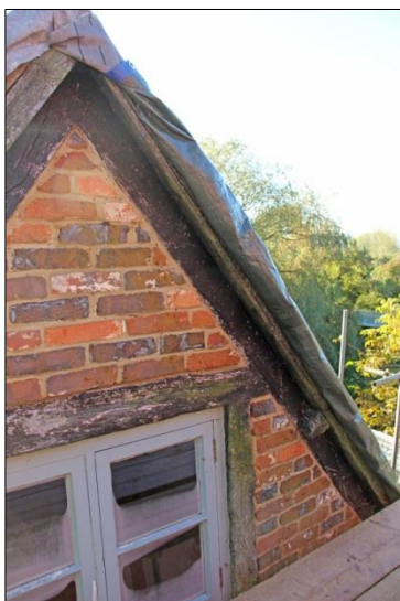
Plate 5: North elevation, west range, upper level (8)
