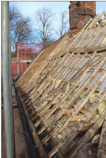
Plate 9: West range roof, west side (22)
