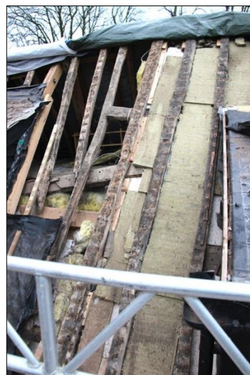
Plate 24: East range roof, south side (44)
