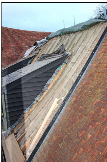
Plate 23: East range roof, south side (43)
