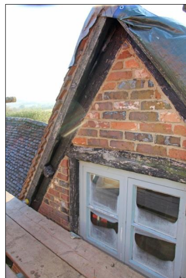
Plate 6: North elevation, west range, upper level (7)
