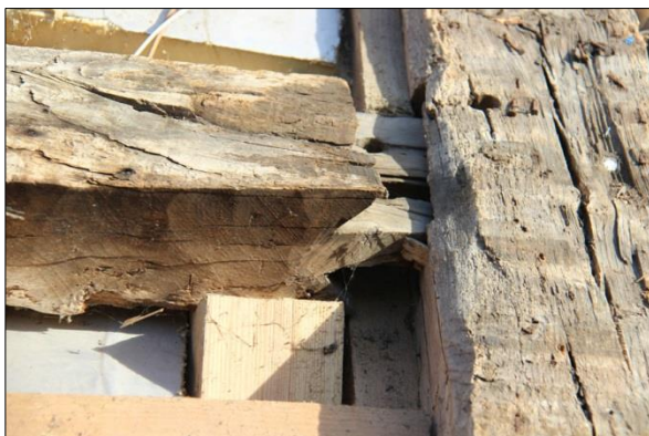
Plate 11: West range roof, west side: central tenon with spurred shoulders between purlin and principal rafter (31)
