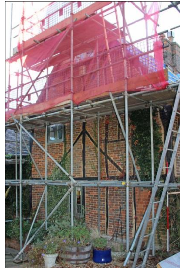
Plate 2: North elevation, west range (2)
