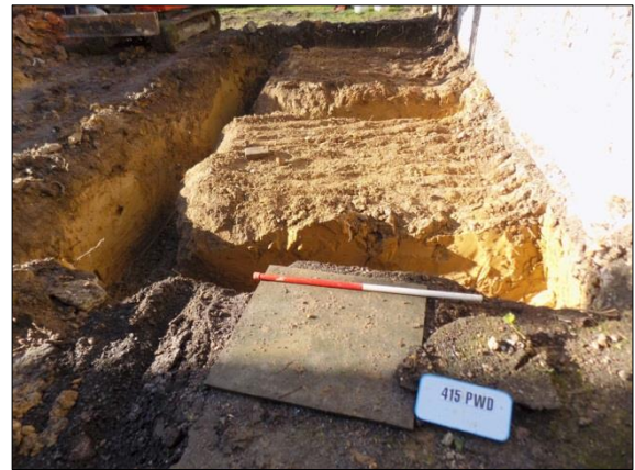
Plate 2: Footings and ground reduction, view WSW
