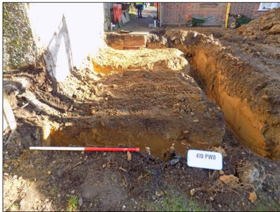
Plate 1: Footings and ground reduction, view ENE
