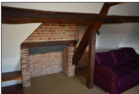
Plate 113: Room S4: fireplace detail (92)
