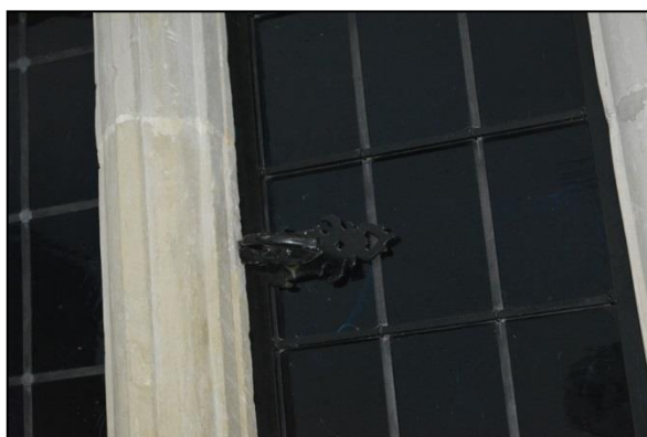
Plate 91: Room F7: window furniture detail (73)
