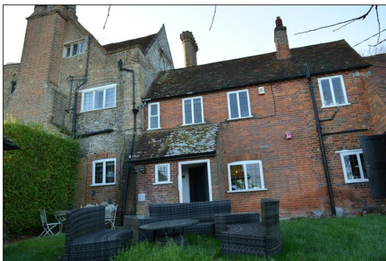
Plate 20: Building 2: north elevation (5)
