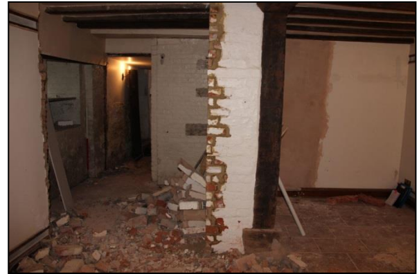
Plate 38: Room B3: view to south during works
