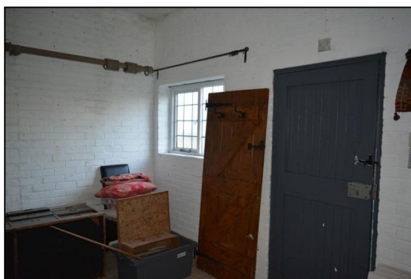
Plate 124: Outbuilding 2: view to northwest(105)
