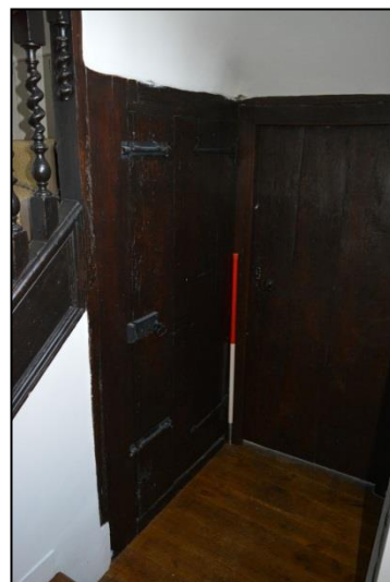
Plate 67: Room G5: southeast corner (49)
