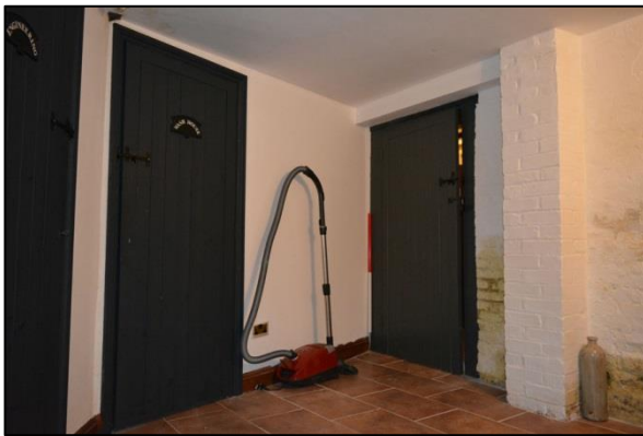
Plate 29: Room B1: northwest corner (14)
