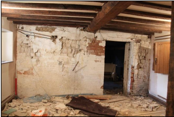
Plate 37: Room B3: north wall fabric exposed
