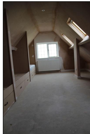
Plate 100: Room F12: view to west after restoration
