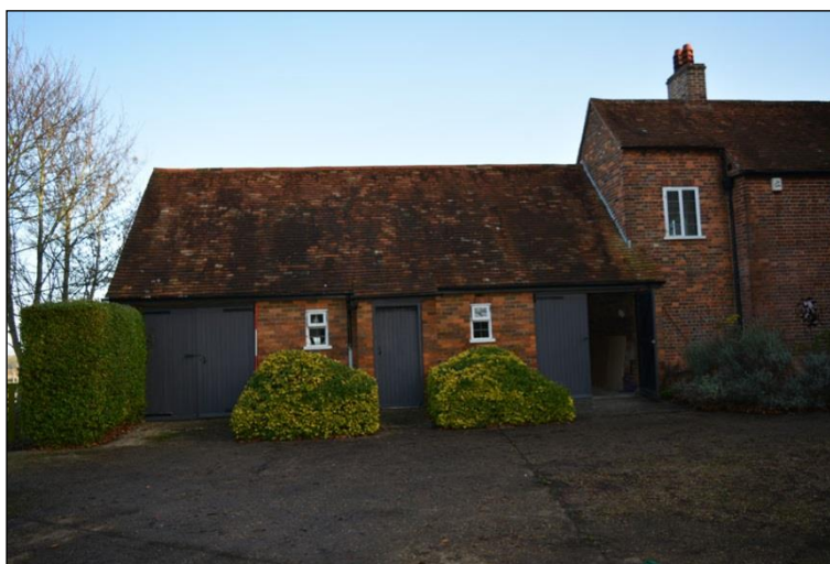
Plate 23: Building 3: south elevation (8)
