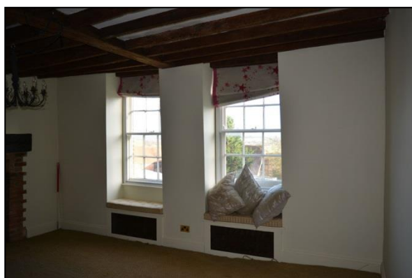
Plate 85: Room F6: east wall (67)
