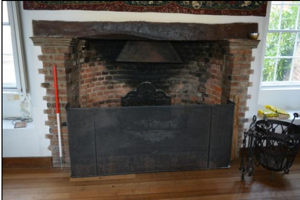
Plate 59: Room G3: fireplace detail (42)
