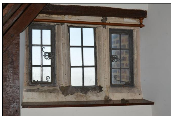
Plate 105: Room S1: north window detail (85)
