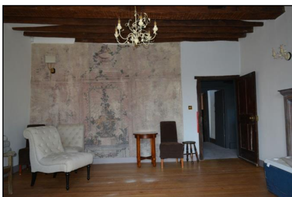
Plate 50: Room G2: view to west (33)
