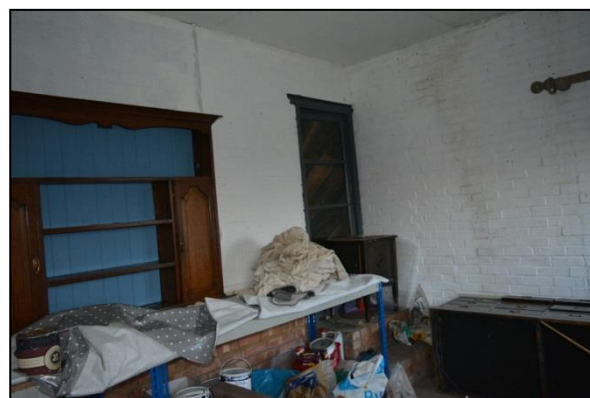
Plate 123: Outbuilding 2: view to southwest(104)
