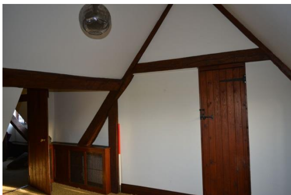
Plate 116: Room S5: west wall (95)
