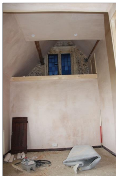
Plate 93: Room F8: view to east during renovation
