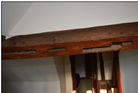
Plate 118: Room S5: redundant mortices in southern purlin (98)
