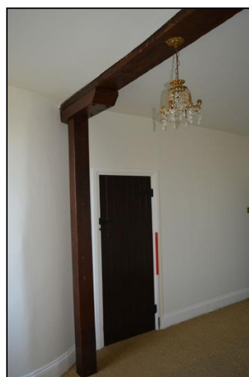
Plate 81: Room F4: timber detail (63)
