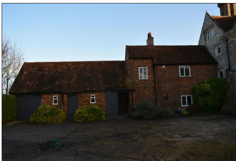
Plate 24: Buildings 2 & 3: south elevation (9)
