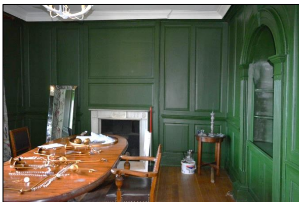
Plate 61: Room G4: south wall (43)
