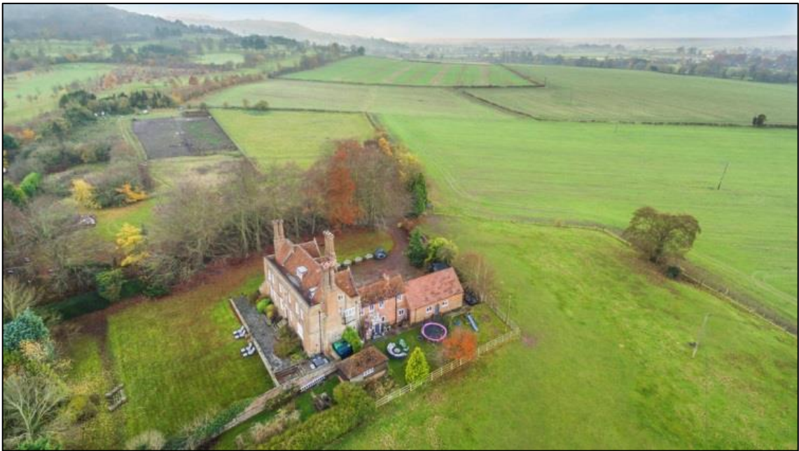
Plate 3: Aerial photo from the north(Courtesy of Fine & Country)
