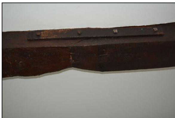
Plate 84: Room F5: timber detail (66)
