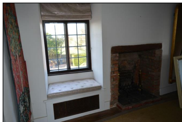
Plate 78: Room F3: window detail (60)
