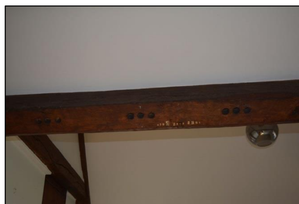
Plate 117: Room S5: stave holes in northern purlin (97)
