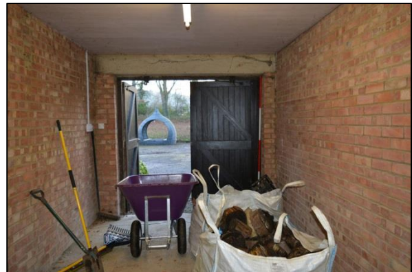
Plate 126: Outbuilding 3: view to south (107)
