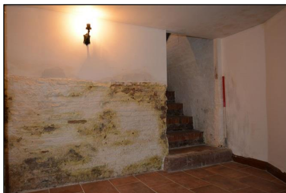
Plate 31: Room B1: east wall (16)
