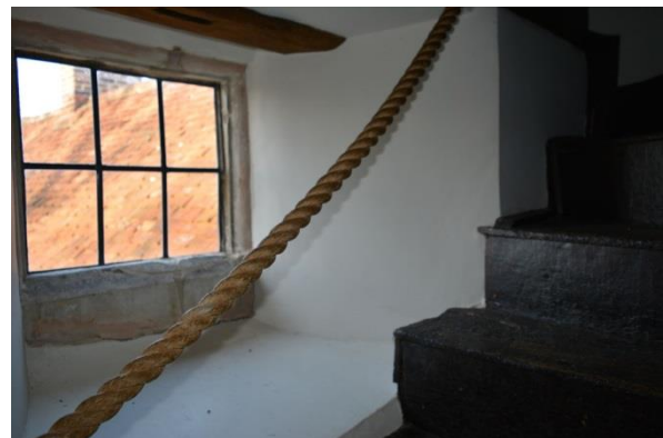
Plate 109: Room S2: stair detail (99)
