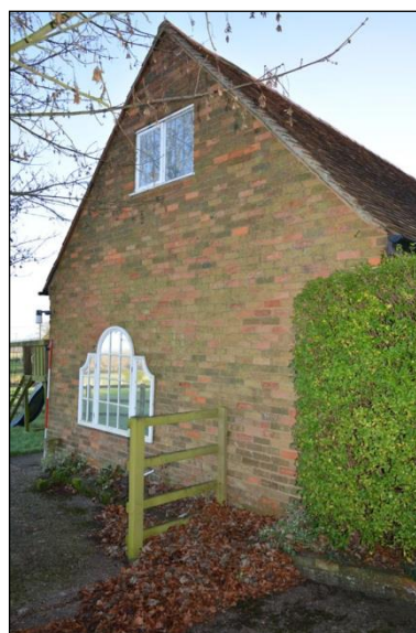
Plate 22: Building 3: west elevation (7)
