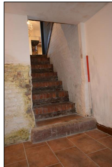
Plate 30: Room B1: southeast corner (15)
