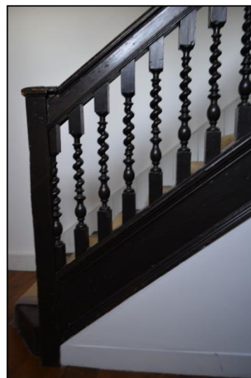
Plate 65: Room G5: stair detail (47)
