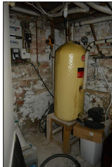
Plate 46: Room B7: southeast corner (29)
