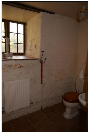
Plate 44: Room B6: view to northwest (27)
