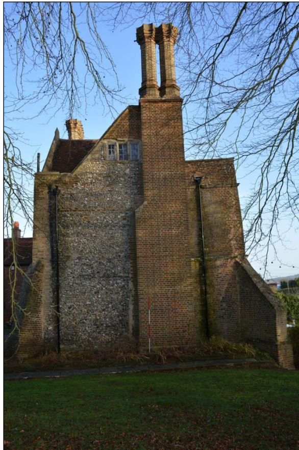
Plate 26: Building 1: south elevation (11)
