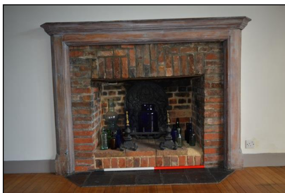
Plate 54: Room G2: fireplace detail (37)
