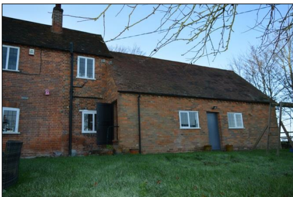
Plate 21: Building 3: north and east elevations (6)
