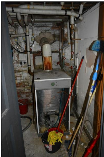
Plate 45: Room B7: view to south (28)
