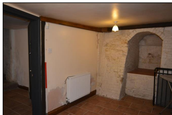
Plate 43: Room B5: view to southeast (26)
