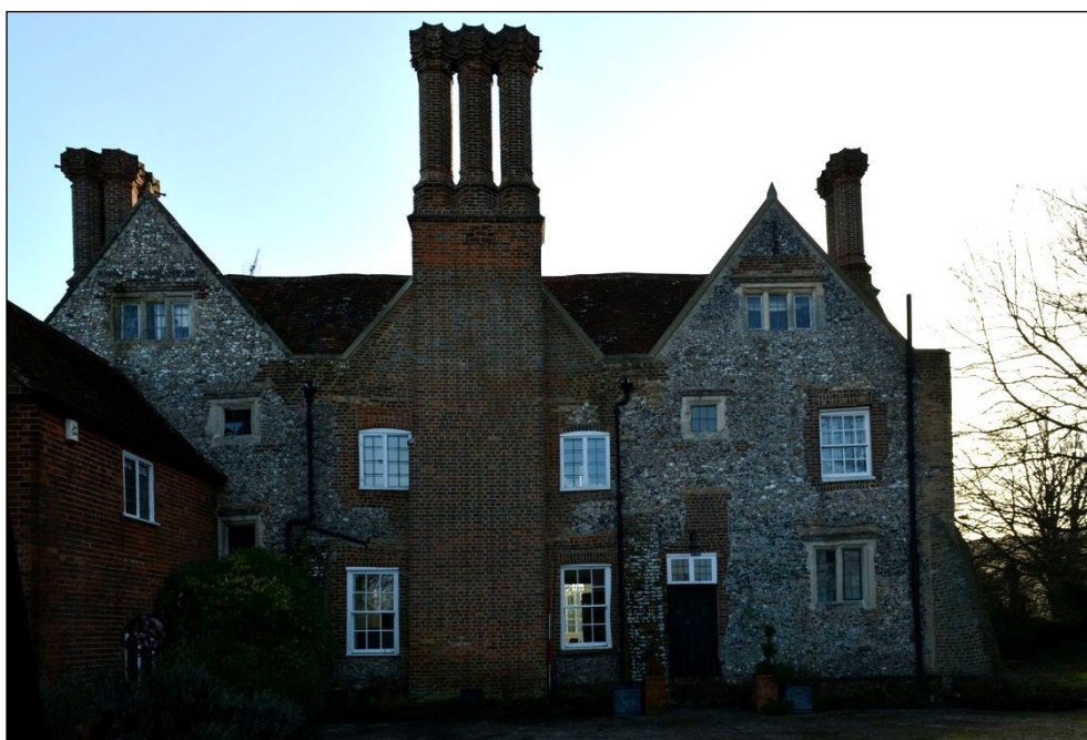
Plate 25: Building 1: west elevation (10)
