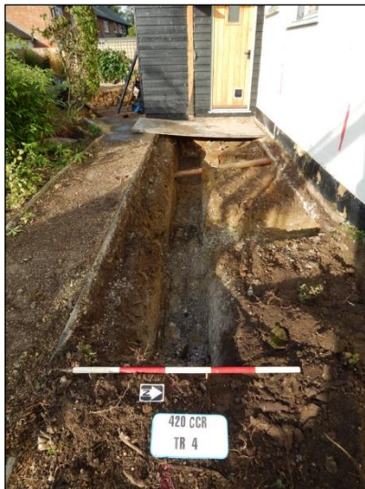
Plate 7: Trench 4, looking west
