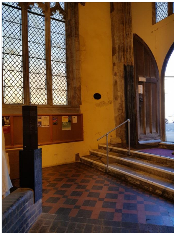
Plate 3: Northeast corner of the porch (courtesy of R. Turner)
