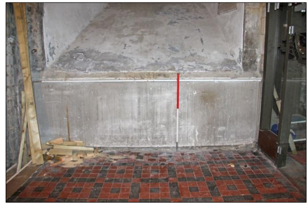
Plate 12: North aisle floor beneath northwest tower, view west
