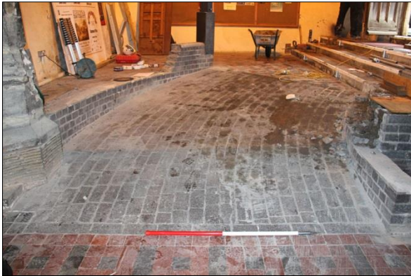
Plate 5: North porch floor, view north
