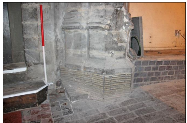
Plate 10: Southwest column and floor in North porch, view west-northwest
