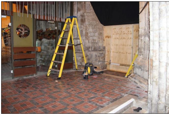
Plate 11: North aisle floor beneath northwest tower, view north-northeast
