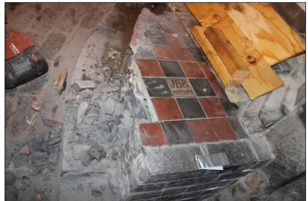
Plate 8: Removed section of floor in North porch, view northeast
