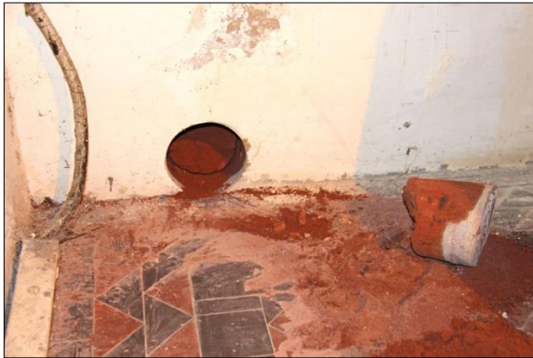
Plate 32: Hole for drainage in north wall of porch, view north
