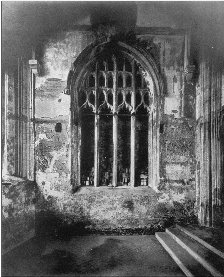
Figure 5: The north porch in 1899, with the north window still blocked by the Shambles (Beloe 1899, plate 9)
