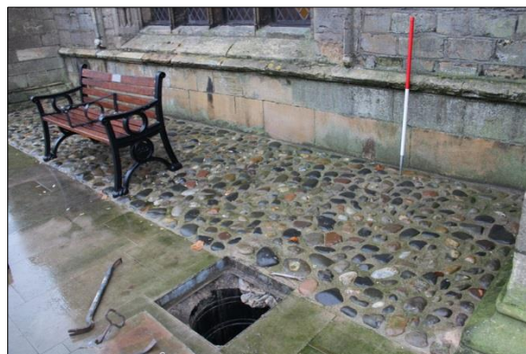
Plate 27: Pavement and cobbles to the north of the porch, before excavation
