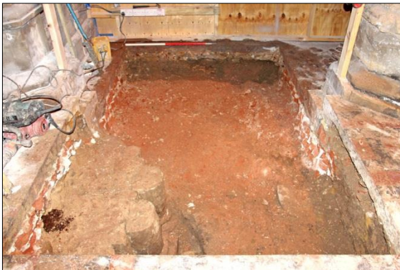
Plate 22: Excavation for wheelchair lift, view east
