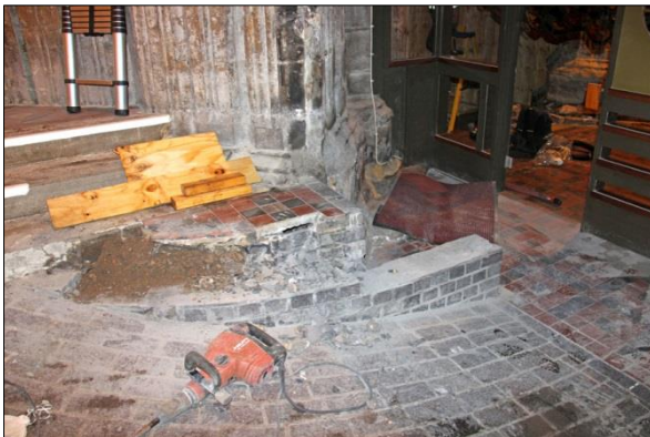
Plate 7: North porch steps, view southeast
