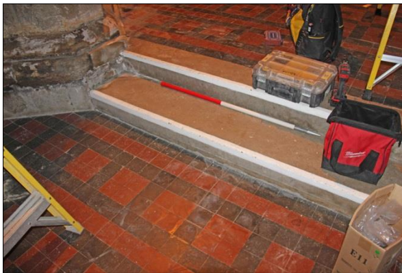
Plate 13: North aisle steps before removal for lift, view west-southwest
