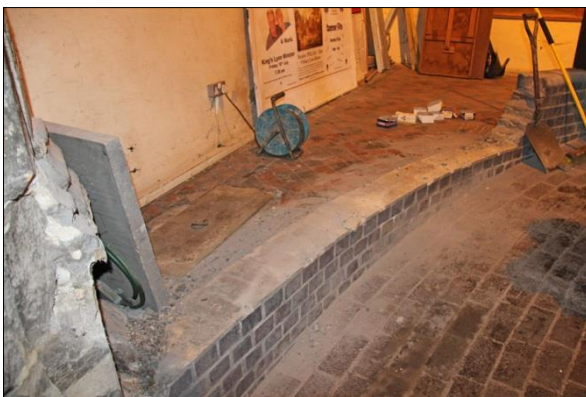
Plate 9: Removed wall in North porch, view north-northwest
