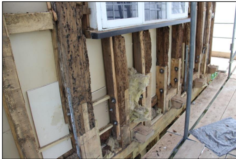
Plate 14: Modern repairs in the west elevation
