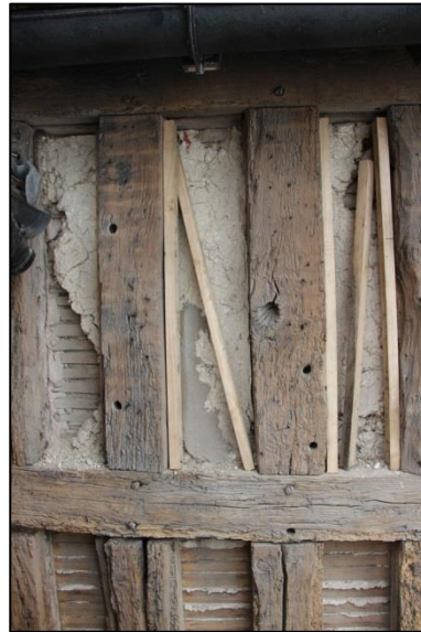
Plate 48: Stage 1: heightening studs ii
