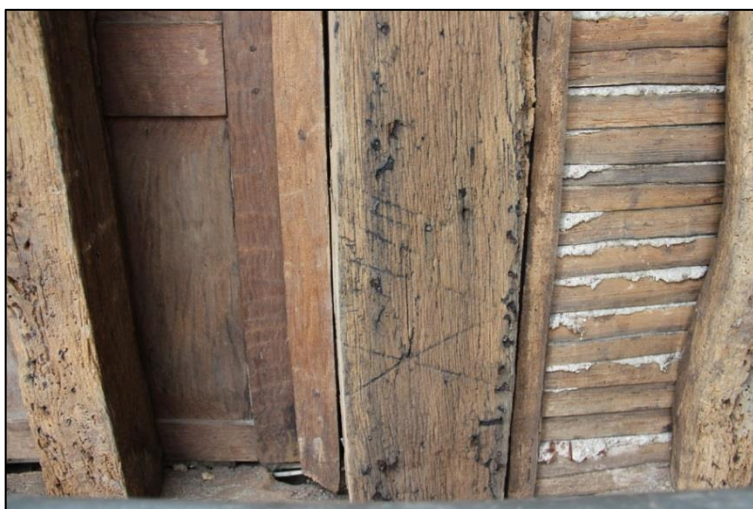
Plate 5: Carpenter's mark on a first floor post
