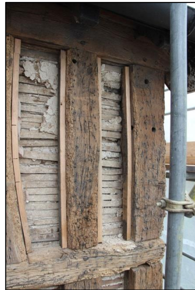
Plate 52: Stage 1: heightening studs ii
