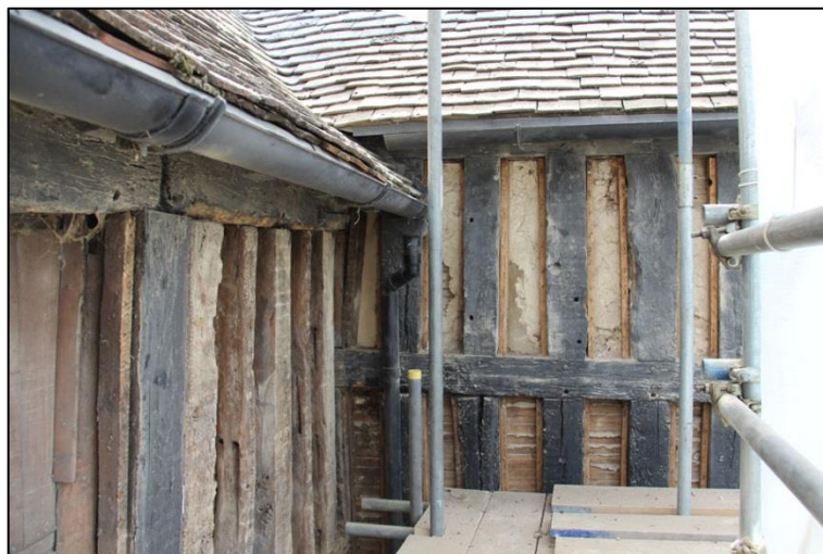
Plate 6: Cross wing north elevation
