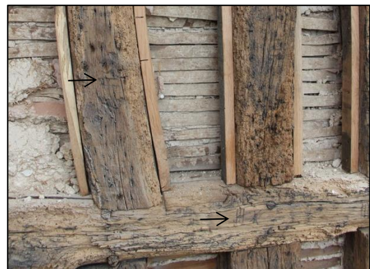
Plate 19-20: Carpenter's marks on the north elevation
