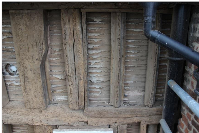
Plate 12: Eastern window in the south elevation
