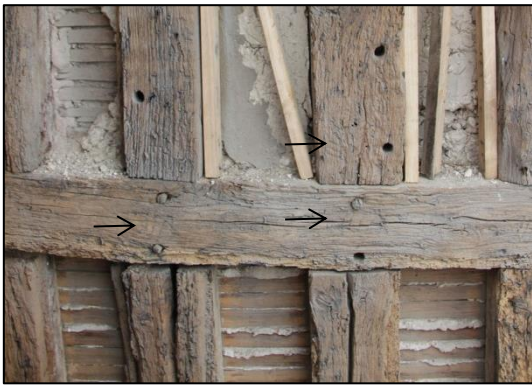
Plate 17-18: Carpenter's marks on the north elevation
