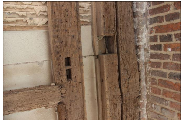
Plate 88: First floor: mortice details
