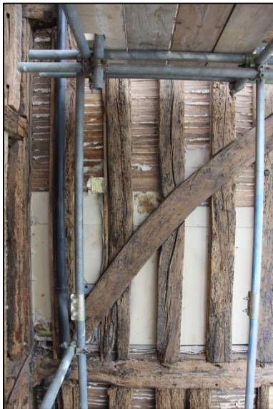
Plate 53: First floor: brace
