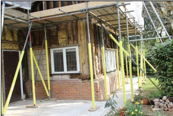
Plate 45: Ground floor with modern brick plinth
