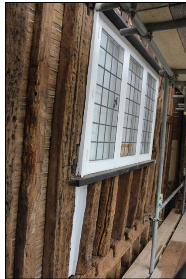
Plate 41: First floor window
