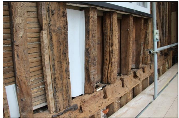
Plate 31: Midrail with redundant seatings for window
