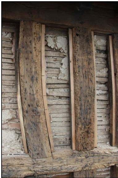
Plate 51: Stage 1: heightening studs v
