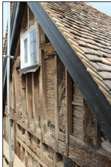
Plate 59: Upper window from the south
