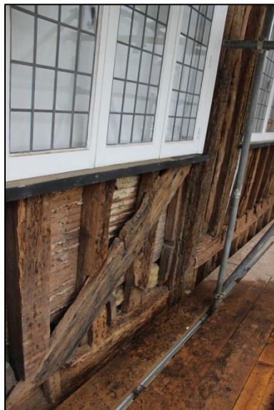
Plate 38: Brace beneath first floor window
