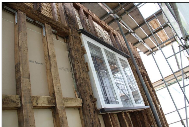
Plate 13: Fenestration at first floor level in the west wall of the cross wing
