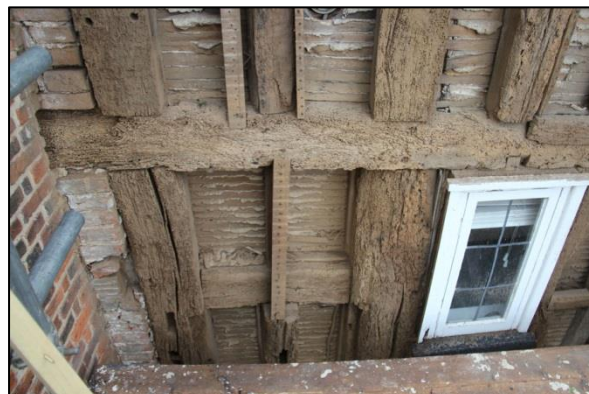
Plate 93: Top stage: western end detail
