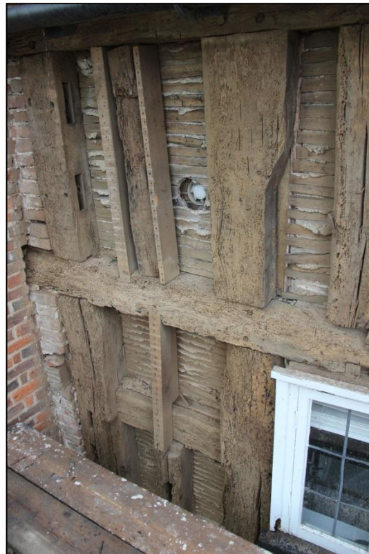
Plates 8 & 9: South elevation; cut and re-instated jowlposts to the west and east of chimney stack
