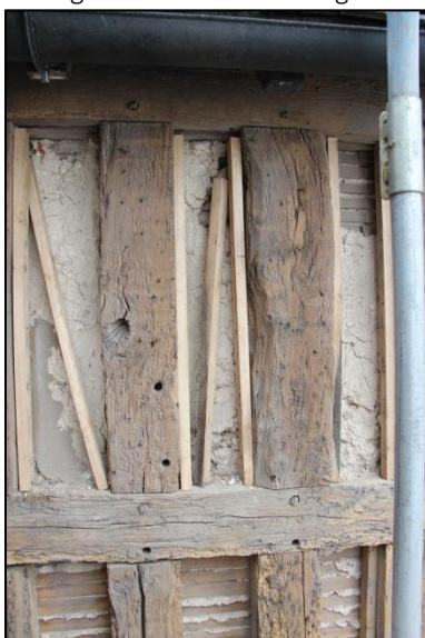
Plate 49: Stage 1: heightening studs iii
