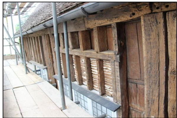
Plate 25: Top stage from the south
