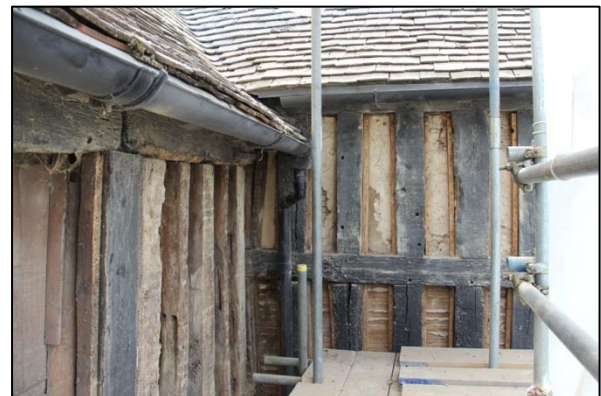
Plate 56: Upper level of timberwork before cleaning
