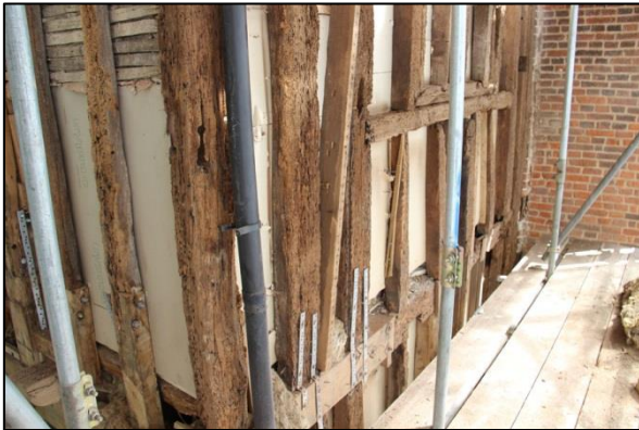
Plate 87: First floor timbers from the west
