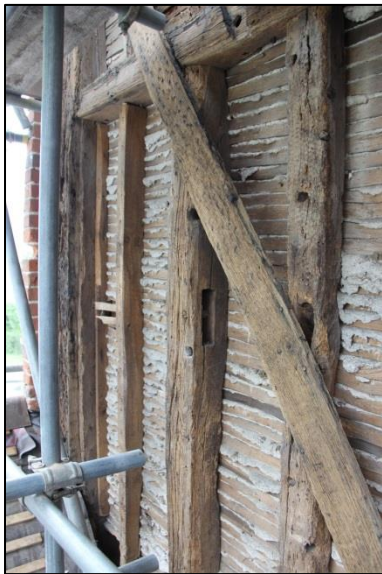
Plate 40: Brace at the northern end
