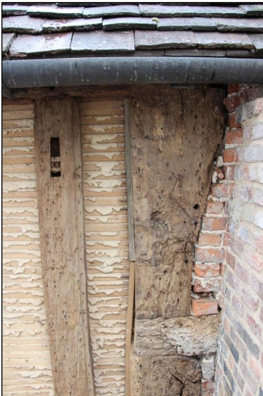
Plates 8 & 9: South elevation; cut and re-instated jowlposts to the west and east of chimney stack
