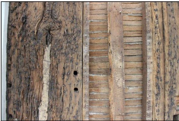
Plate 30: Detail photo of post and laths
