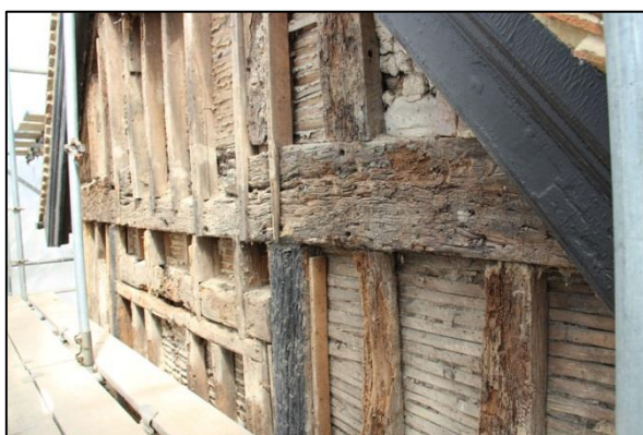
Plate 60: Top stage: timberwork from the south
