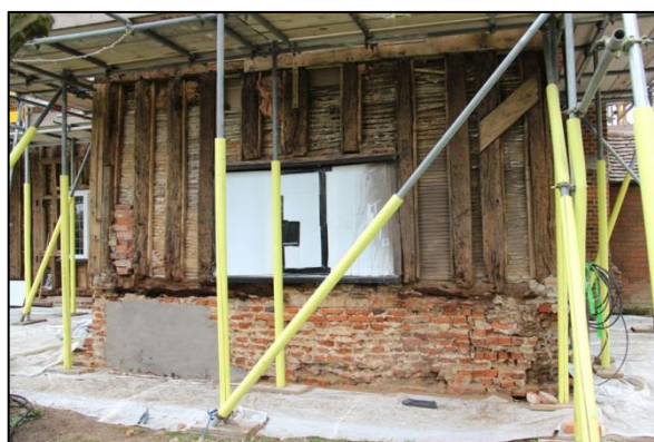
Plate 74: Ground floor with the original dwarf wall
