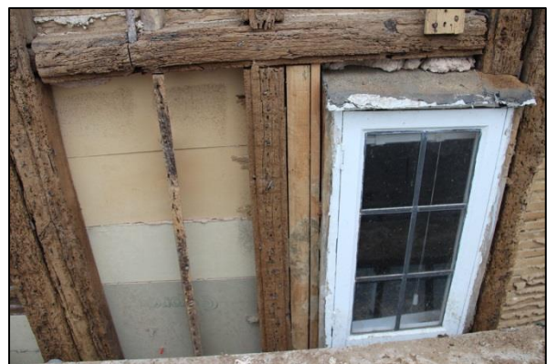
Plate 78: Top stage : later window set within frame of mullioned window
