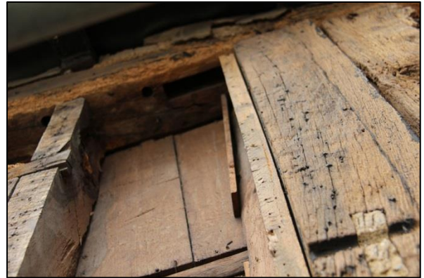
Plate 35: First Floor: internal panelling & Hertfordshire grooves in the soffit
