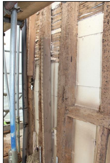
Plate 82: First floor level from the east
