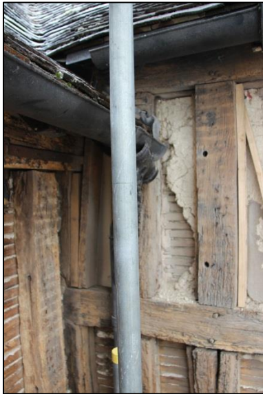
Plate 47: Stage 1: later studs to heighten the wing
