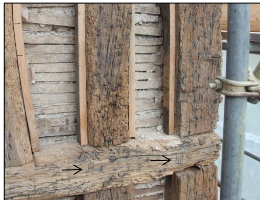
Plate 21: Carpenter's marks on the north elevation
