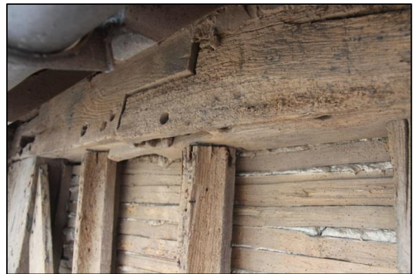
Plate 37: Bridle butted scarf joint in the wallplate
