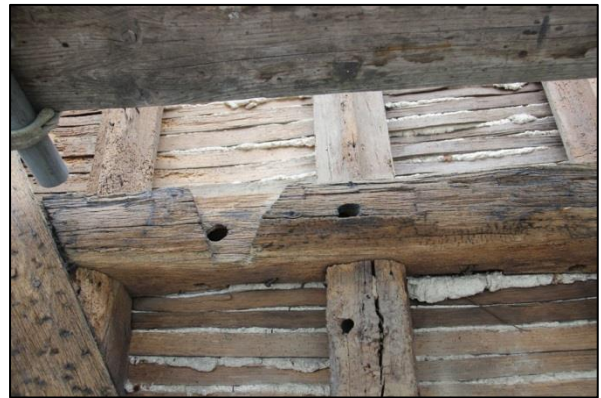
Plate 29: Redundant mortice and peg holes
