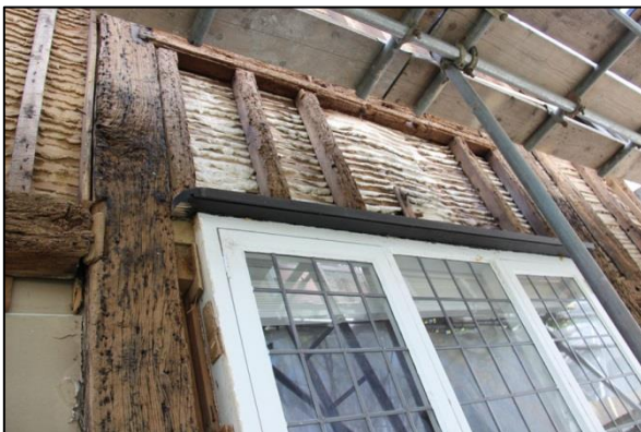
Plate 68: Frame above the first floor window
