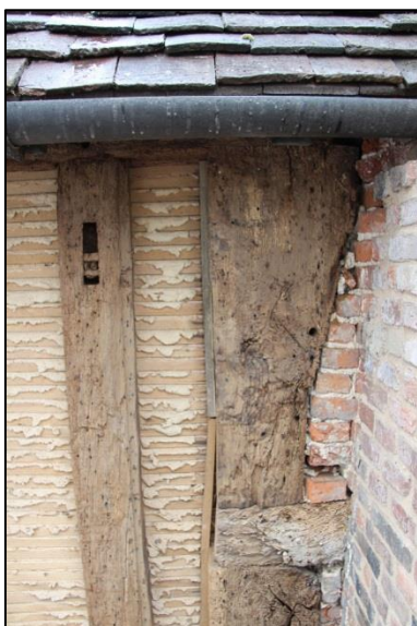
Plate 79: Top stage: truncated and reinstated jowlpost
