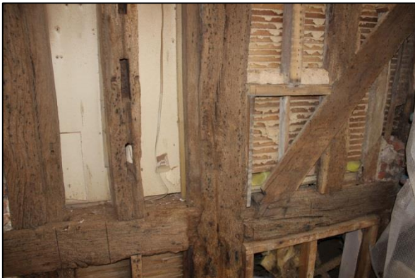
Plate 104: First floor timber detail
