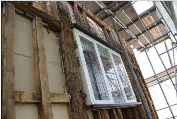
Plate 64: First floor window from the north
