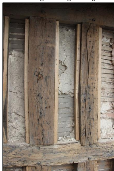
Plate 50: Stage 1: heightening studs iv
