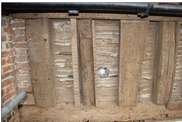
Plate 92: Top stage: western end detail
