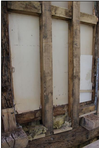
Plate 66: Timbers north of the first floor window
