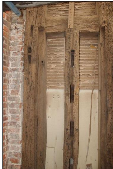
Plate 105: First floor timber detail
