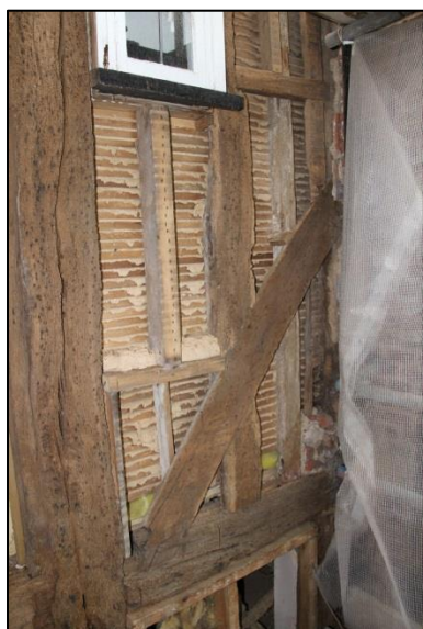
Plate 100: First floor: eastern end
