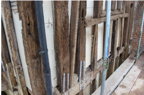
Plate 81: First floor level from the west
