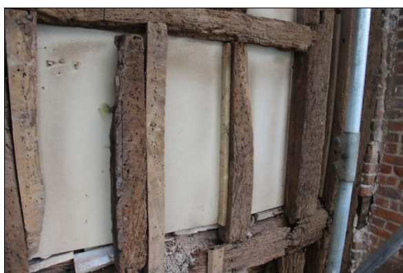
Plate 85: Timbers below mullioned window
