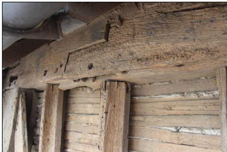
Plate 2: Bridle butted scarf joint and Hertfordshire staves
