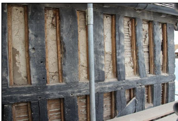
Plate 57: Upper level of timberwork before cleaning
