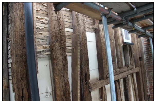
Plate 80: First floor level from the west
