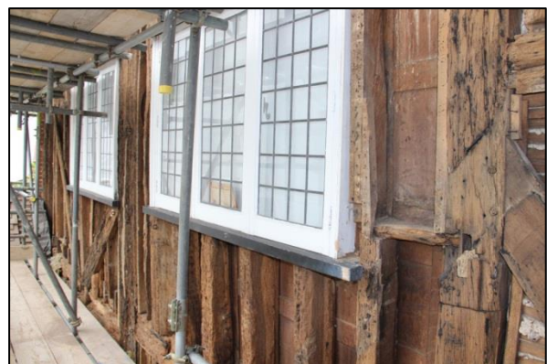
Plate 27: First Floor level from the south
