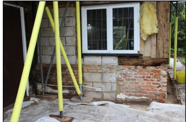
Plate 46: Ground floor with original brick dwarf wall
