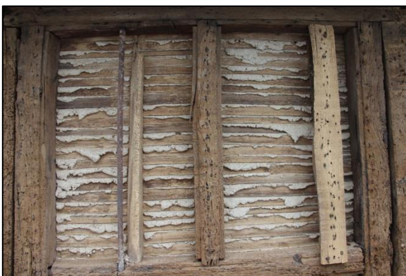
Plate 77: Top stage : mullioned window
