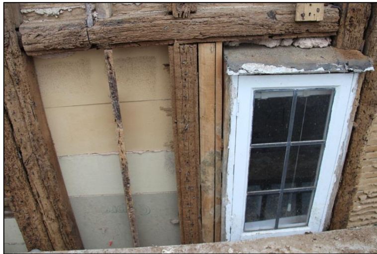
Plate 11: Lower section of mullioned window incorporating later casement
