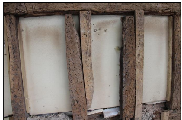
Plate 84: Timbers below mullioned window
