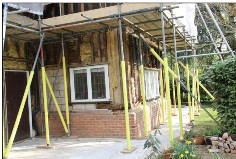
Plate 16: Breeze block in the north elevation of the cross wing
