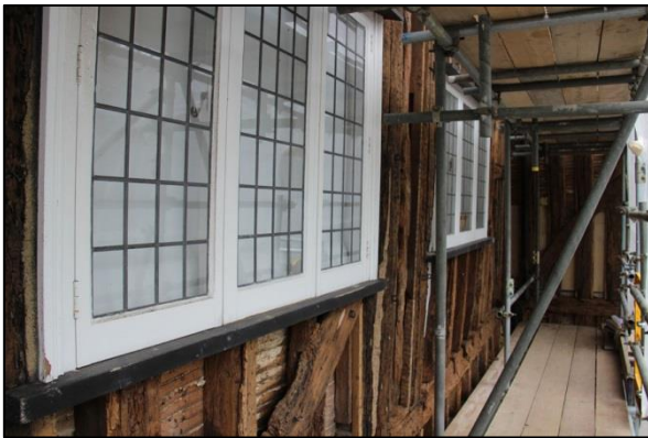
Plate 28: First floor level looking south
