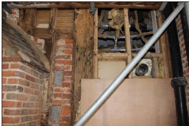
Plate 15: Modern studwork in the south elevation
