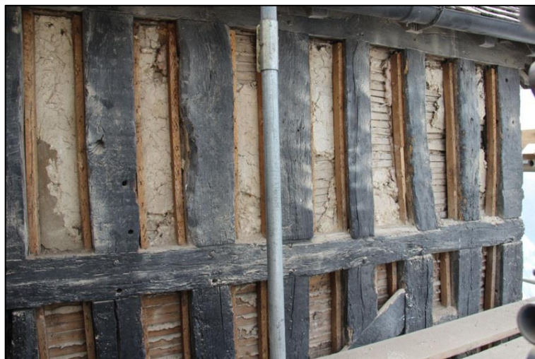
Plate 7: Cross wing north elevation
