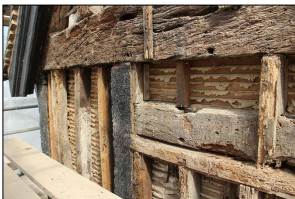
Plate 62: Top stage: detail of timberwork from the south
