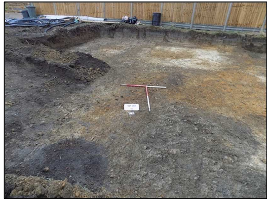
Plate 2: Trench 1, looking east (scale 2x1m)
