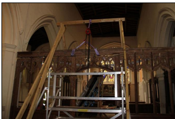
Plate 56: Chancel screen being removed
