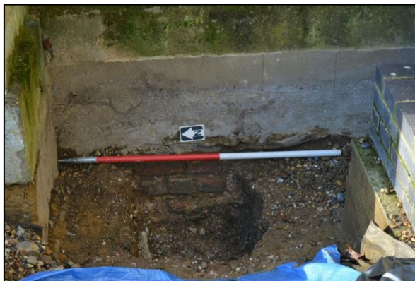
Plate 1: External test pit (NB arrow is pointed south)
