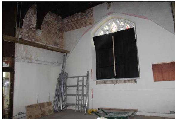
Plate 51: South and east walls of the south transept
