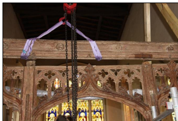
Plate 57: Chancel screen beam being lifted
