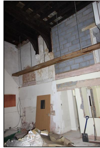
Plate 50: West wall of the south transept
