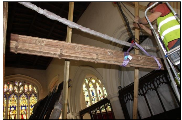
Plate 61: Underside of upper beam of chancel screen
