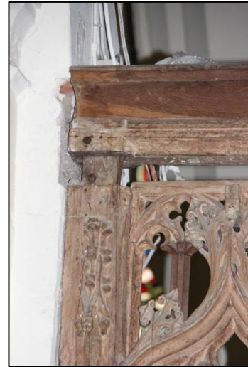
Plate 59: Chancel screen, mortice & tenon detail
