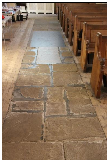
Plate 102: South aisle floor: view to west (35)
