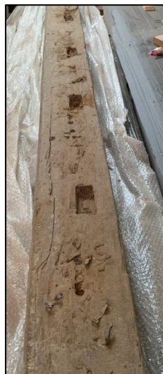
Plate 62: Mortices on the top of the chancel screen beam (Photo courtesy of Tom Frost)
