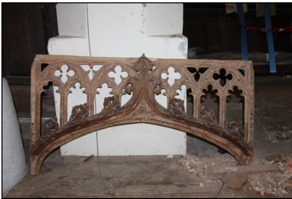
Plate 60: Central tracery detail showing later repair
