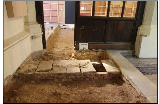
Plate 46: Structural details revealed in ground reduction in the Lady Chapel
