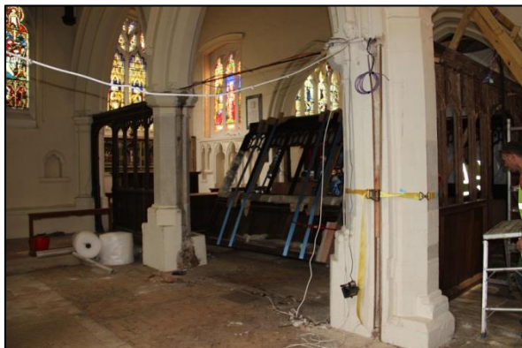
Plate 64: Screen having been removed
