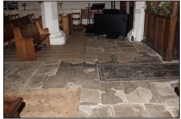
Plate 99: Nave floor, east end: view to north (32)
