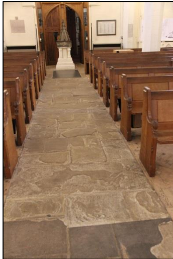
Plate 100: Nave floor: view to west (33)
