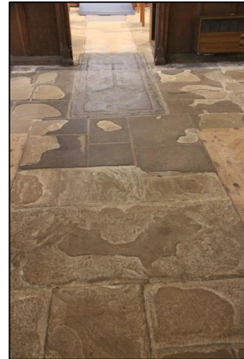
Plate 101: Nave floor: view to east (34)
