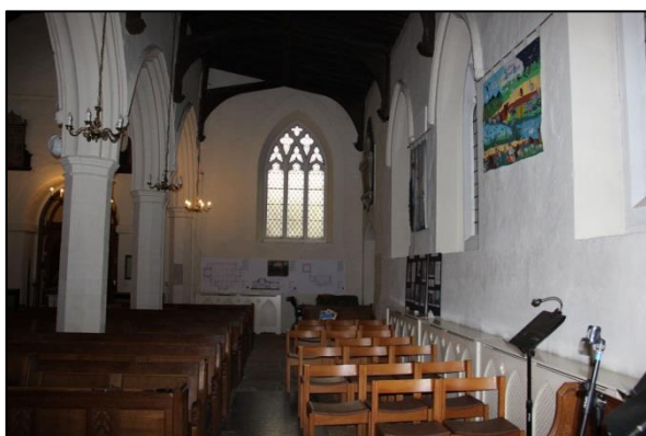
Plate 84: North aisle: view to west (17)
