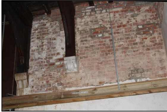
Plate 49: Corbels on the east wall of the south transept
