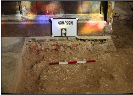
Plate 45: Footings below the Lady Chapel screen from the south
