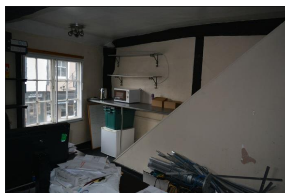
Plate 19: Room F3: view to northeast (9)
