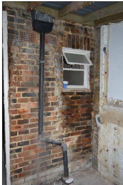
Plate 10: Room G4: northeast corner (18)
