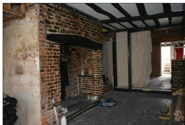
Plate 6: Room G2: fireplace (14)
