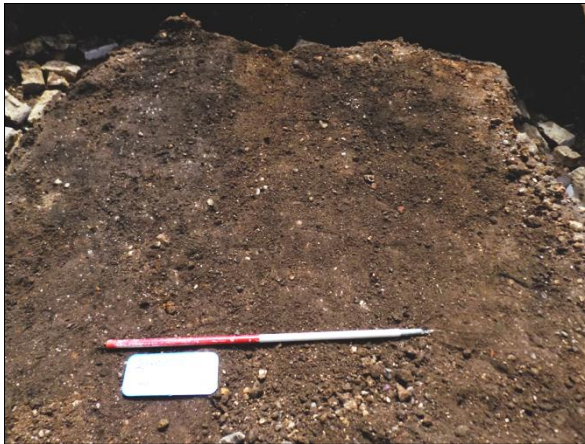
Plate 1: Graded area for proposed patio, facing southwest
