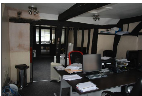
Plate 18: Room F3: view to south (8)
