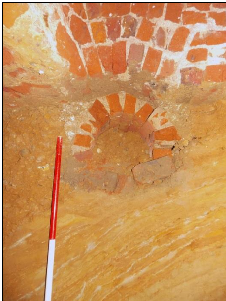
Plate 9: Section of brick drain and footing
