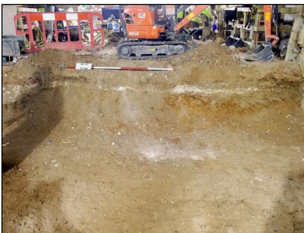
Plate 11: Section of Surface [024], facing southeast
