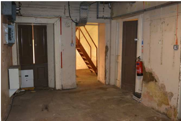
Plate 43: B4: south wall with the dumb waiter to the left (21)
