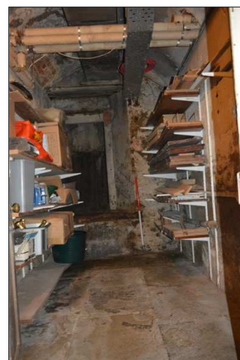
Plate 34: B5: former pantry, view to west (27)
