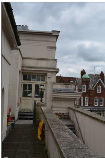
Plate 7: Western walkway looking north (80)
