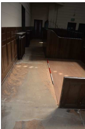
Plate 102: G13: view to east after the floor was stripped (24)
