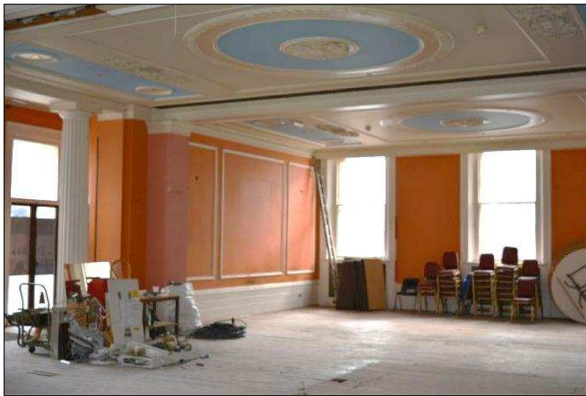
Plate 59: G2a & b: northeast corner (5)
