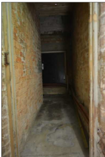
Plate 12: Cellar: side room, looking west (3)
