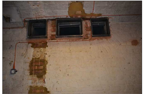
Plate 42: B8 & 9: north wall (20)
