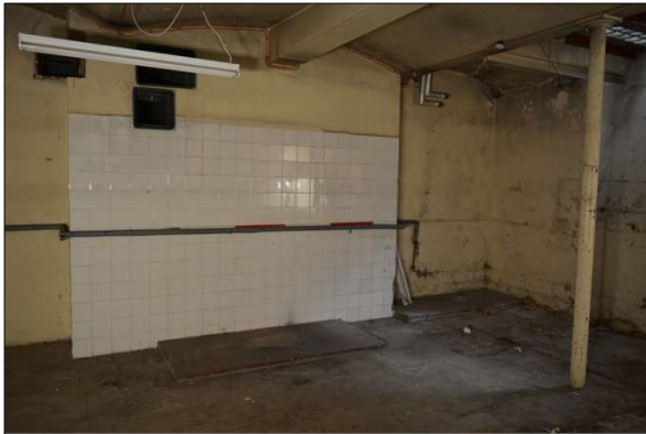
Plate 41: B10: north wall (18) (38)
