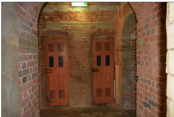
Plate 14: Cell doors with relieving arch above (5)
