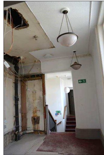
Plate 129: F7-8: facing south once stripped (14)
