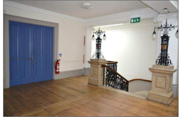
Plate 118: F2: view towards the stairs (70)
