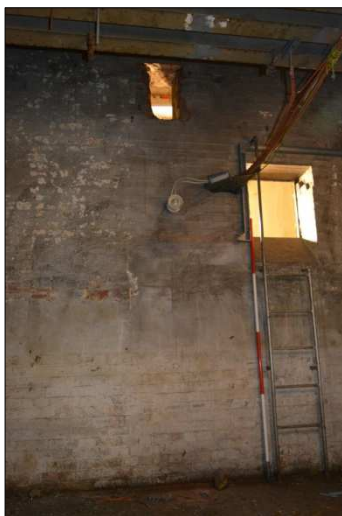
Plate 45: B3: north wall (23)
