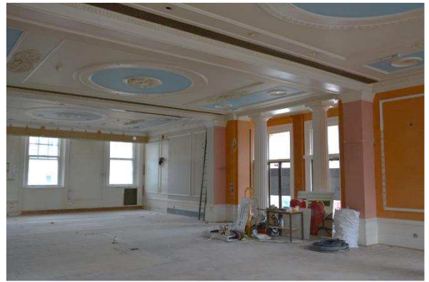
Plate 56: G2a & b: northwest corner (2)
