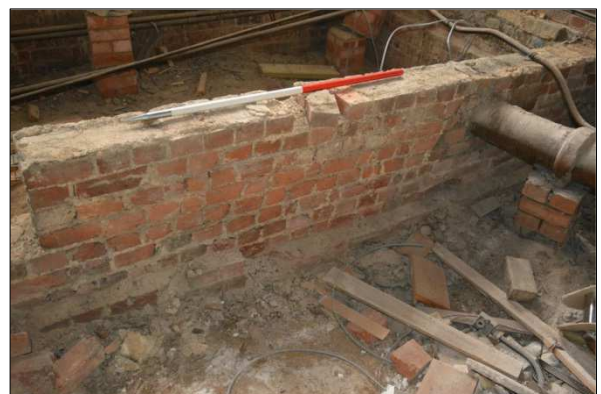
Plate 74: G2: supporting wall detail (42)
