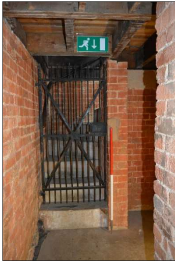
Plate 10: Cellar: stairs leading to the courtroom (1) (8,9)
