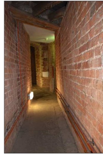
Plate 11: Cellar: passage to the court view to south (2)
