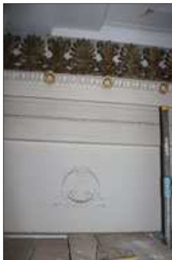
Plate 123: F3: cornice and moulding detail (58)
