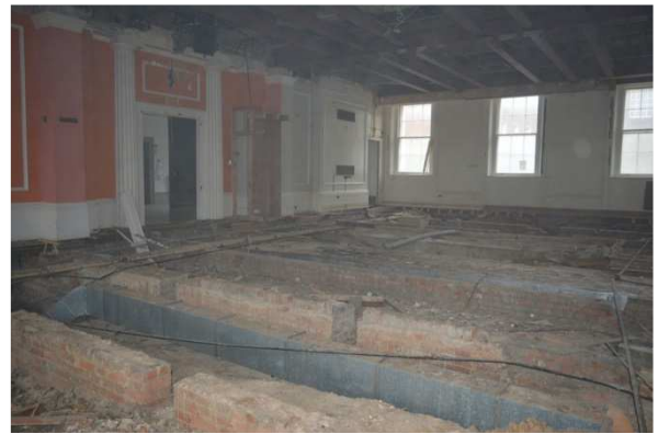
Plate 68: G2a & b: view to southwest (35)
