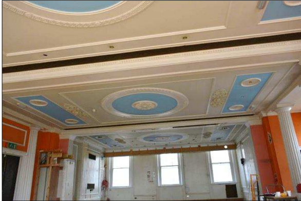
Plate 63: G2a & b: ceiling detail (9)
