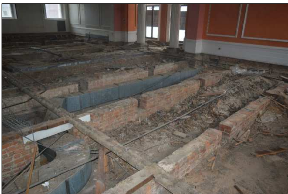
Plate 67: G3: supporting wall detail (34)
