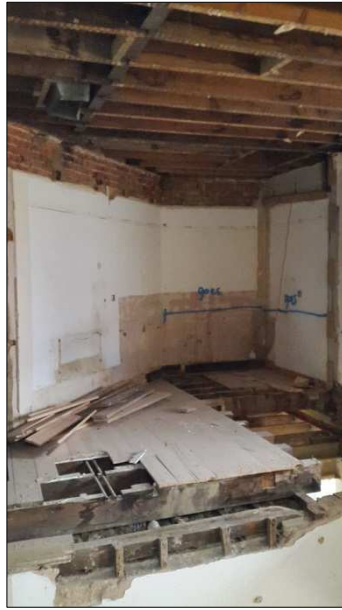
Plate 132: F10: view to south once stripped (30)
