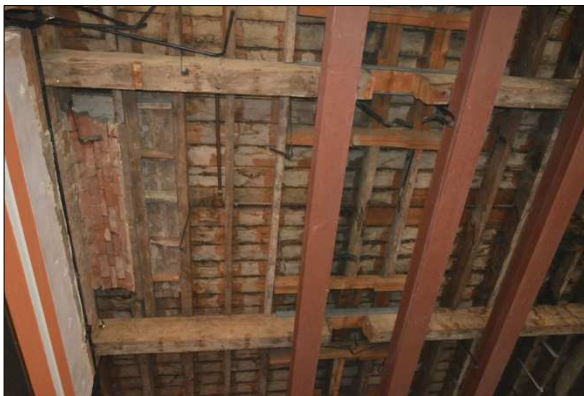
Plate 71: G2a & b: ceiling detail (38)
