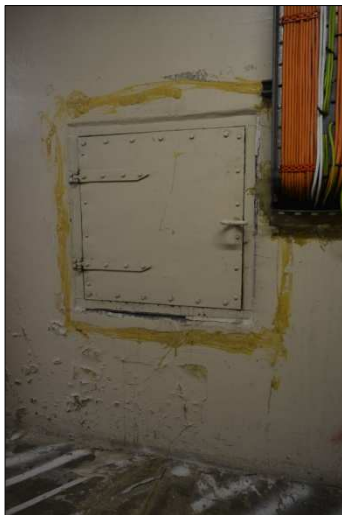
Plate 37: B7: hatch in south wall (30)
