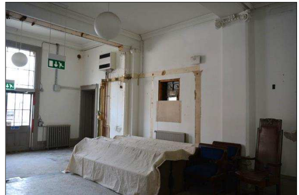
Plate 85: G3: northwest corner after the office was removed (10)
