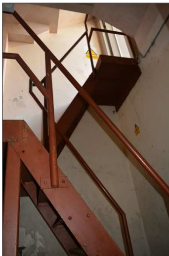
Plate 27: B1: staircase to service cellar (20)
