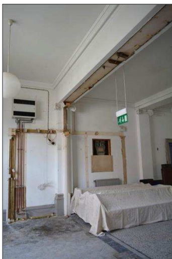
Plate 86: G3: detail of former partition wall (11)
