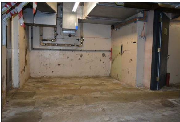
Plate 31: B4: north wall (24)
