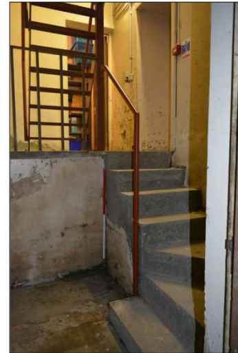
Plate 30: B1: steps into main service area (23)
