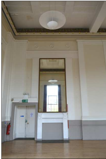
Plate 121: F3: fireplace in south wall (76)
