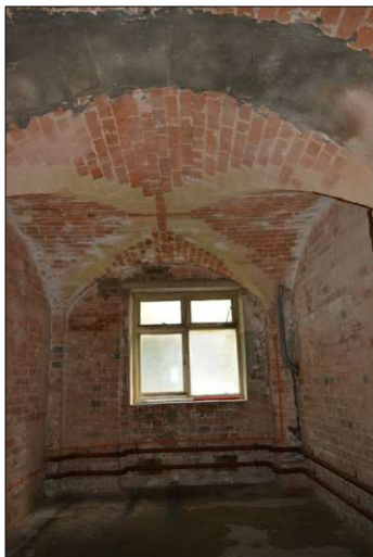
Plate 18: Cellar: former men's cell looking south (9)
