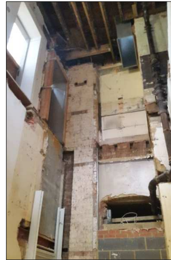
Plate 89: Lift shaft stripped
