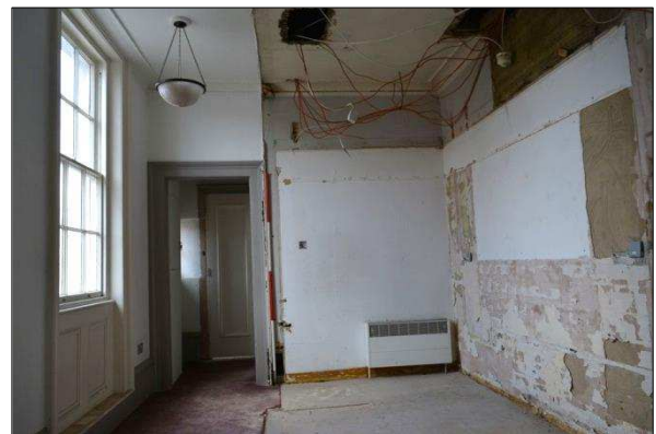
Plate 131: F8: facing north once stripped (16)
