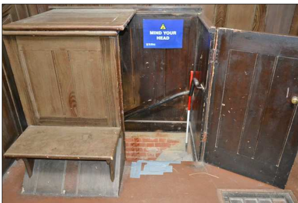
Plate 90: G13: stair from the cells (18)
