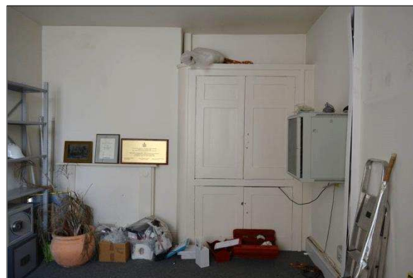
Plate 136: F21: south wall (86)
