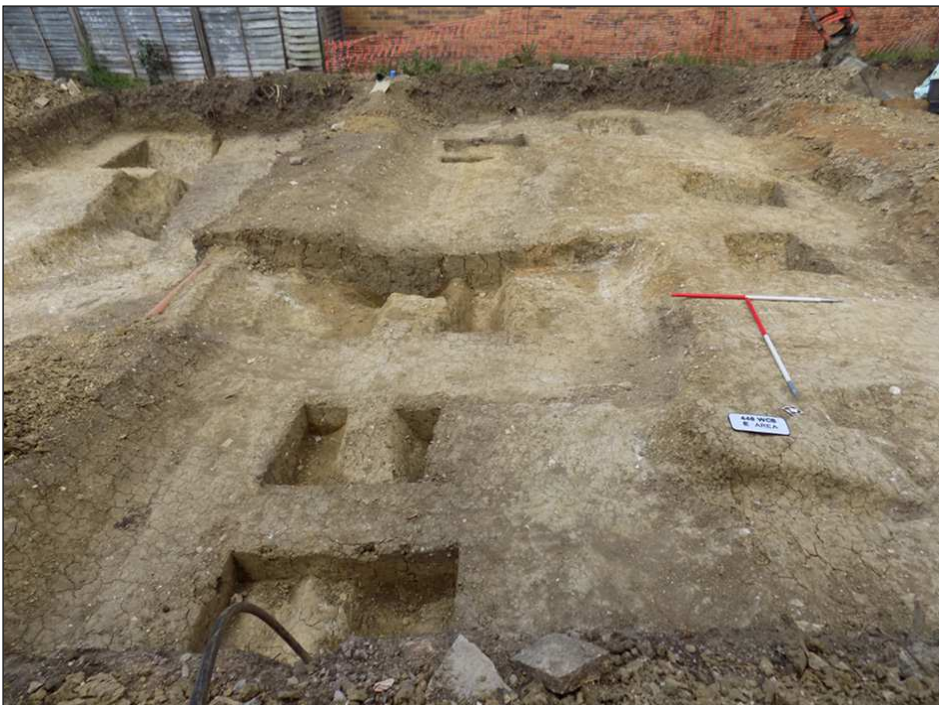
Plate 8: Excavation area overview, looking northeast
