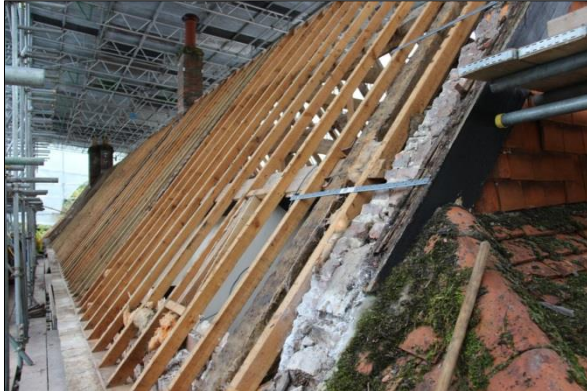
Plate 73: North roof, oblique (49)
