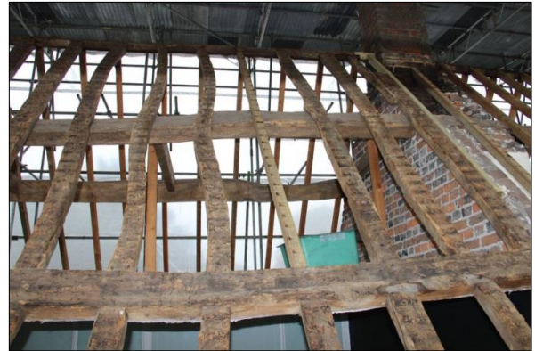
Plate 44: South roof, Bay 2 (94)
