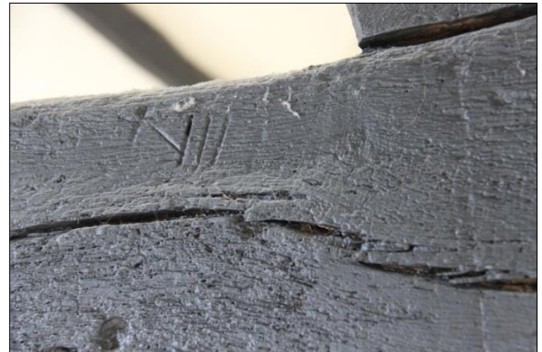
Plate 22: Truss 3 carpenter's marks, facing west (22)
