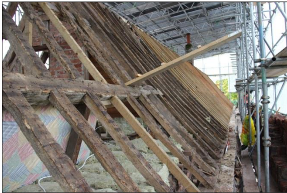
Plate 93: North roof, Bay 7 (78)
