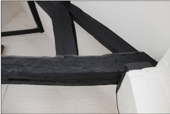
Plate 25: Truss 4 carpenter's marks, facing west (25)
