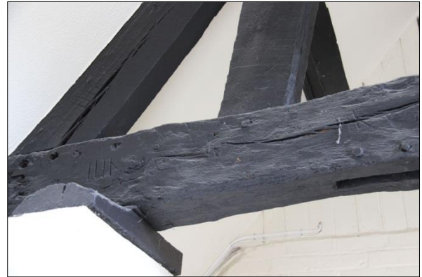
Plate 26: Truss 4 carpenter's marks, facing west (26)
