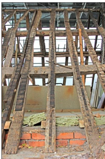
Plate 59: South roof, Bay 6 (113)
