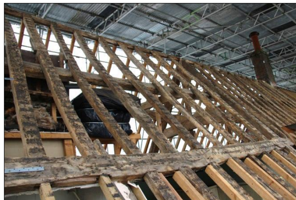
Plate 38: South roof, Bay 1 (86)
