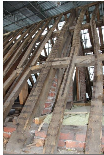
Plate 56: South roof, Truss 5 (110)
