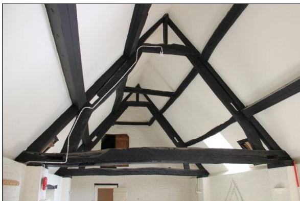
Plate 11: Truss 3, facing east (10)
