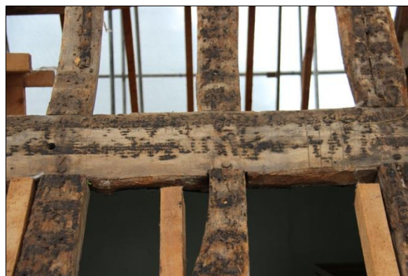
Plate 40: South roof, Bay 1 (91)
