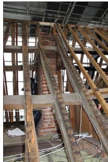
Plate 82: North roof, Bay 5 (62)
