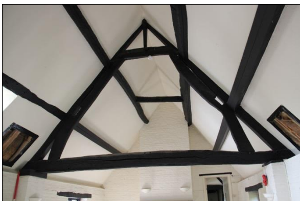
Plate 17: Truss 3, facing west (6)
