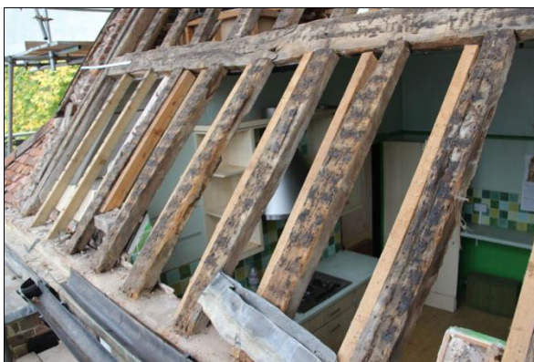
Plate 35: South roof, Bay 1 (90)
