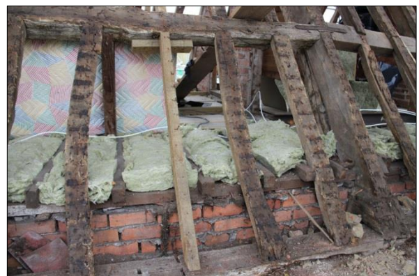
Plate 90: North roof, Bay 6 (71)
