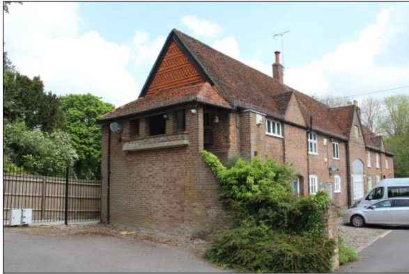
Plate 2: West and south elevations (40)
