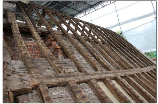
Plate 68: South roof, Bay 7 (118)
