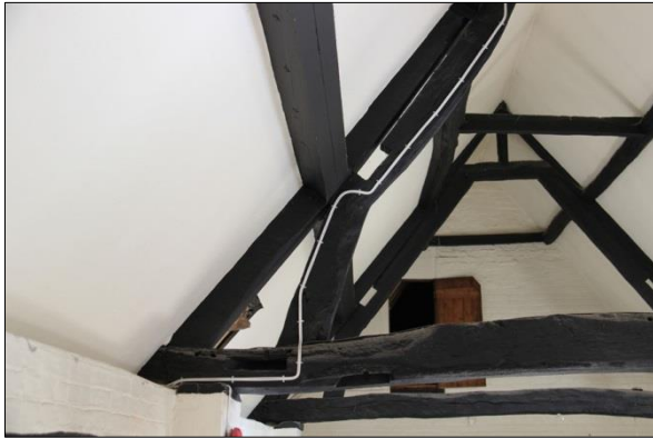
Plate 13: Truss 3, facing east (13)
