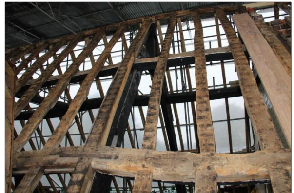
Plate 52: South roof, Truss 4 (104)
