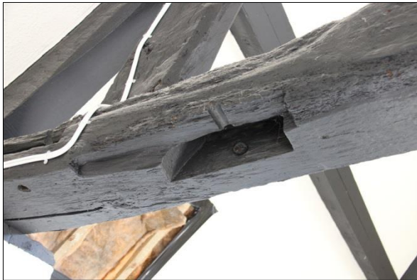
Plate 15: Truss 3 soffit mortice, facing east (15)
