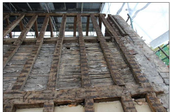
Plate 72: South roof, Bay 7 (123)
