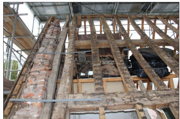
Plate 34: South roof, Bay 1 (87)
