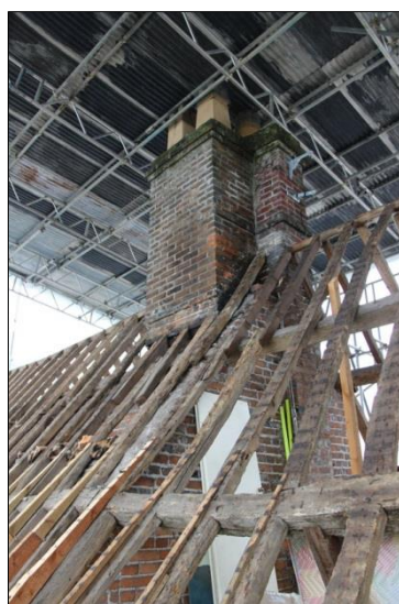
Plate 95: North roof, Bay 6 (75)
