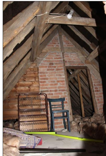
Plate 28: Truss 5 in the roof space above F5, facing east (41)
