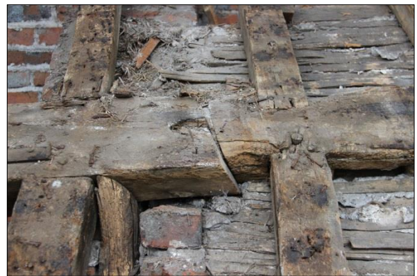
Plate 64: South roof, Bay 7 scarf joint (120)
