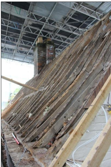
Plate 81: North roof, Bay 5 (61)
