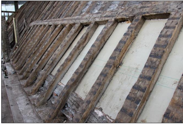
Plate 67: South roof, Bay 7 (124)
