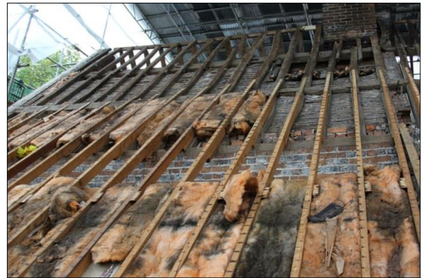
Plate 98: North roof, Bay 7 (80)
