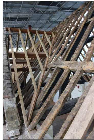
Plate 50: South roof, Bay 4 (103)
