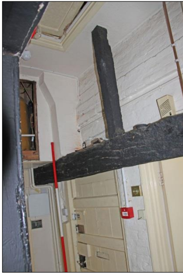
Plate 7: Truss 1, facing southwest (1)
