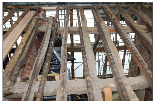
Plate 54: South roof, Bay 5 (107)
