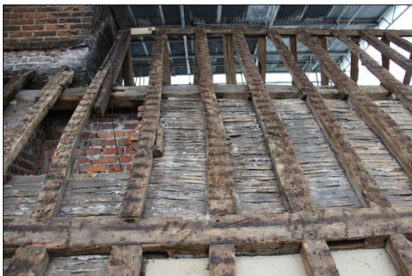
Plate 65: South roof, Bay 7 (121)
