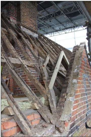
Plate 61: South roof, main chimney (115)
