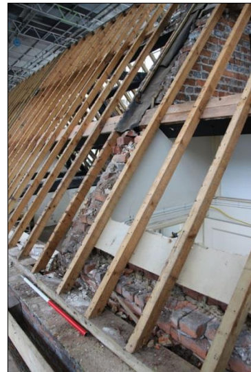
Plate 76: North roof, Bay 1 (52)
