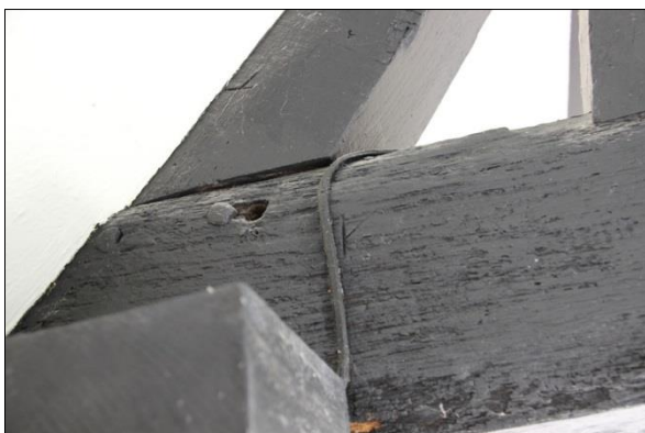
Plate 23: Truss 3 carpenter's marks, facing west (23)
