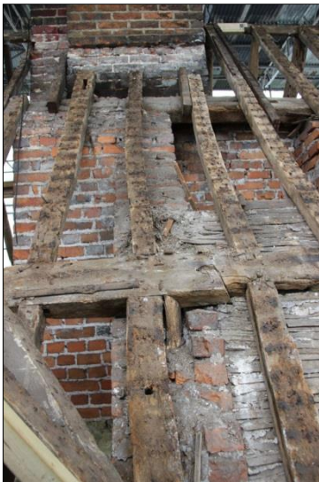
Plate 63: South roof, main chimney (117)
