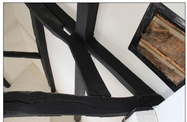
Plate 18: Truss 3, facing west (7)
