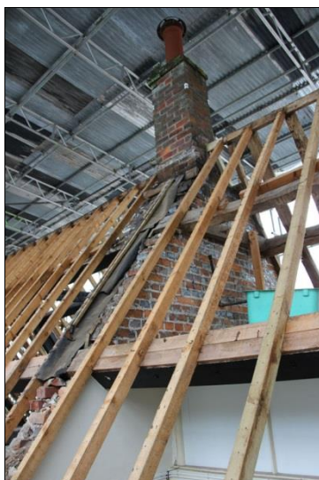
Plate 77: North roof, Bay 2 (53)
