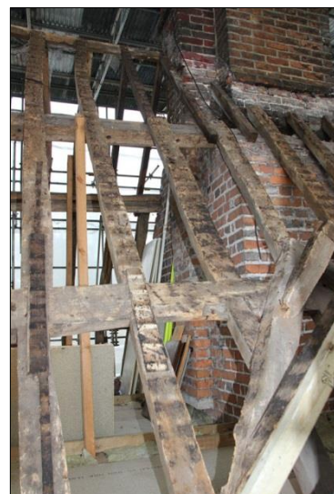
Plate 60: South roof, Bay 6 (114)
