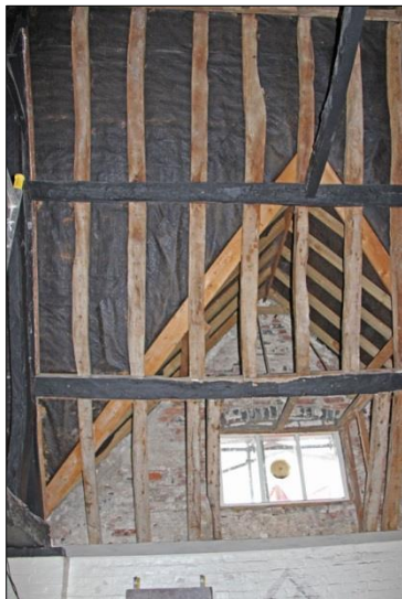
Plate 31: Rafters exposed in F4, facing south (47)
