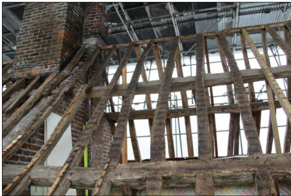
Plate 91: North roof, Bay 6 (72)
