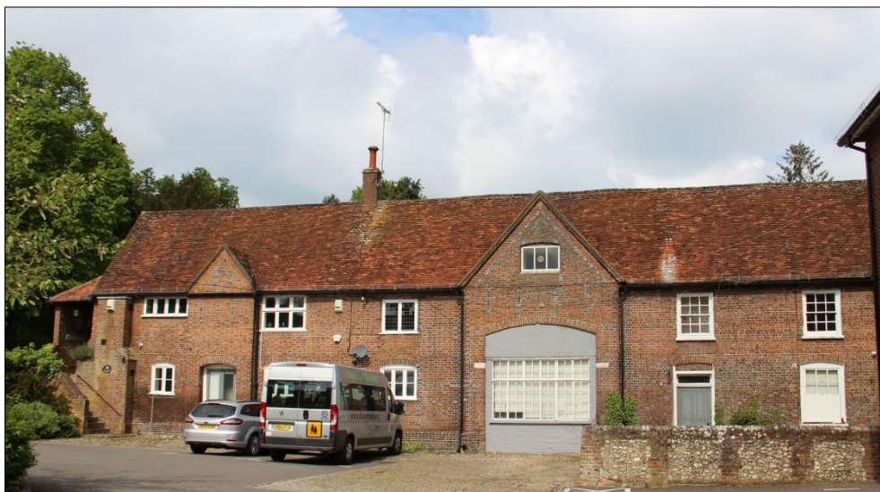
Plate 1: Main elevation with the date over the former carriageway (Shot 37)
