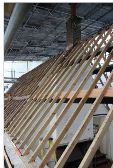
Plate 48: South roof, Bay 3 (101)
