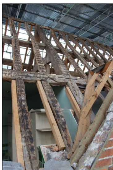
Plate 41: South roof, Truss 2 (92)
