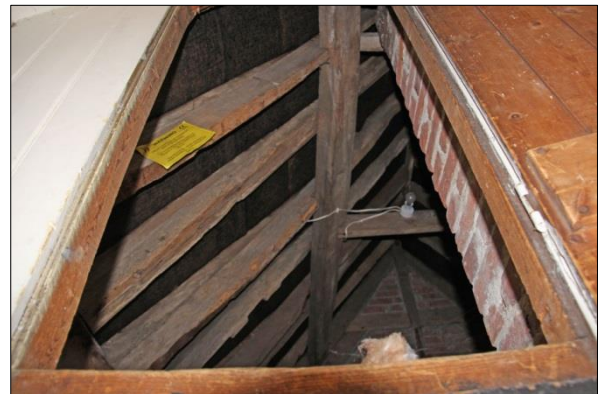
Plate 32: Roof space above F5, facing east (31)
