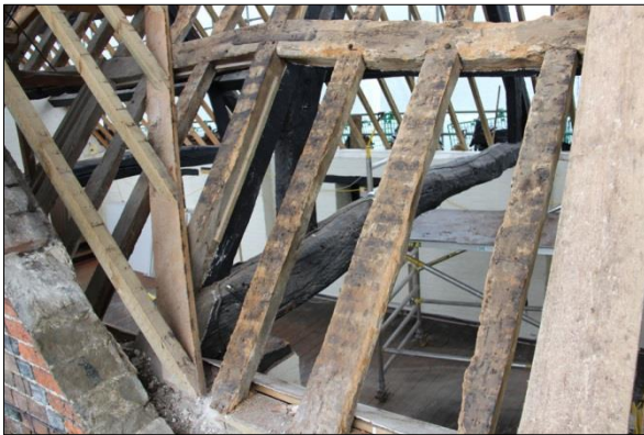
Plate 51: South roof, Truss 4 (105)
