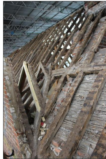
Plate 62: South roof, main chimney (116)
