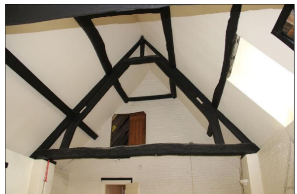
Plate 24: Truss 4, facing east (24)
