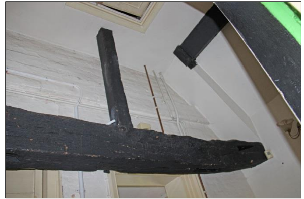
Plate 8: Truss 1, facing northwest (2)
