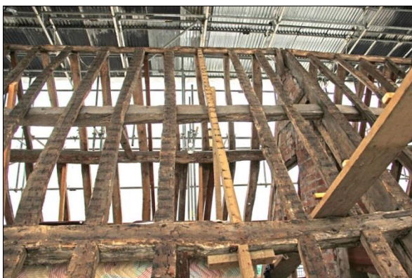
Plate 89: North roof, Bay 6 (70)
