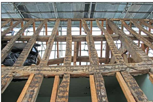
Plate 39: South roof, Bay 1 (89)
