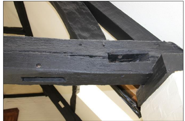
Plate 16: Truss 3 mortices, facing east (17)
