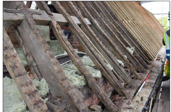
Plate 88: North roof, Bay 5 (69)
