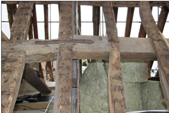
Plate 87: North roof, Truss 5 (68)
