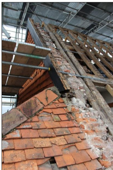
Plate 33: South roof, west gable and Truss 1 (84)
