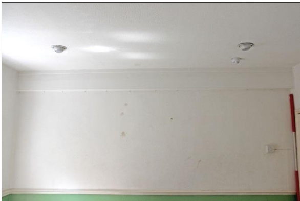
Plate 27: Truss 5 location in F6, facing west (27)
