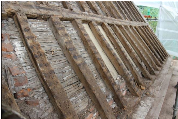
Plate 69: South roof, Bay 7 (119)
