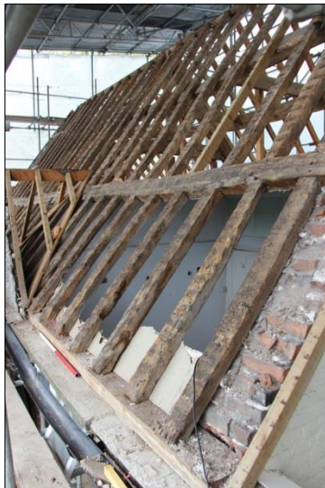
Plate 45: South roof, Bay 2 (98)
