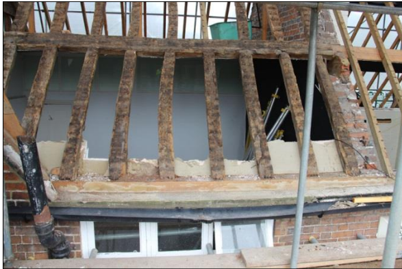
Plate 43: South roof, Bay 2 (95)
