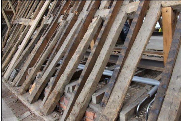
Plate 55: South roof, Bay 5 (109)
