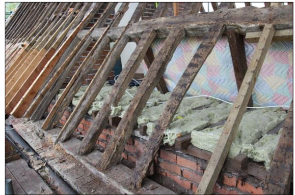
Plate 92: North roof, Bay 6 (73)
