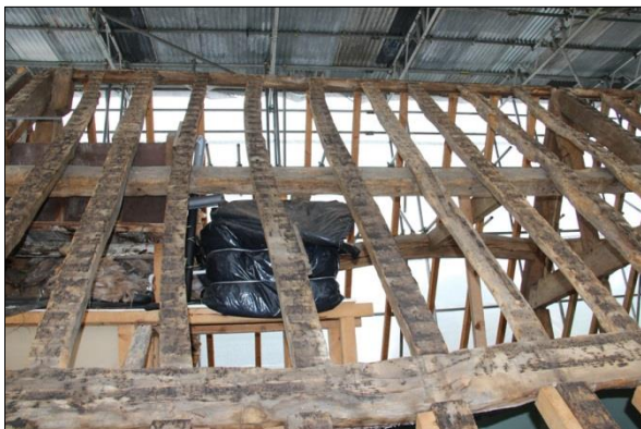
Plate 37: South roof, Bay 1 (88)
