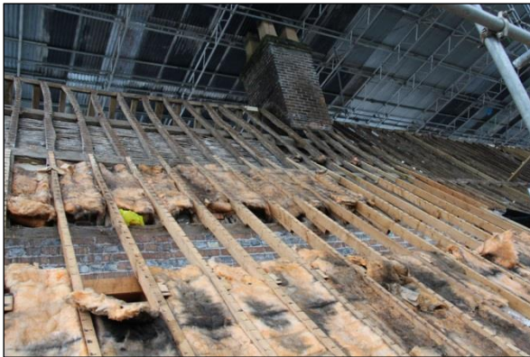
Plate 97: North roof, Bay 7 (82)
