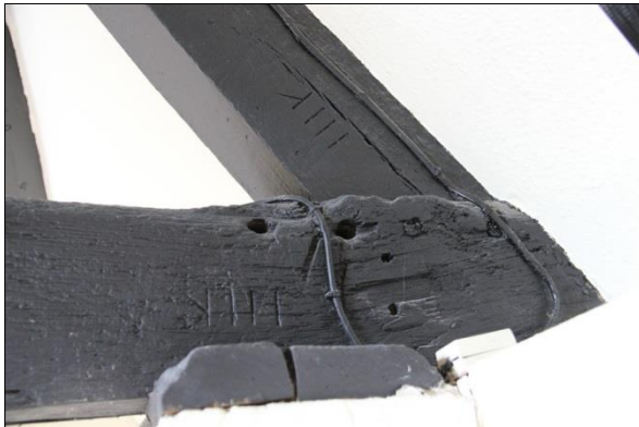
Plate 21: Truss 3 carpenter's marks, facing west (21)
