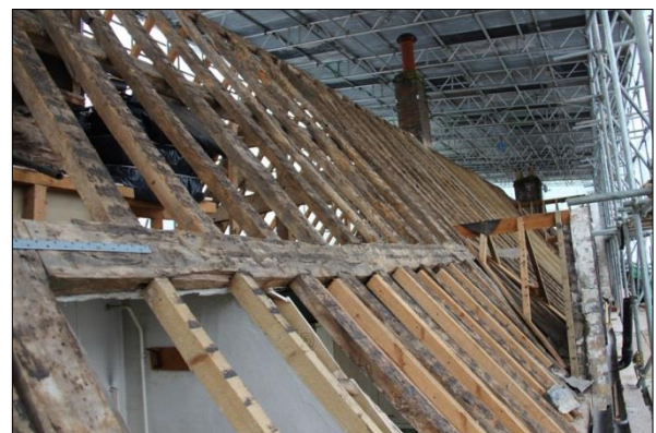
Plate 36: South roof, view to east(85)
