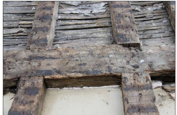
Plate 70: South roof, Bay 7 carpenter's marks (125)
