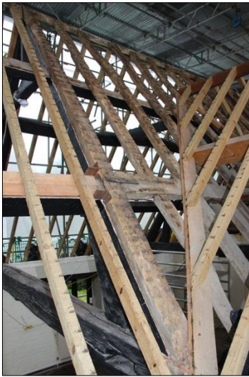
Plate 49: South roof, Truss 3 (102)
