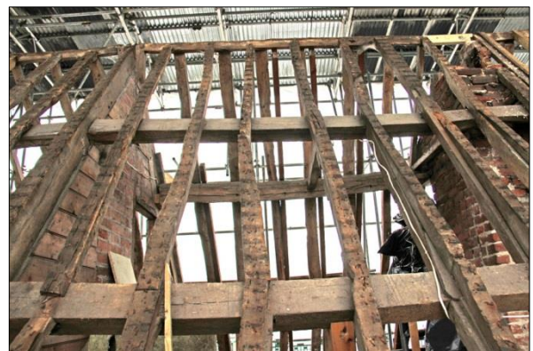
Plate 84: North roof, Bay 5 (65)
