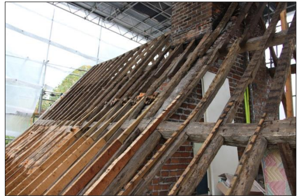
Plate 94: North roof, Bay 6 (74)
