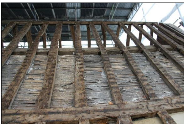
Plate 71: South roof, Bay 7 (122)
