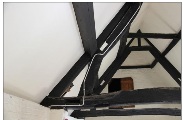
Plate 12: Truss 3, facing east (12)
