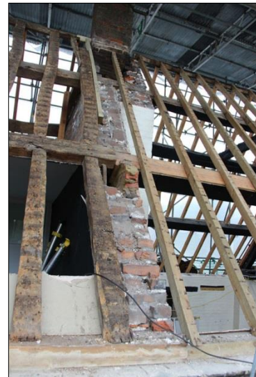
Plate 46: South roof, brick partition and chimney (96)
