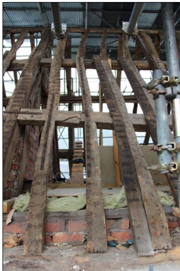
Plate 57: South roof, Bay 6 (111)
