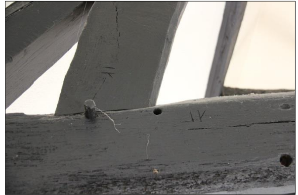
Plate 20: Truss 3 carpenter's marks, facing west (20)
