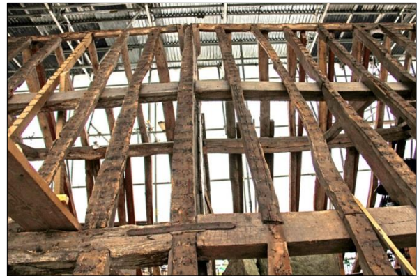
Plate 86: North roof, Truss 5 (67)
