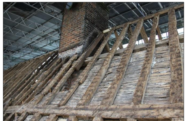
Plate 66: South roof, Bay 7 (127)
