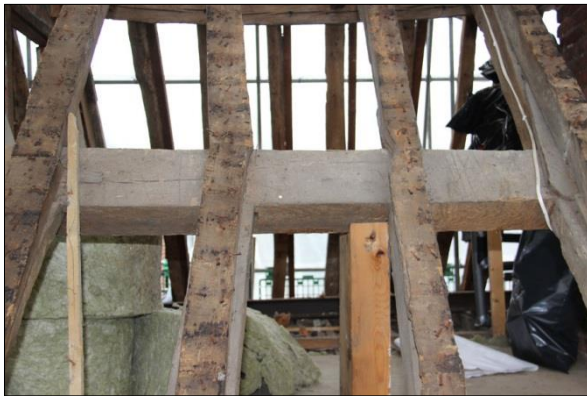
Plate 85: North roof, Bay 5 (66)
