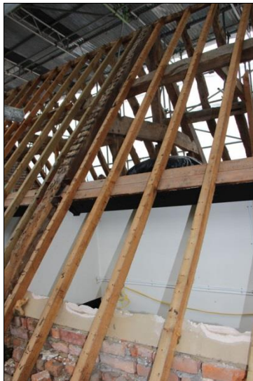
Plate 75: North roof, Bay 1 (51)
