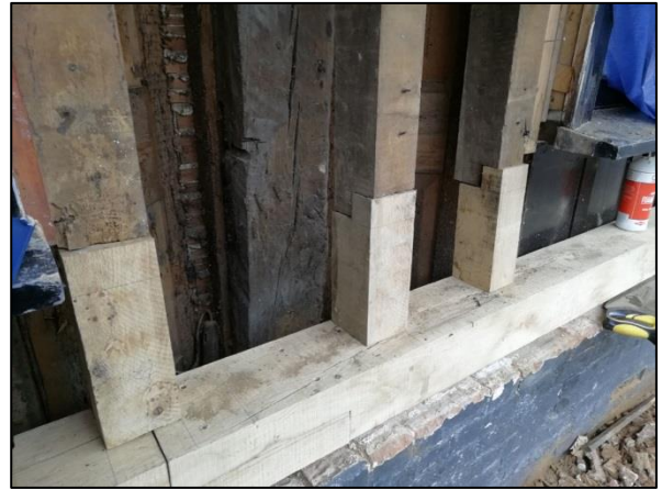
Plate 17: North wall: repairs to studs
