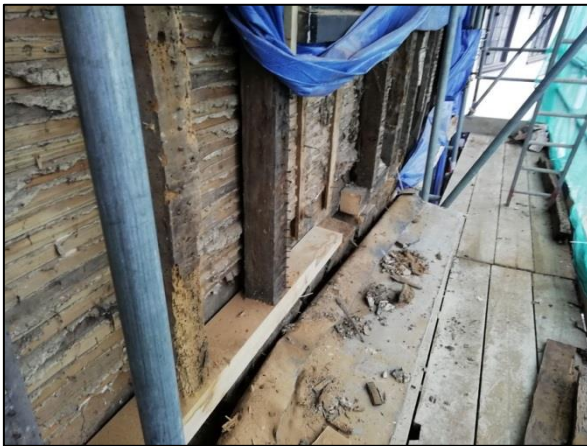
Plate 12: North wall: first floor studs looking west
