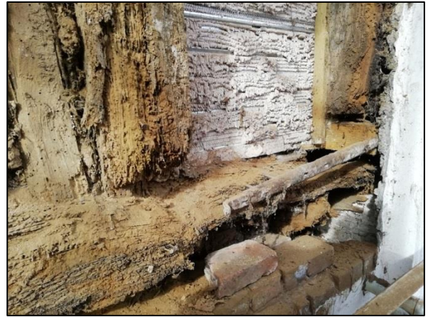
Plate 31: East wall: bressumer beam
