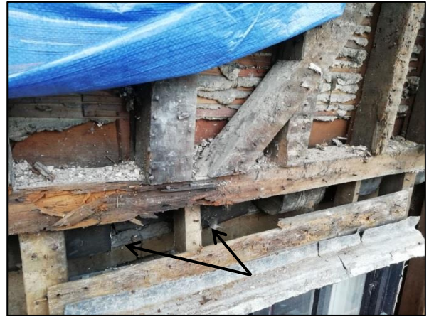
Plate 11: North wall; first floor joists
