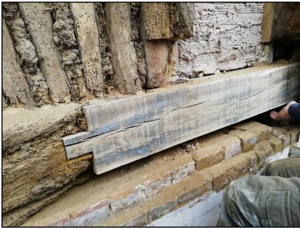
Plate 52: Wall plate repair
