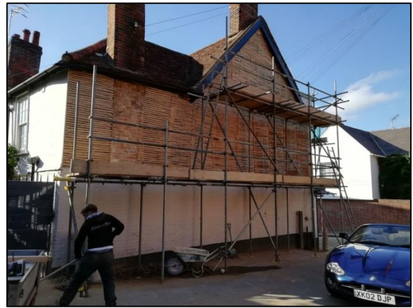
Plate 45: East elevation completed lath repair
