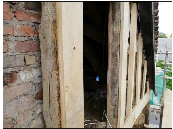
Plate 43: East wall: new studs in front of the original
