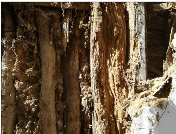
Plate 28: East wall: wattle and daub detail
