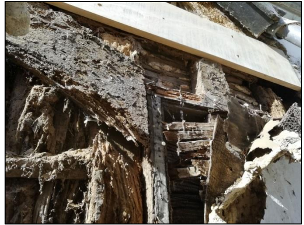
Plate 37: East wall: northern brace
