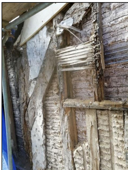
Plate 34: East wall: southern post
