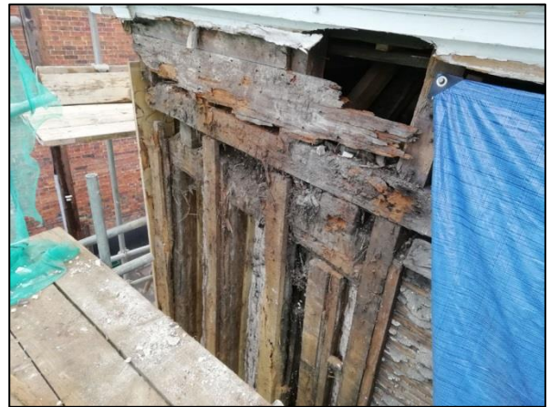
Plate 13: North wall: studwork at eastern end
