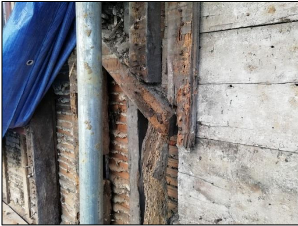
Plate 16: North wall: stud detail
