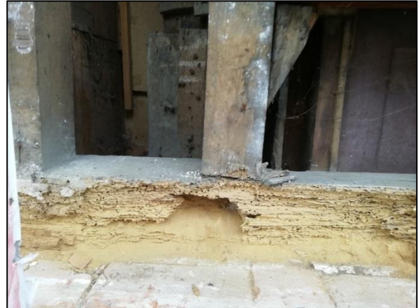
Plate 5: North wall: 18 th century sill beam with original walling behind
