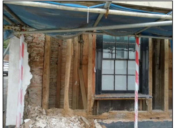
Plate 23: North elevation: ground floor eastern end
