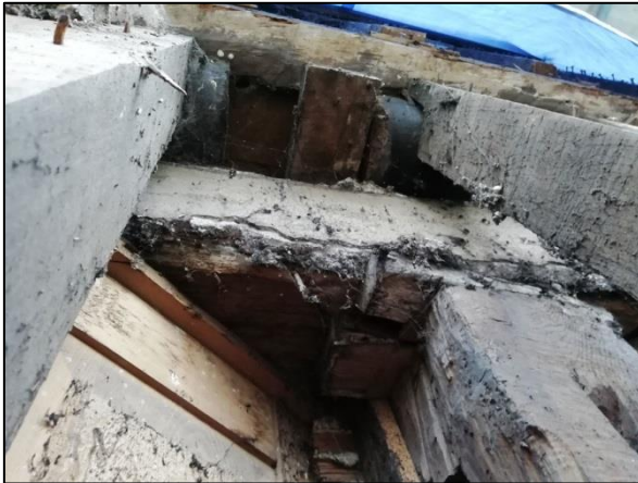
Plate 6: North wall; wallplate & first floor joists
