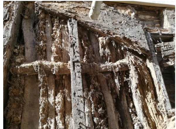
Plate 27: East wall: wattle and daub
