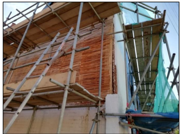
Plate 55: Detail of new laths
