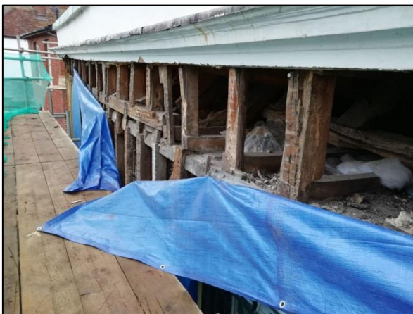
Plate 14: North wall: uppermost studs
