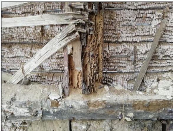
Plate 26: East wall: later plasterwork either side of an original stud
