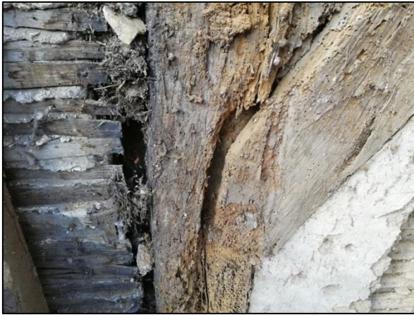
Plate 36: East wall: southern post with lath & plaster detail to the left
