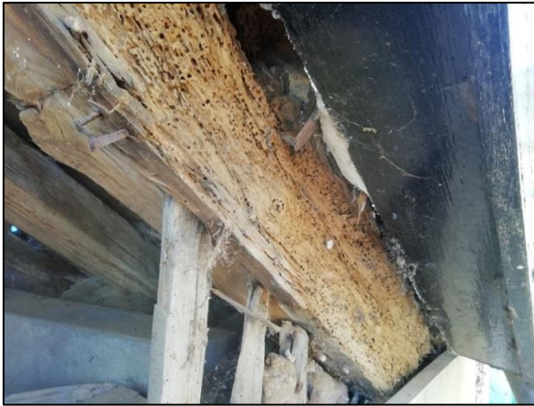
Plate 30: East wall: laths detail
