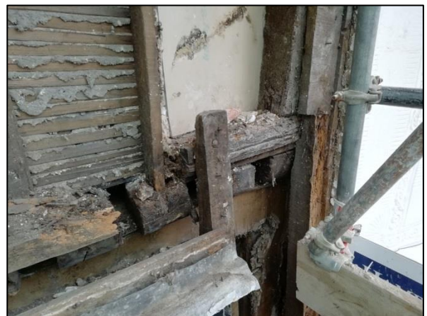
Plate 15: North wall: first floor west end
