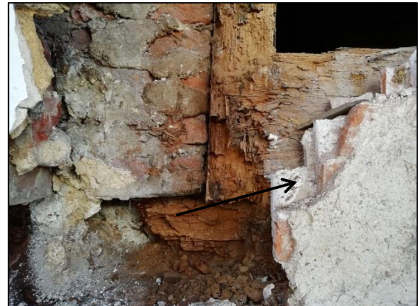
Plate 3: Mathematical tile on north wall
