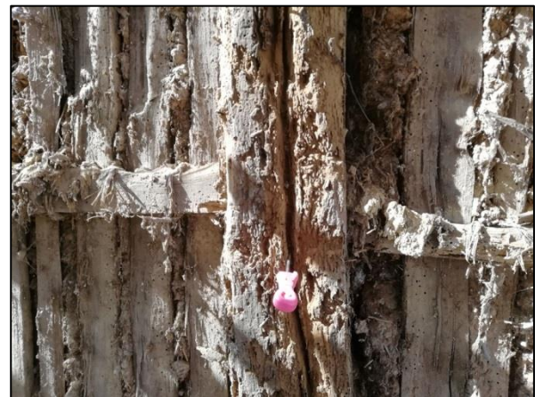
Plate 29: East wall: lath and plaster detail
