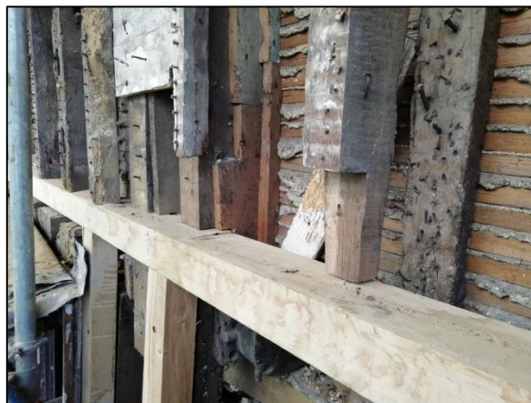
Plate 56: Ongoing repair to studs
