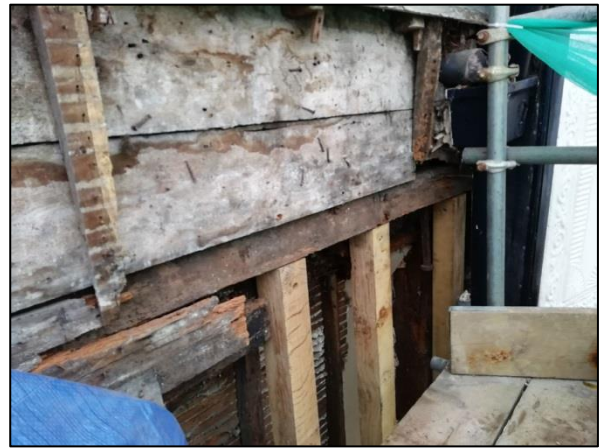
Plate 19: North wall: repairs
