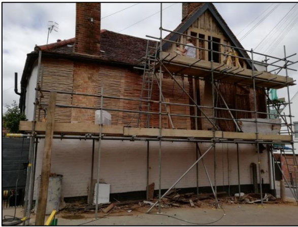
Plate 44: East elevation under repair
