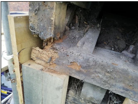
Plate 8: North elevation: eastern first floor corner
