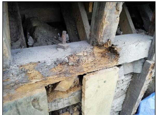
Plate 9: North elevation: wallplate
