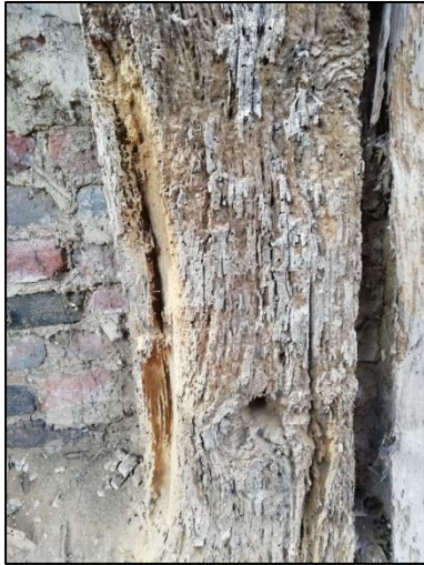
Plate 24: East wall: brickwork and stud detail looking north
