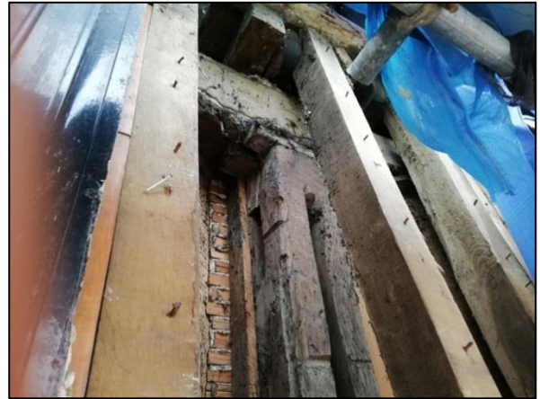
Plate 7: North elevation: original post and wallplate behind modern frame
