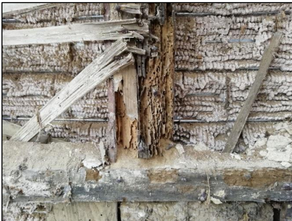
Plate 38: East wall: modern plaster and original stud
