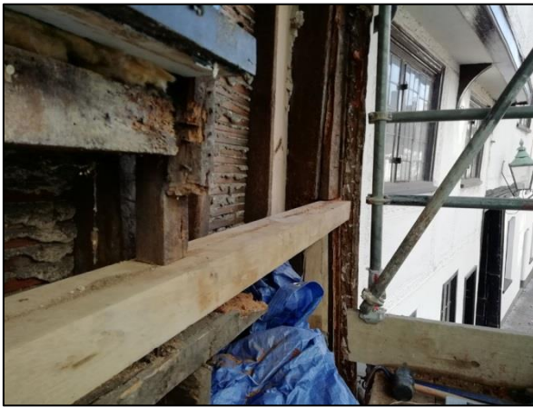
Plate 18: North wall: repairs
