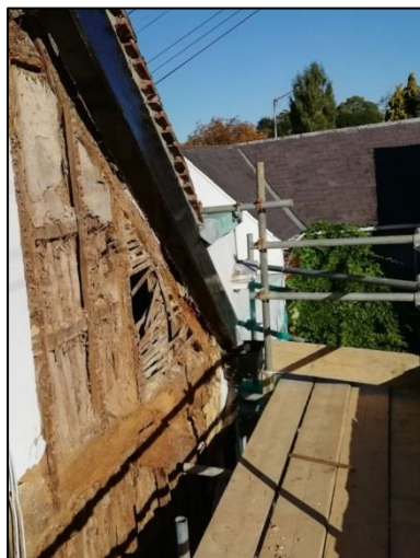
Plate 40: East wall: view to north
