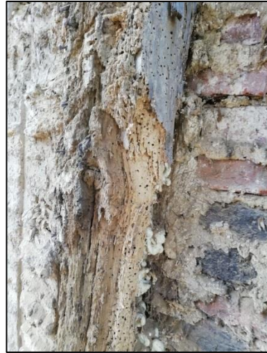
Plate 25: East wall: brickwork and stud detail looking south
