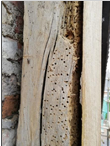
Plate 54: New stud in front of original, infested stud
