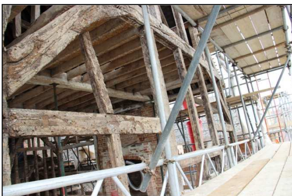
Plate 45: East elevation, external view from the southwest
