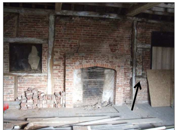
Plate 40: Remains of locked mullion window to the east of the fireplace
