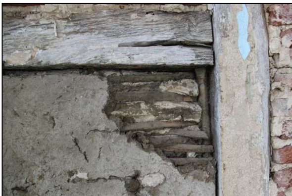
Plate 31: North elevation: wattle and daub detail
