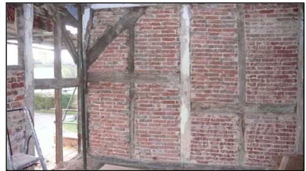
Plate 28: South elevation: west end before brick infill was removed
