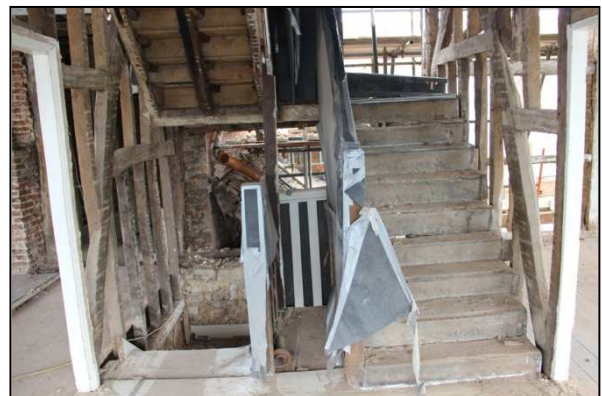
Plate 32: North elevation: stairs to upper and lower floors
