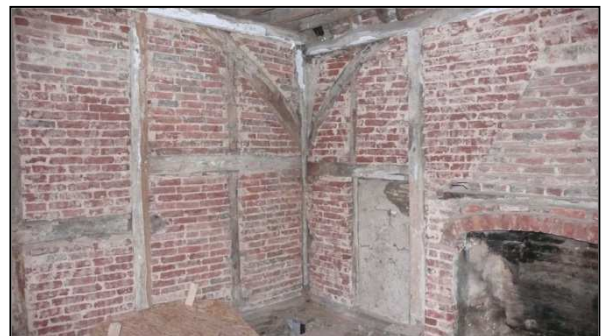
Plate 38: Northwest corner before the brick infill was removed
