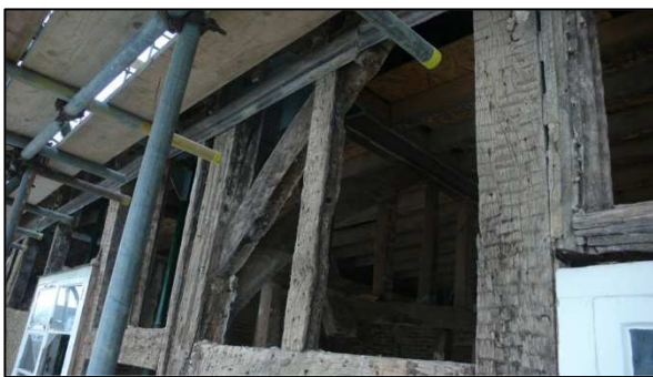
Plate 21: South elevation: panel 5 detail
