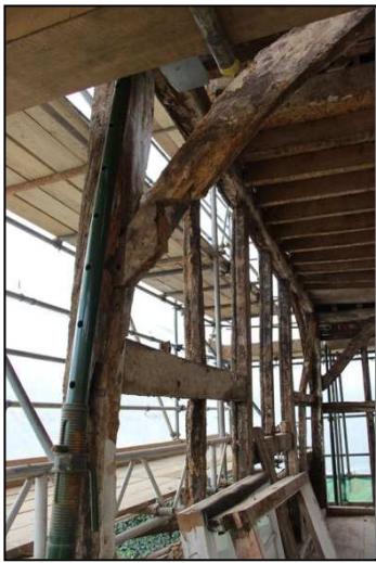
Plate 47: East elevation, northeast corner
