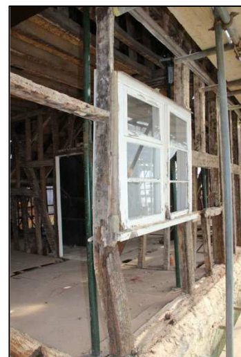
Plate 6: South elevation: panels 2-3
