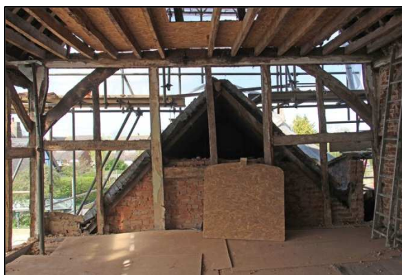
Plate 51: West gable end
