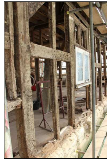
Plate 8: South elevation: panels 4-5
