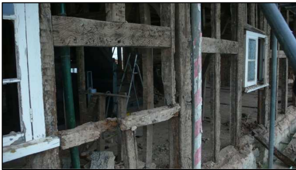
Plate 25: South elevation: panel 4 detail
