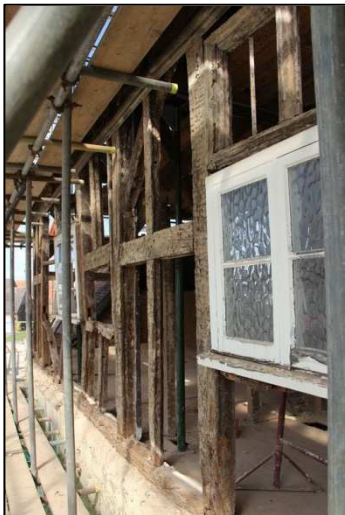
Plate 15: South elevation: view from the east
