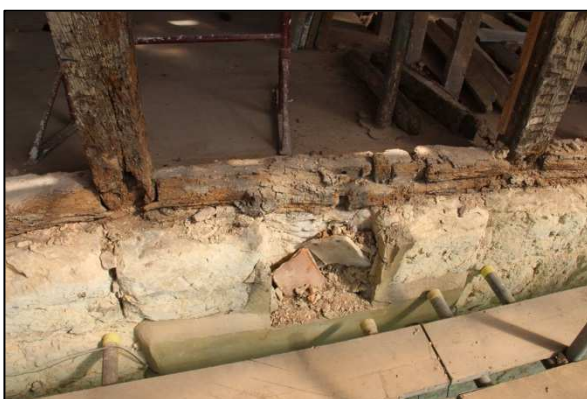
Plate 11: South elevation: bressumer beam in panel 6
