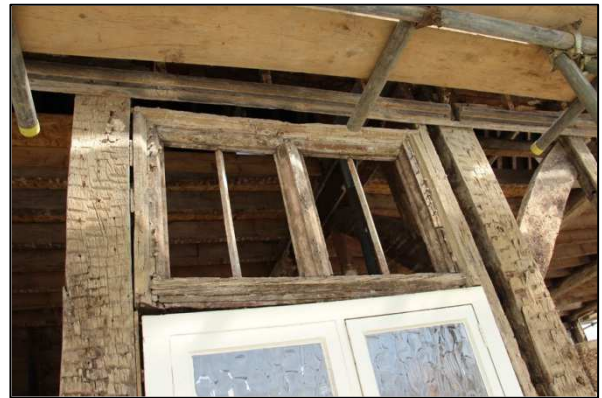
Plate 10: South elevation: timber mullioned window in panel 6
