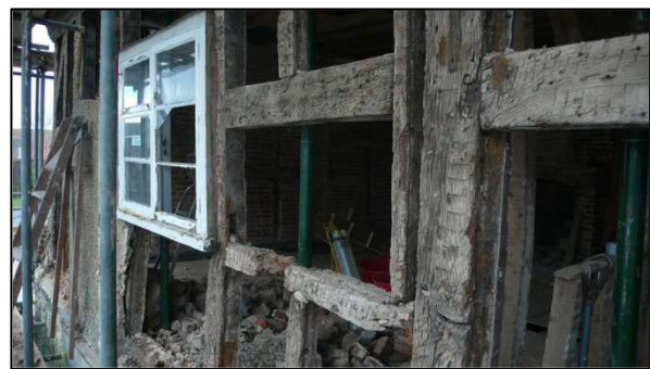
Plate 22: South elevation: evidence for earlier window in panel 4
