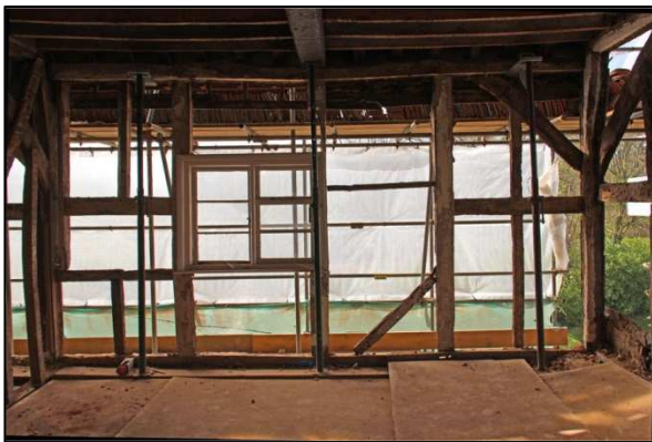
Plate 3: South elevation: west end
