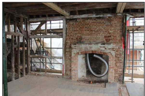
Plate 34: North elevation: east end
