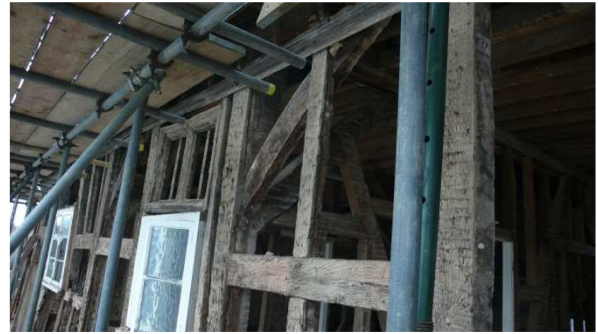
Plate 20: South elevation: stud in panel 8 without V groove
