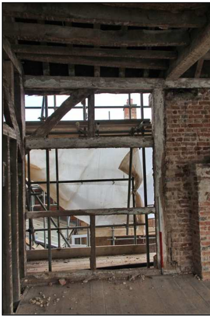
Plate 35: North elevation: timberwork detail, east end
