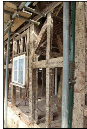
Plate 14: South elevation: panels 6-7 from the east
