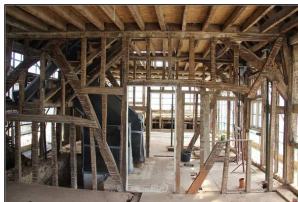
Plate 50: Partition between western room and landing
