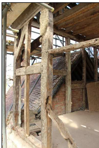
Plate 5: South elevation: panels 1-2
