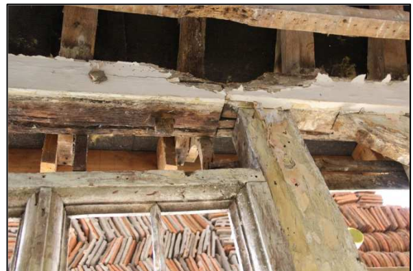
Plate 18: South elevation: bridle butted scarf joint
