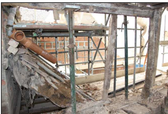
Plate 33: North elevation: timberwork behind the staircase
