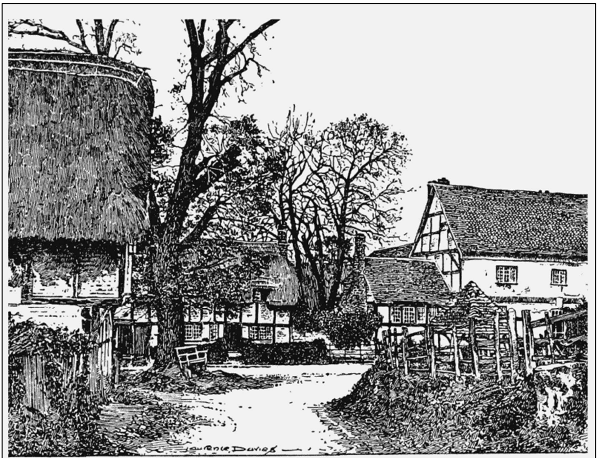
Figure 4: New Farm from the southwest in the early 20 th century (reproduced from VCH)
