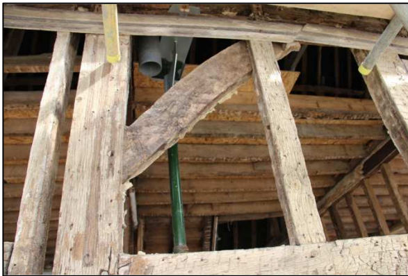
Plate 9: South elevation: brace in panel 5
