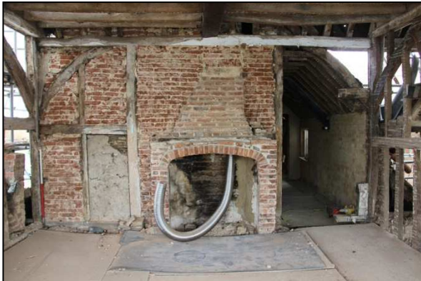
Plate 29: North elevation: west end
