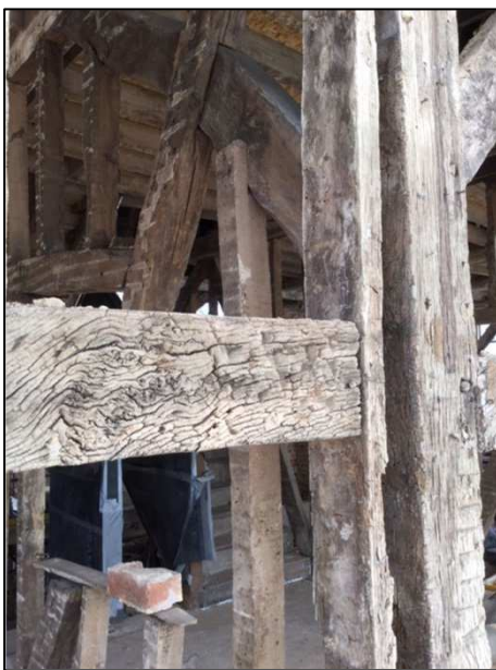
Plate 27: South elevation: eastern side of former window
