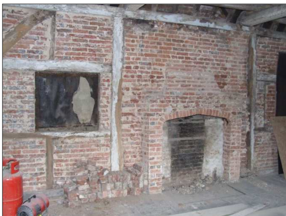
Plate 39: Blocked mullion window to the left of the fireplace
