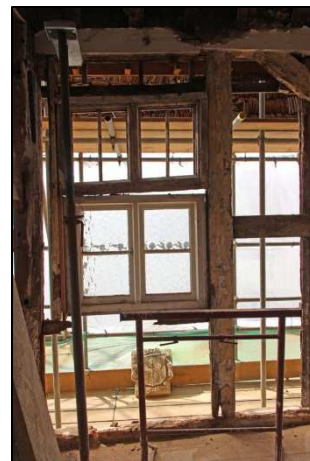
Plate 4: South elevation: window detail
