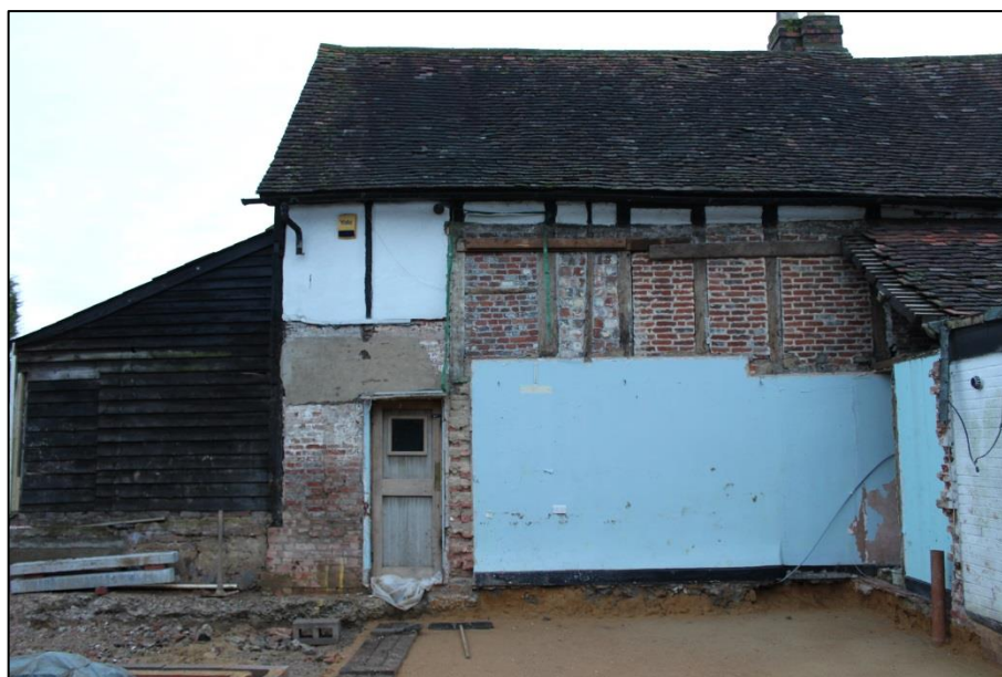
Plate 1: Rear/west elevation, looking east
