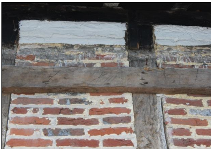
Plate 3: Carpenter mark 'XIII' on brace
