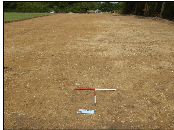
Plate 2: Initial topsoil strip, looking NW (scale 2x1m)
