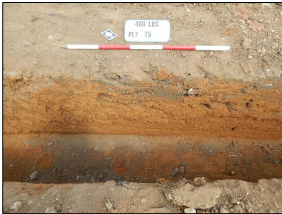
Plate 27: Footing trench 5, plot 7, looking northeast
