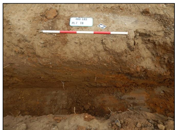
Plate 30: Footing trench 8, plot 7, looking northeast
