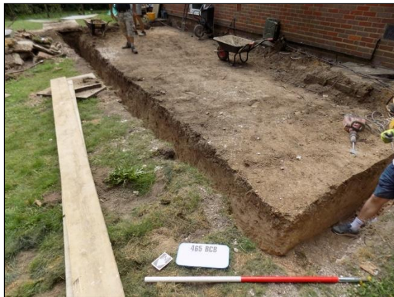
Plate 1: Footing trenches, looking southeast
