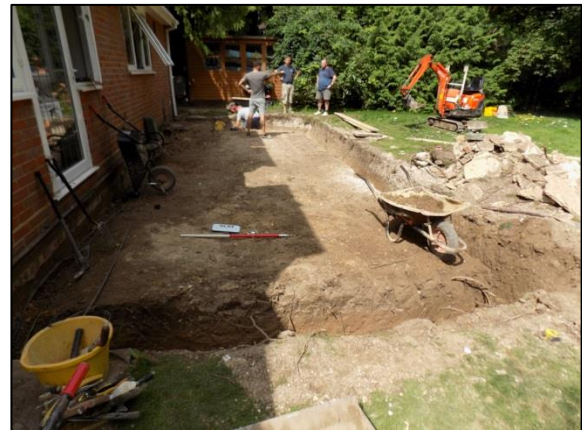
Plate 2: Footing trenches, looking northwest
