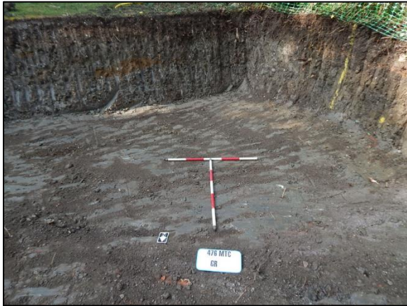
Plate 1: Ground reduction area, facing south
