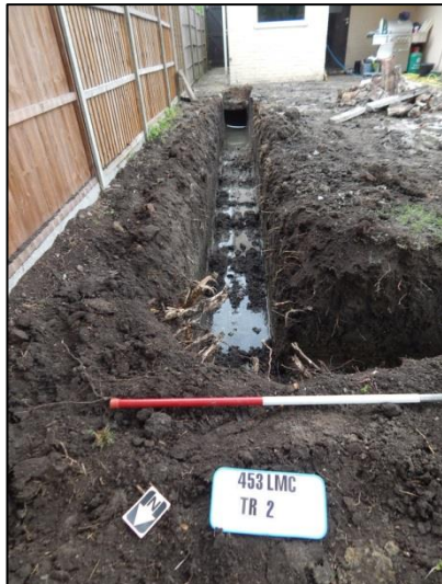
Plate 3: Trench 2, looking southeast
