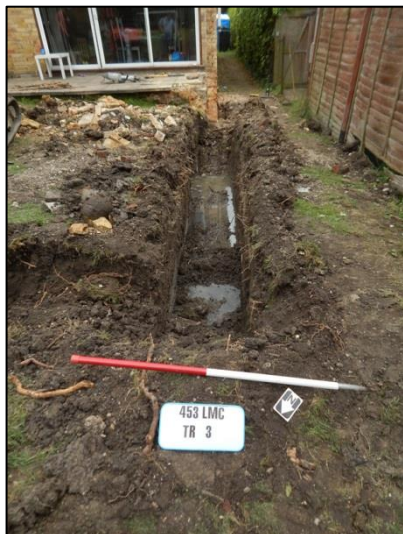
Plate 5: Trench 3, looking southeast
