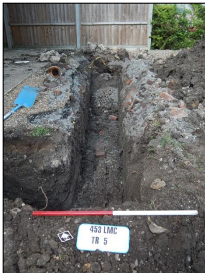
Plate 9: Trench 5, looking northeast
