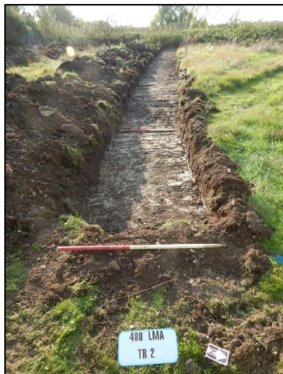
Plate 3: Trench 2, looking southwest
