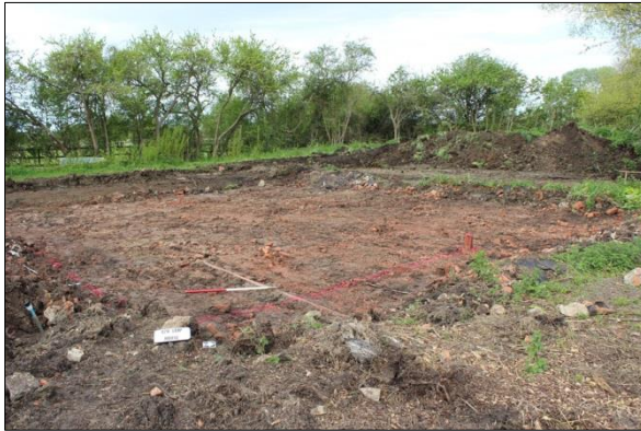
Plate 1: Reduced footprint for house, looking west
