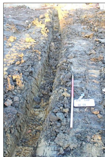
Plate 6: Service trench, looking west-northwest
