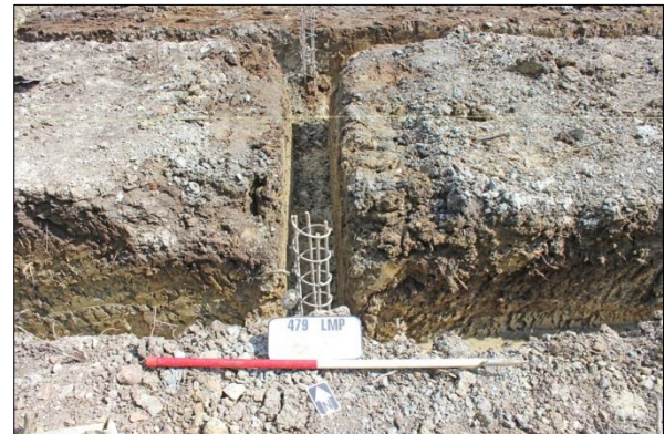
Plate 4: Interior house foundation trench, looking north-northeast
