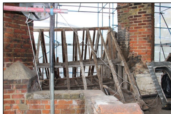
Photo 248: R14: Roof 5, facing west
