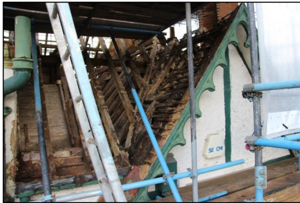
Photo 237: R3: Roof 1, facing southwest
