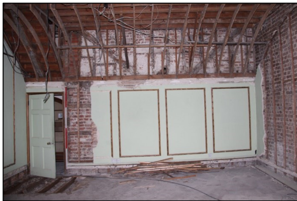
Photo G41: G3: North wall partially stripped
