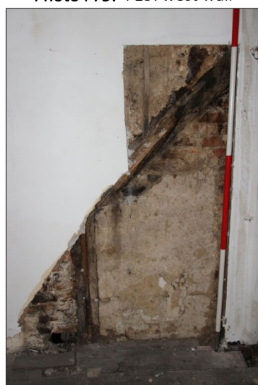
Photo F81: F15: detail of timber framing in north wall
