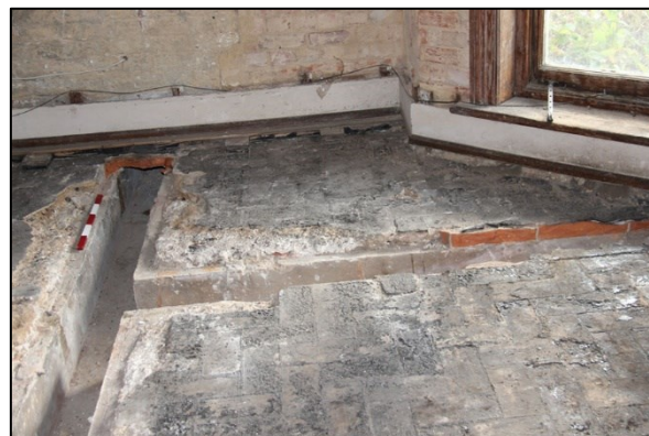
Photo G50: G4: channels within the concrete
