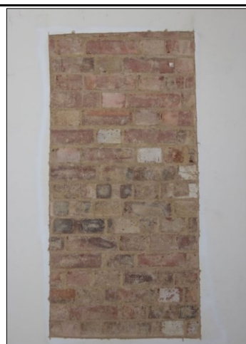
Photo G2: G1: detail of exposed brick on south wall
