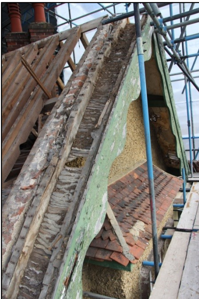
Photo 245: R11: Roof 5, facing northeast
