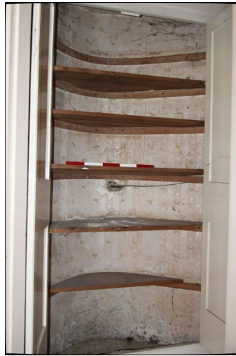
Photo S5: S1: curved-back cupboard outside S5, facing northwest
