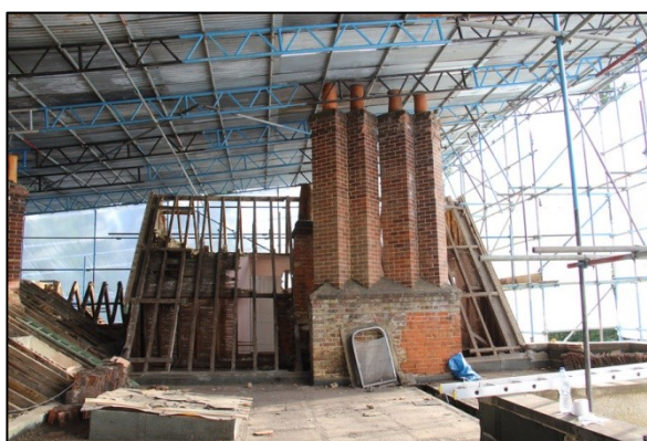
Photo 253: R19: Roof 6, facing east
