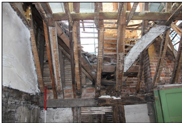
Photo F68: F11: south end of roof, facing west
