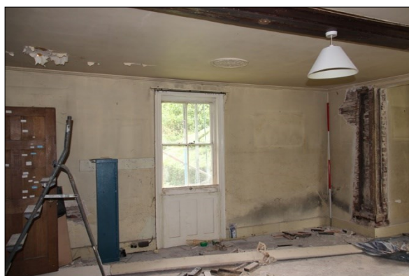
Photo G23: G2: North wall
