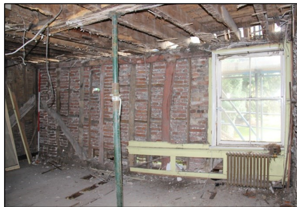
Photo F30: F4: east wall stripped
