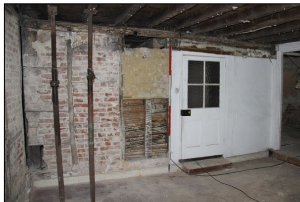
Photo G83: G11: east wall stripped
