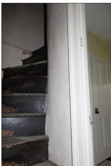
Photo S1: S1: bottom of stair to second floor (S01)
