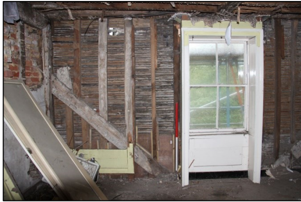
Photo F33: F4: west end of north wall stripped
