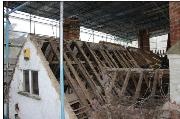
Photo 240: R6: Roof 3, facing northeast
