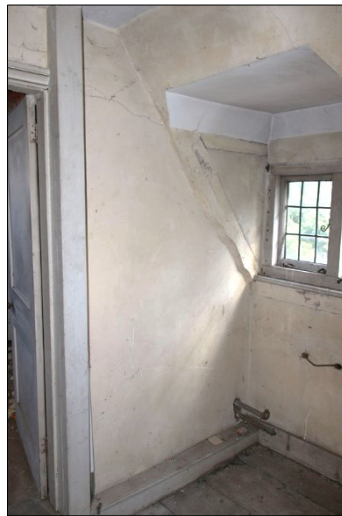
Photo S10: S2: northeast corner of room, facing northeast
