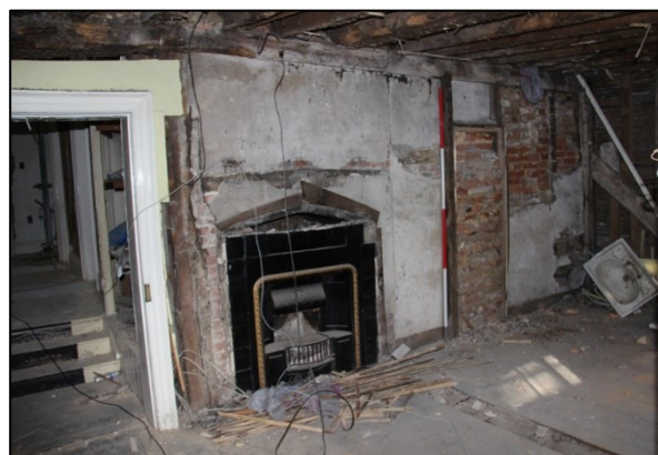
Photo F32: F4: west wall stripped
