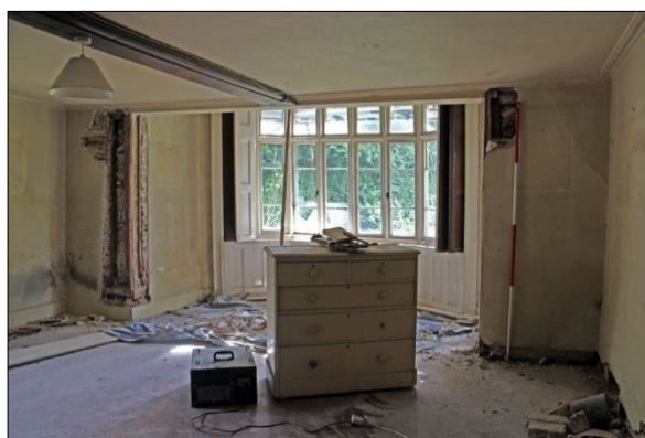
Photo G21: G2: East wall, facing northeast
