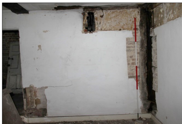
Photo G75: G11: north wall
