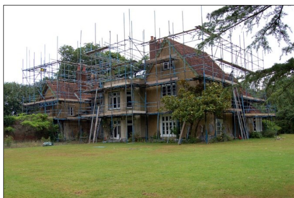
Photo 1: South elevation, facing northwest
