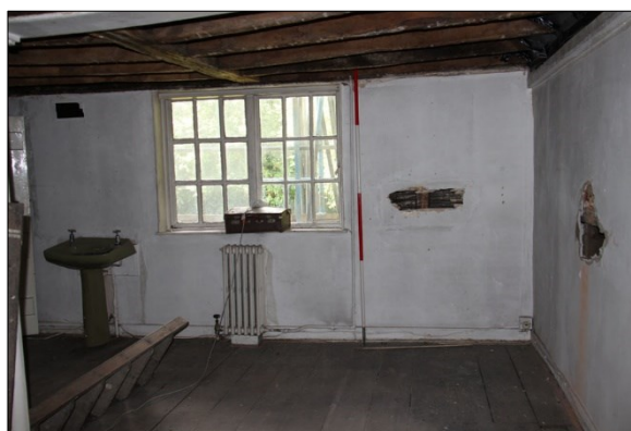
Photo F79: F15: west wall
