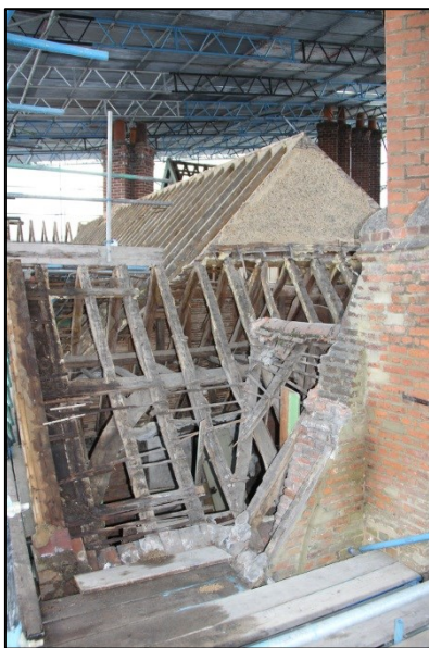
Photo 239: R5: Roof 2, facing southeast
