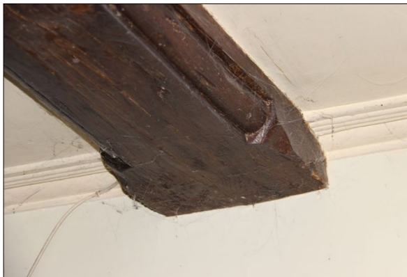
Photo G27: G2: Spinal beam, facing southwest
