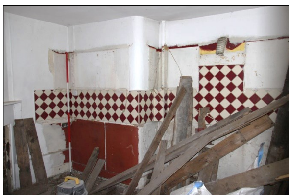
Photo G94: G16: south wall, facing southeast
