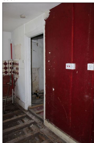
Photo G97: G16: north wall, facing northwest
