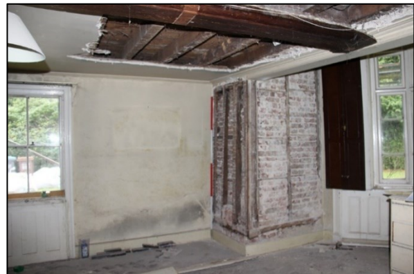
Photo G34: G2: North east corner partially stripped
