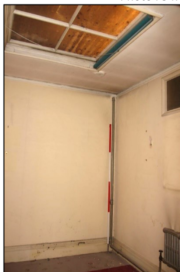
Photo F55: F9: northeast corner, skylight above
