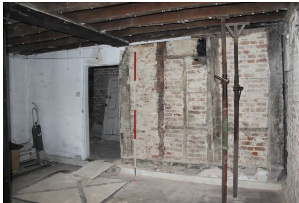
Photo G82: G11: north wall partially stripped
