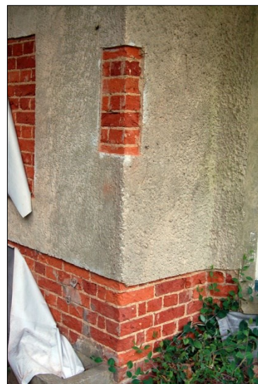
Photo 6: Exposed brick on south elevation (G4)
