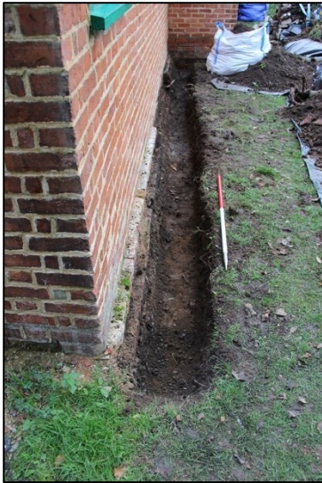
Plate 2: French drain to the south of the outbuilding
