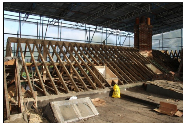
Photo 252: R18: Roof 1, facing northeast
