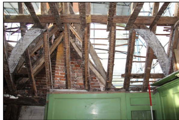
Photo F69: F11: north end of roof, facing west
