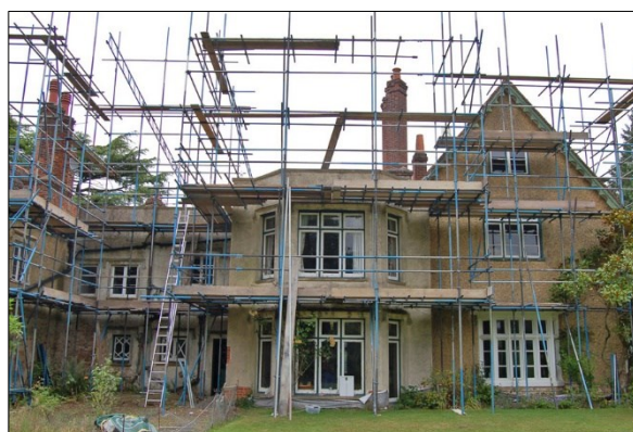
Photo 2: South elevation, facing north
