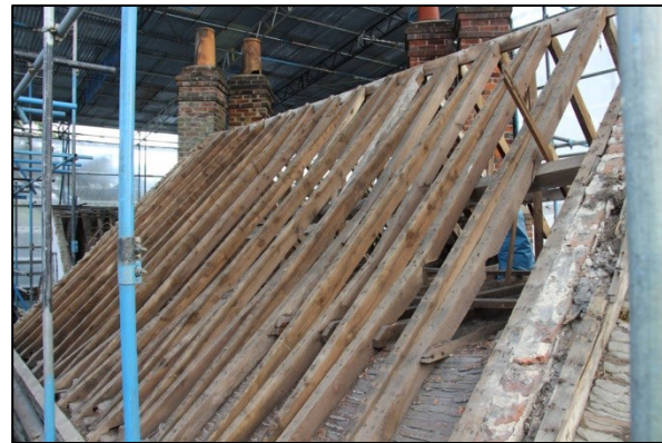
Photo 244: R10: Roof 5, facing northeast
