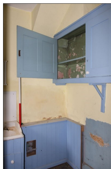
Photo G54: G6: facing northeast
