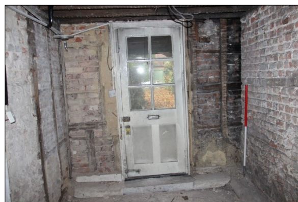
Photo G72: G10: west wall
