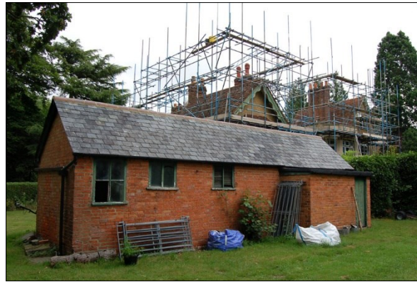
Photo 7: Outbuildings, view facing northeast
