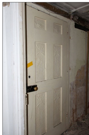
Photo G87: G13: detail of door into G14a, facing southeast
