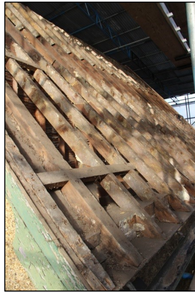
Photo 256: R22: Roof 6, facing northwest
