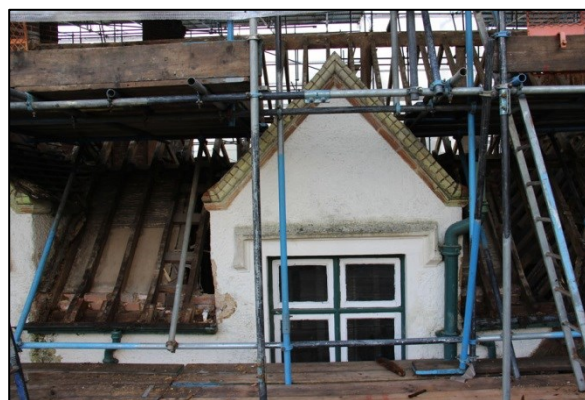
Photo 236: R2: Roof 1, facing southwest
