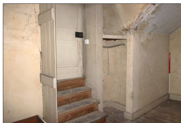
Photo S7: S2: south wall with steps to S01
