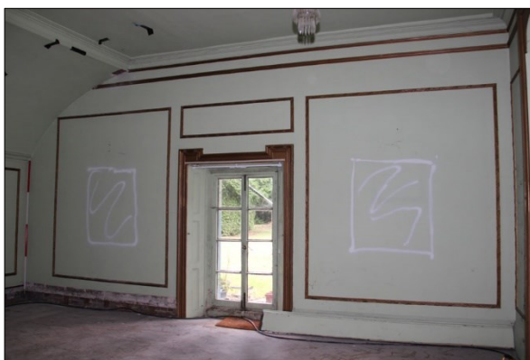
Photo G39: G3: East wall
