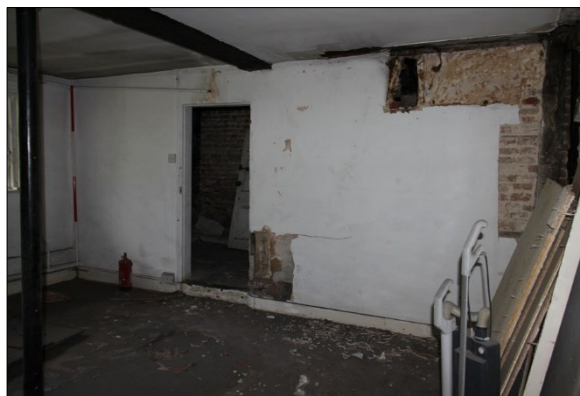
Photo G81: G11: north wall
