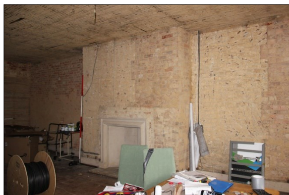
Photo G47: G4: east wall
