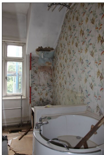
Photo F15: F2: east and north walls, facing northeast
