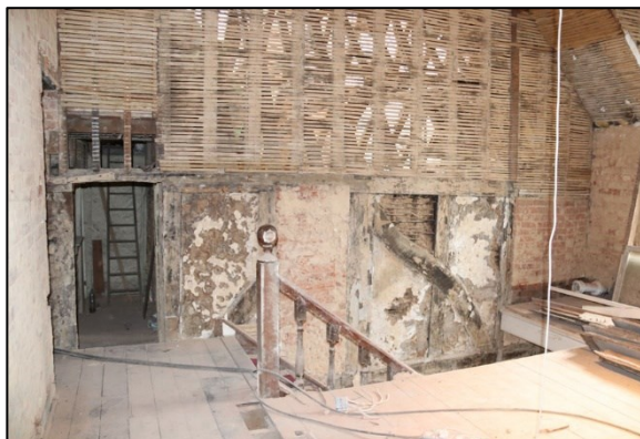
Photo F13: F1: east wall stripped
