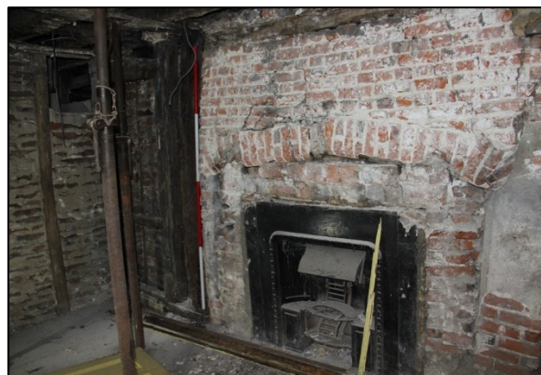
Photo G64: G8: southwest corner
