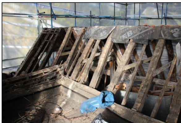
Photo 251: R17: Roof 3, facing northwest
