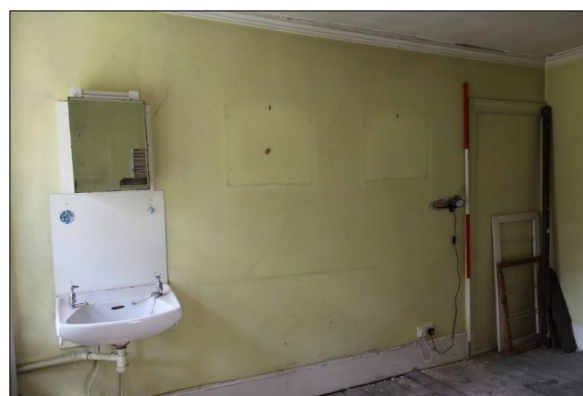
Photo F36: F5: south wall
