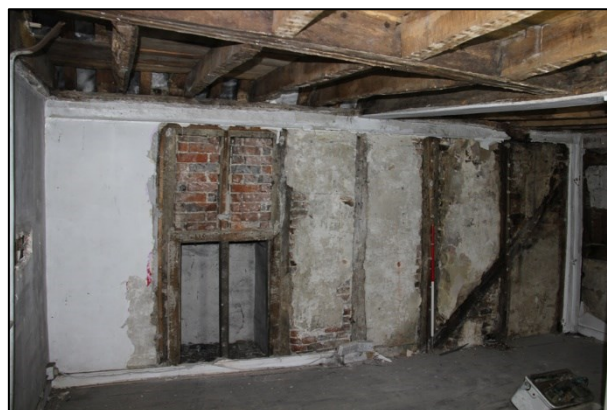
Photo F87: F15: south wall stripped
