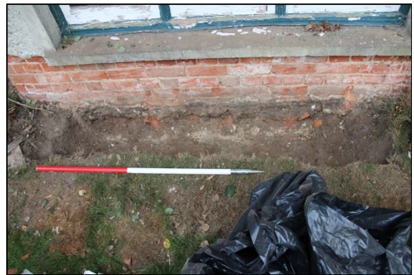
Plate 5: Brick footing beneath G4
