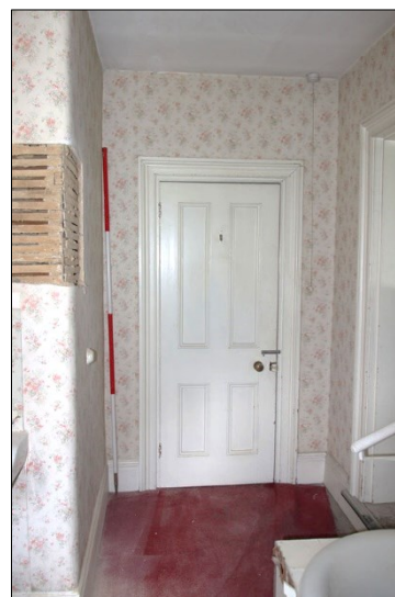
Photo F57: F10: facing north, door to F1
