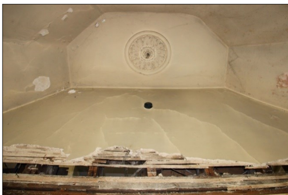
Photo G29: G2: Ceiling rosette in ceiling of bay on east
