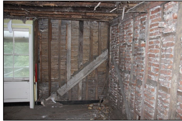
Photo F34: F4: east end of north wall stripped
