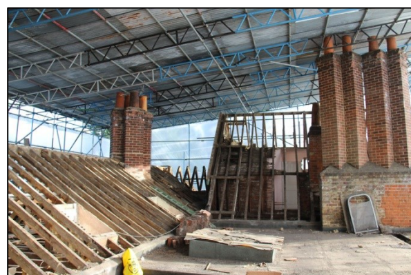
Photo 254: R20: Roofs 1 & 6, facing east
