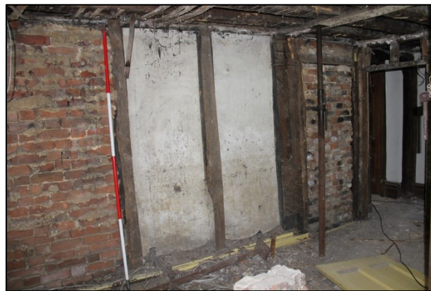
Photo G67: G8: east wall stripped
