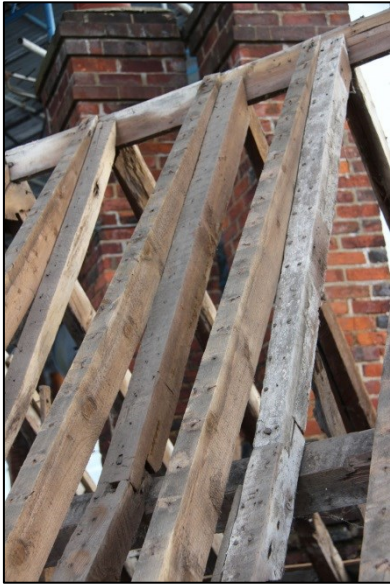
Photo 243: R9: Roof 5, facing east
