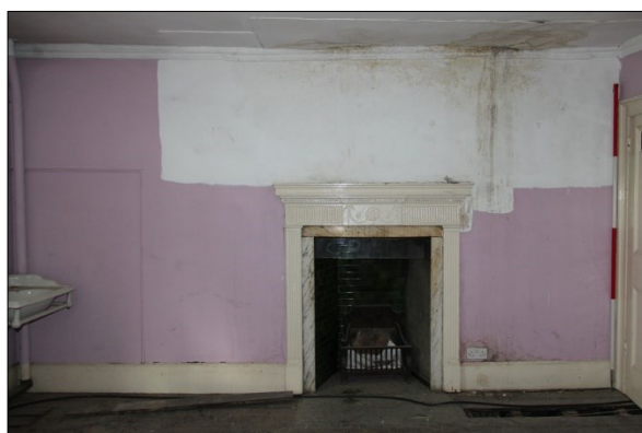
Photo F42: F6: west wall
