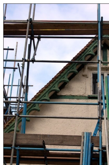
Photo 17: Detail of barge boards on east gable
