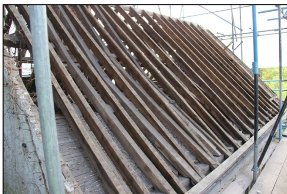
Photo 241: R7: Roof 5, facing southeast
