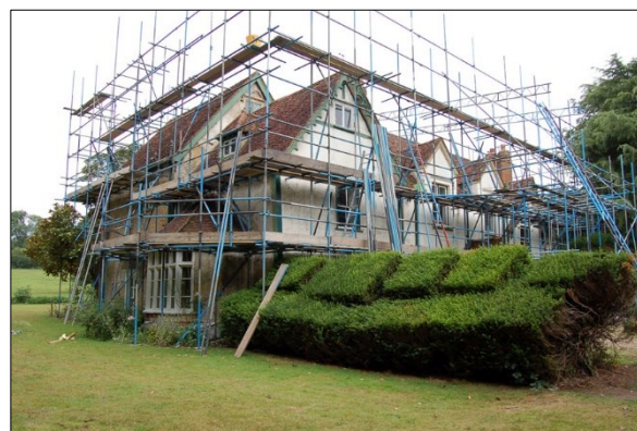
Photo 15: Detail of framing on eastern end
