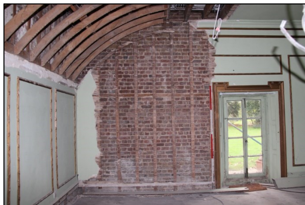
Photo G43: G3: East wall partially stripped
