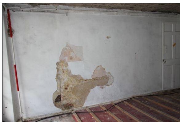
Photo G91: G15: north wall
