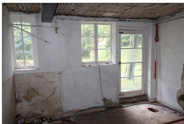
Photo G90: G15: west wall
