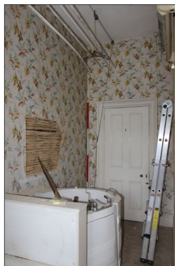
Photo F16: F2: east and south walls, facing southeast
