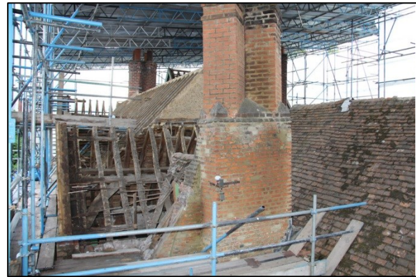
Photo 238: R4: Roof 2, facing east
