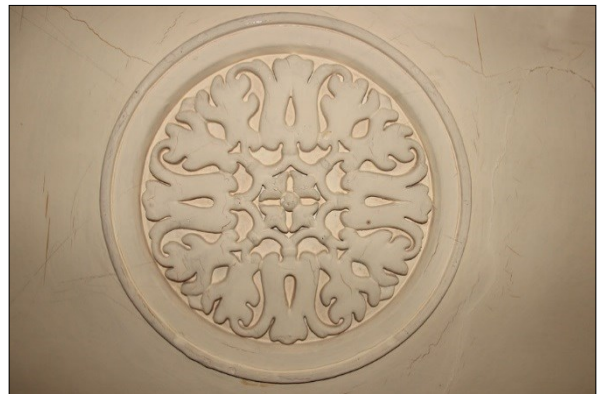
Photo G28: G2: Ceiling rosette to south of beam
