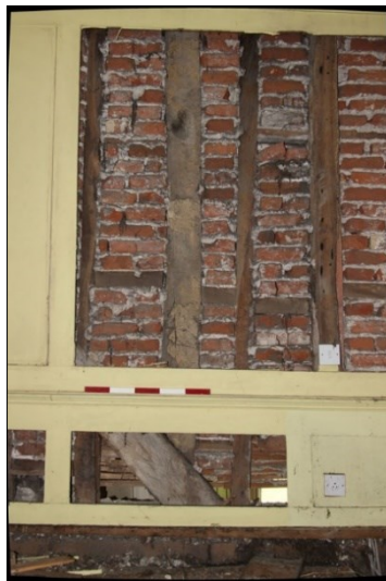
Photo F29: F4: detail of timberwork, east wall
