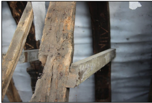
Photo 255: R21: Roof 3, facing north
