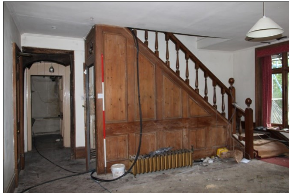
Photo G3: G1: west wall with staircase
