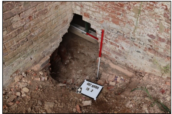
Plate 17: Trench 3 from site southeast
