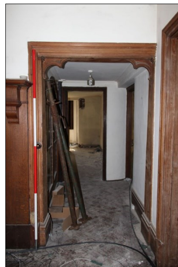
Photo G8: G1: detail of framing to east passage
