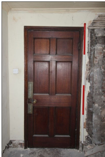
Photo G25: G2: Door to G1, west wall
