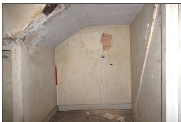
Photo S8: S2: west wall
