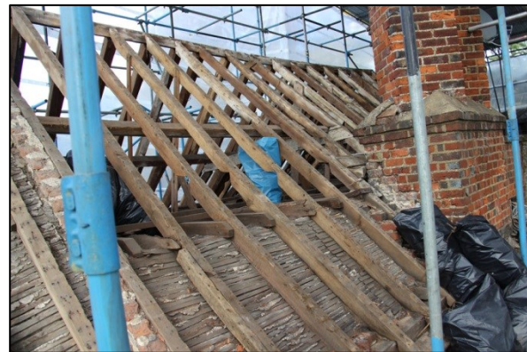
Photo 246: R12: Roof 5, facing northwest
