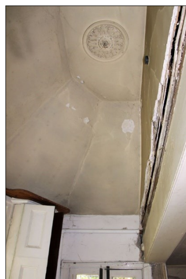
Photo G30: G2: Ceiling in eastern bay
