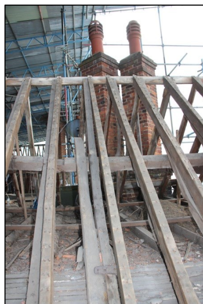
Photo 242: R8: Roof 5, facing east
