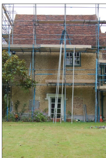
Photo 10: South half of east elevation
