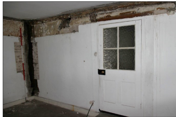
Photo G78: G11: east wall, facing northeast
