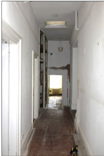
Photo F3: F1: view to east
