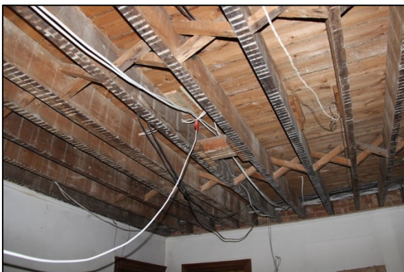
Photo G19: G1: ceiling detail
