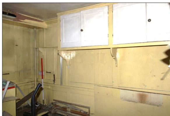
Photo G58: G8: east wall
