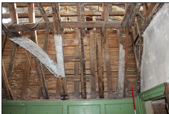
Photo F70: F11: south end of roof, facing east
