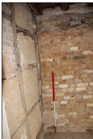
Photo G88: G14: northeast corner
