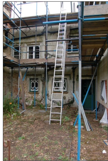
Photo 4: Central section of south elevation
