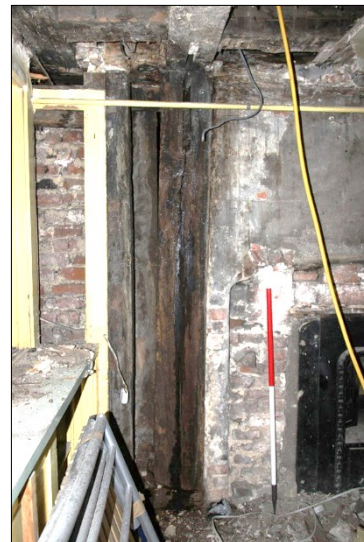
Photo G62: G8: detail of timberwork south of fireplace
