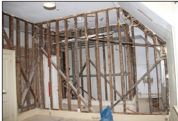
Photo F10: F1-3: 19 th century partitioning
