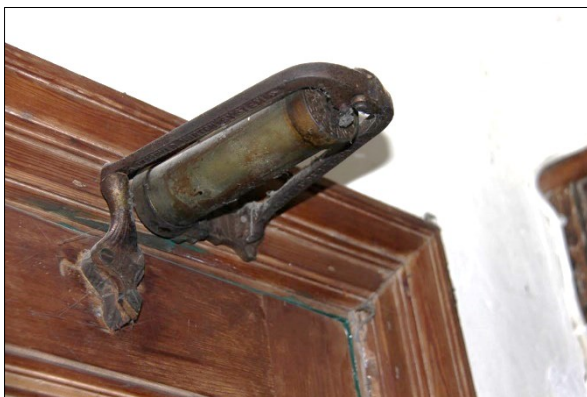
Photo G17: G1: automatic door closer on door to G5
