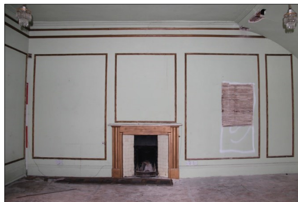
Photo G36: G3: West wall
