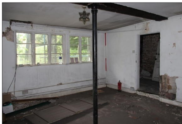
Photo G79: G11: west and north walls, door to G10
