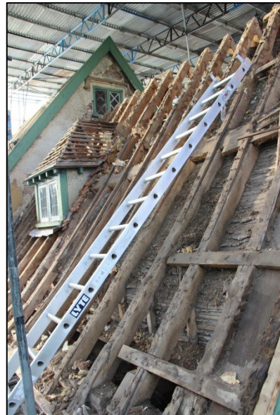
Photo 258: R24: Roof 7, facing southwest
