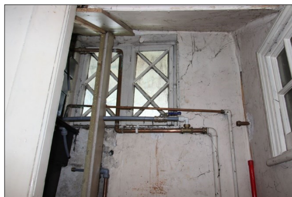
Photo S4: S1: windows above stairs, facing north
