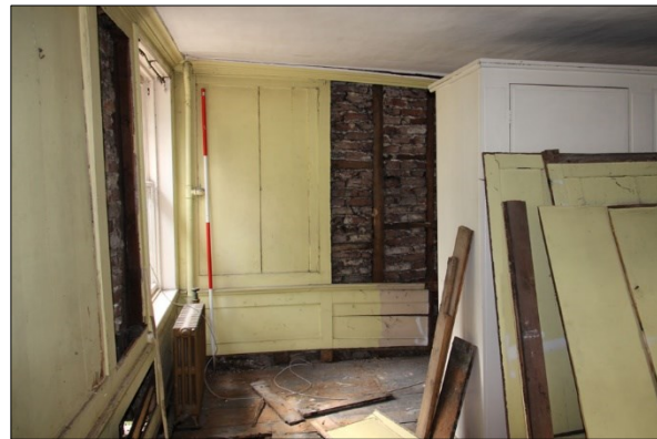
Photo F26: F4: east end of south wall
