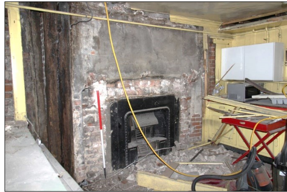
Photo G60: G8: west wall
