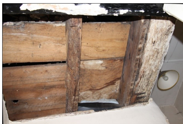
Photo F95: F17: detail of ceiling at north end of F17
