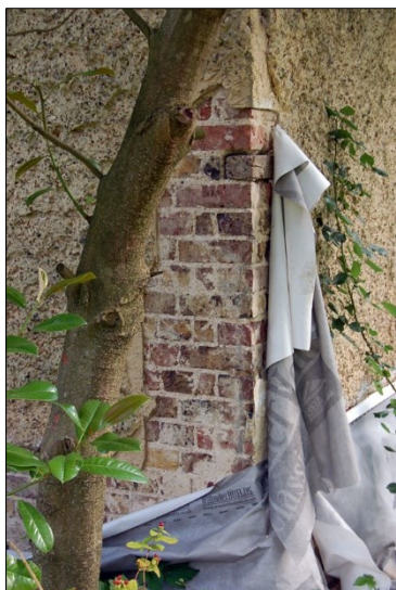
Photo 5: Exposed brick in southeast corner (G3)
