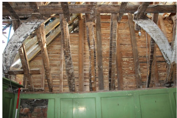
Photo F71: F11: north end of roof, facing east
