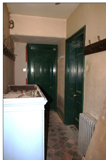
Photo G52: G5: Facing north, door to G4 on right, door to G1 at end
