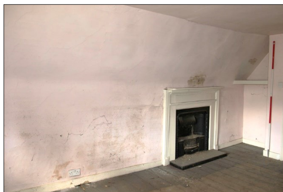
Photo S14: S5: west wall
