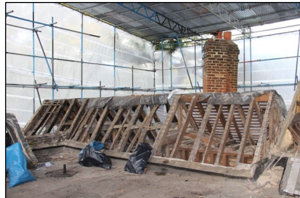
Photo 250: R16: Roof 3, facing northwest
