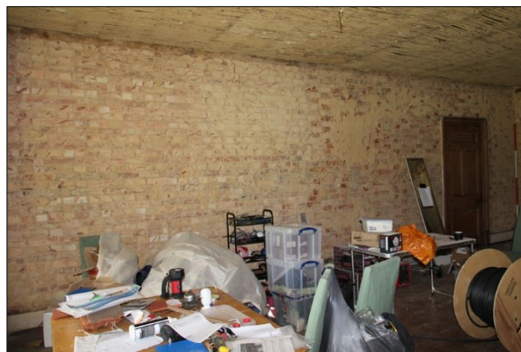
Photo G45: G4: west wall
