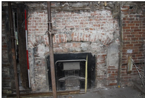
Photo G61: G8: detail of fireplace, west wall
