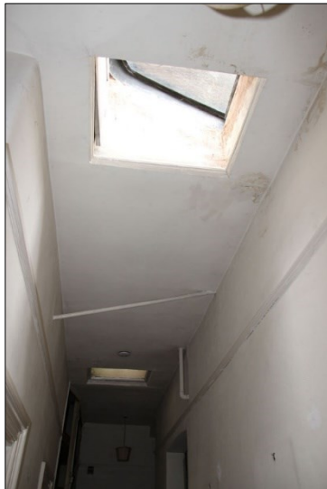
Photo F5: F1: skylight at west end of hall
