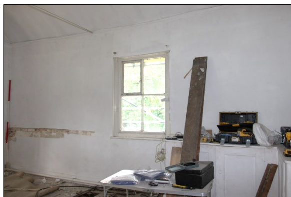
Photo F89: F16: west wall
