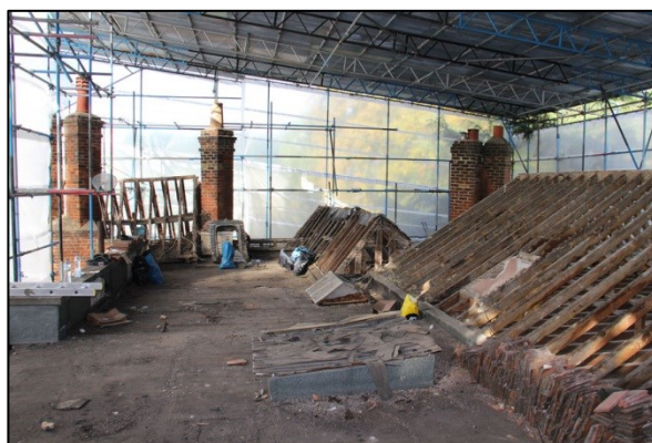
Photo 235: R1: Roofs 1, 3 - 5, facing west
