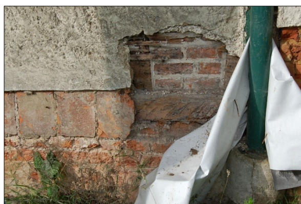
Photo 16: Detail of framing on eastern end of north elevation (G2)
