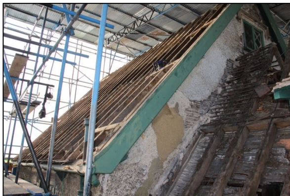
Photo 257: R23: Roof 6, facing southwest
