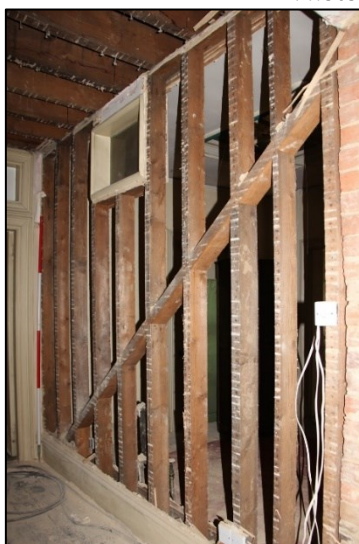
Photo F52: F8: east wall stripped
