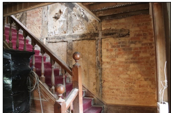
Photo G20: G1: west wall stripped
