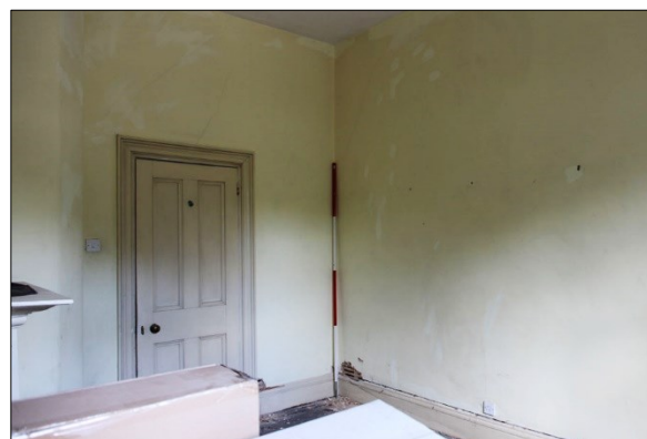
Photo F21: F3: south and west walls, facing southwest
