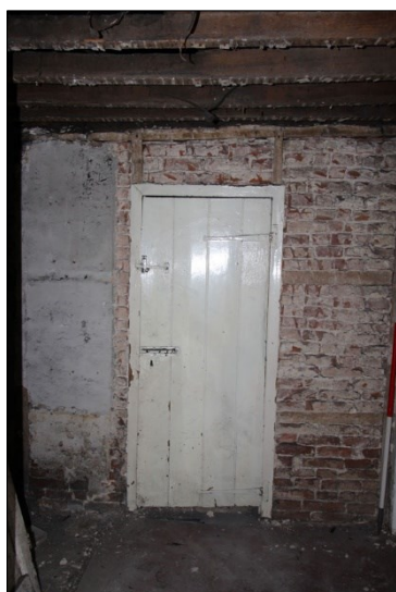
Photo G69: G10: east wall
