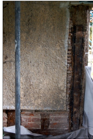
Photo 13: Detail of timberwork on northeast corner, G2
