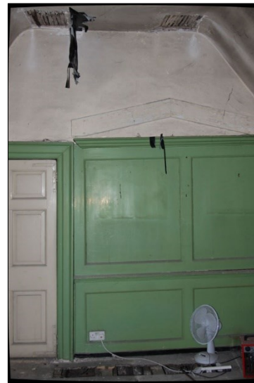
Photo F61: F11: south wall
