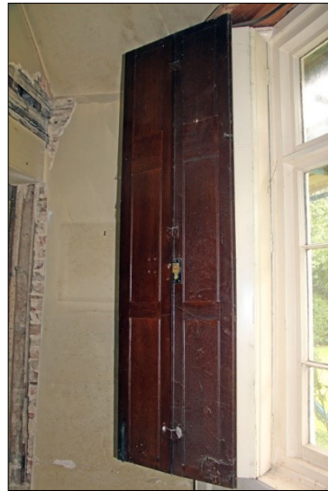
Photo G32: G2: Shutter detail in east bay
