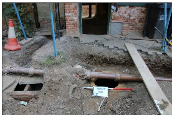
Plate 20: Dumb well and conduit from the west
