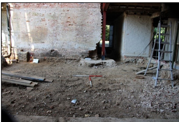
Plate 18: Ground reduction within the proposed conservatory from site east
