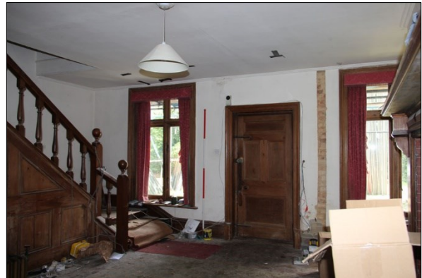
Photo G4: G1: north wall
