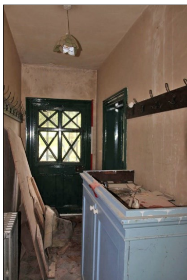
Photo G51: G5: Facing south, door to G6 on right, exterior door at end
