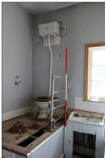
Photo F75: F13: southeast corner, facing southeast
