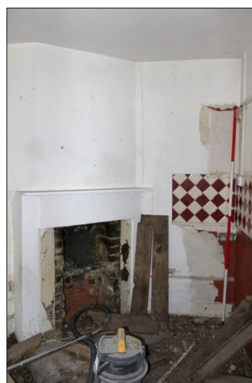
Photo G95: G16: east wall with corner fireplace
