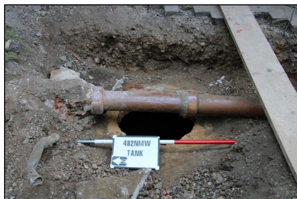
Plate 21: Detail of the dumb well
