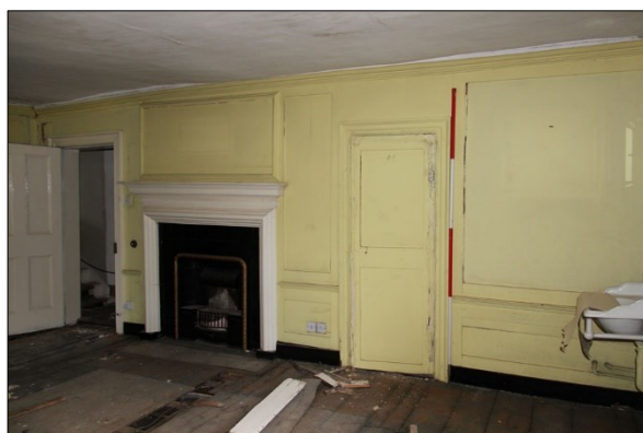
Photo F23: F4: west wall, door to right blocked with brick
