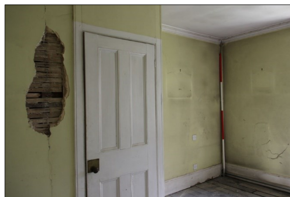
Photo F38: F5: north wall, facing northeast
