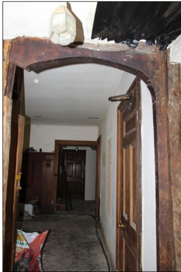
Photo G15: G1: detail of timber arch, facing west
