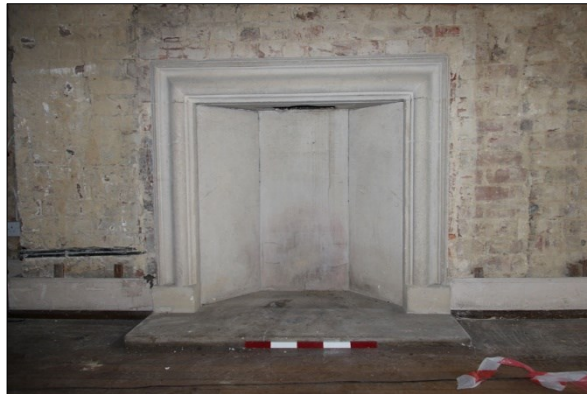
Photo G48: G4: fireplace detail
