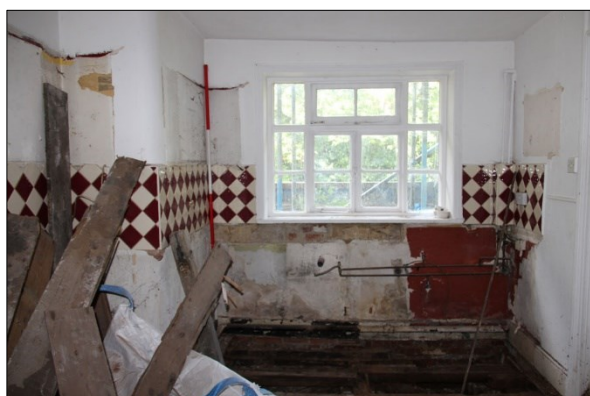
Photo G96: G16: west wall
