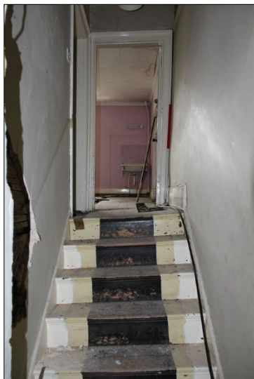
Photo F7: F1: stair up to F5 and F6
