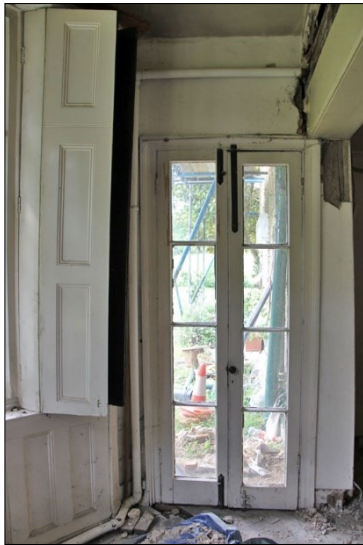
Photo G31: G2: French doors in bay, facing south
