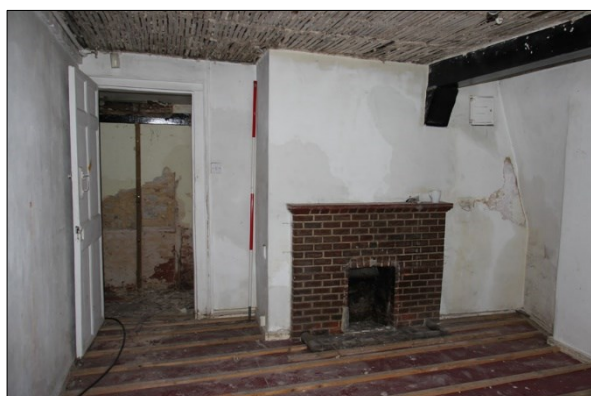
Photo G92: G15: east wall
