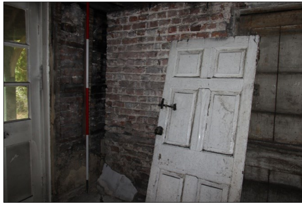
Photo G73: G10: northwest corner
