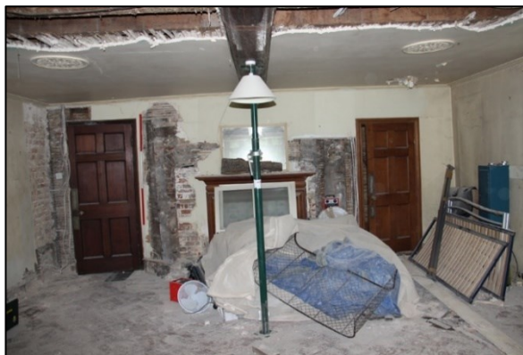
Photo G33: G2: West wall partially stripped
