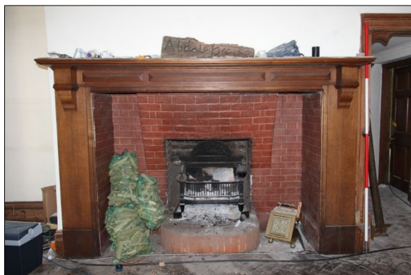
Photo G7: G1: detail of fireplace
