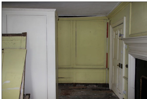
Photo F27: F4: west end of south wall
