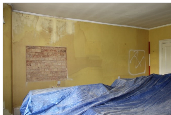
Photo F46: F7: west wall
