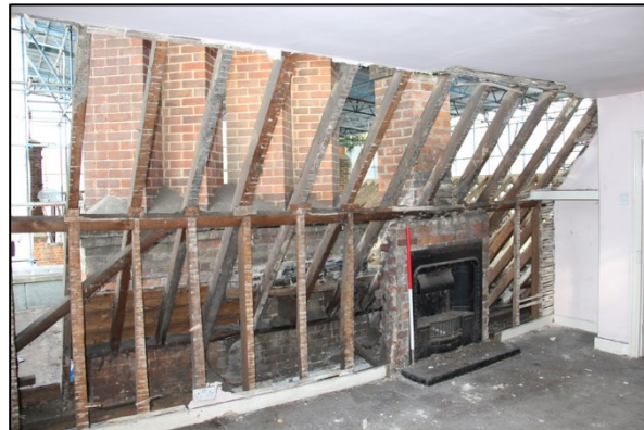
Photo S18: S5: west wall stripped
