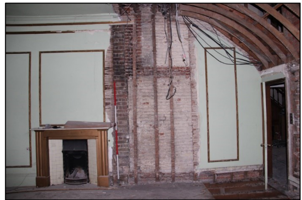
Photo G42: G3: West wall partially stripped
