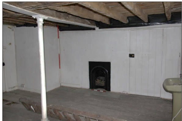
Photo F84: F15: south wall
