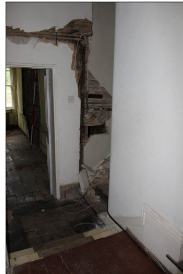
Photo F6: F1: east end of hall
