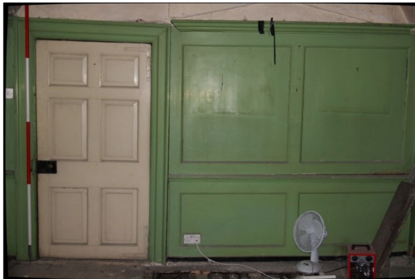
Photo F60: F11: south wall
