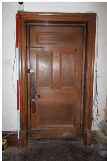
Photo G5: G1: detail of front door
