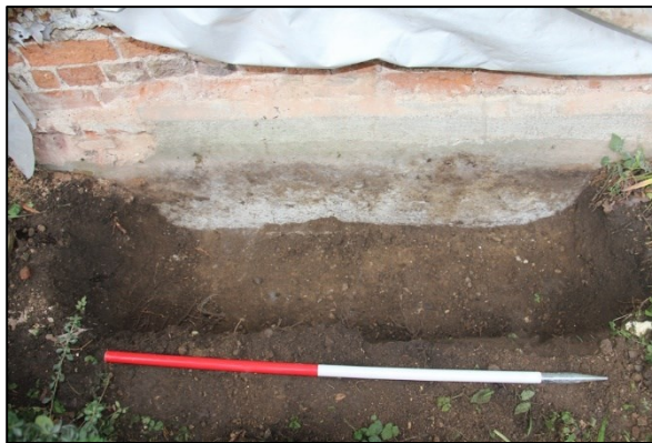
Plate 4: Concrete footing beneath G3
