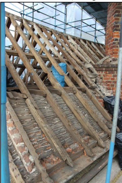
Photo 247: R13: Roof 5, facing northwest
