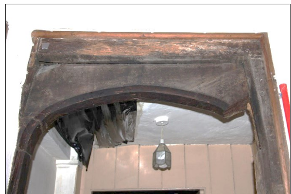
Photo G14: G1: detail of medieval timber arch
