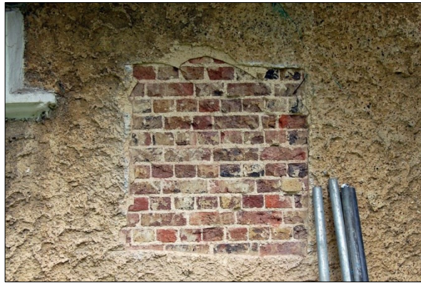
Photo 12: Detail of brickwork to north of French door
