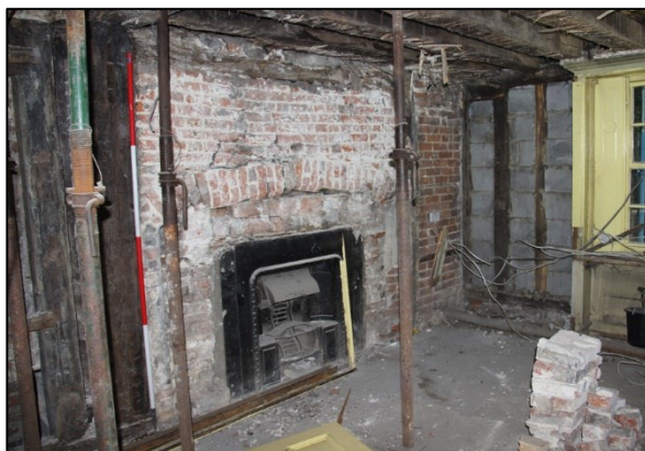
Photo G63: G8: northwest corner
