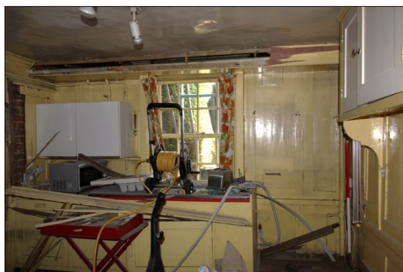
Photo G57: G8: north wall
