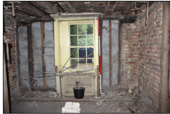
Photo G66: G8: north wall stripped
