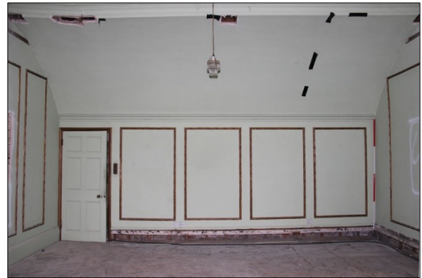
Photo G38: G3: North wall
