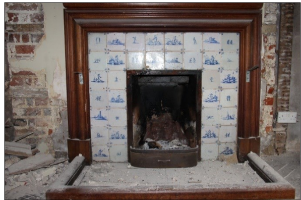
Photo G26: G2: Detail of fireplace, facing west
