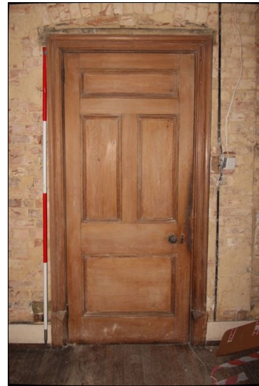
Photo G49: G4: detail of north door
