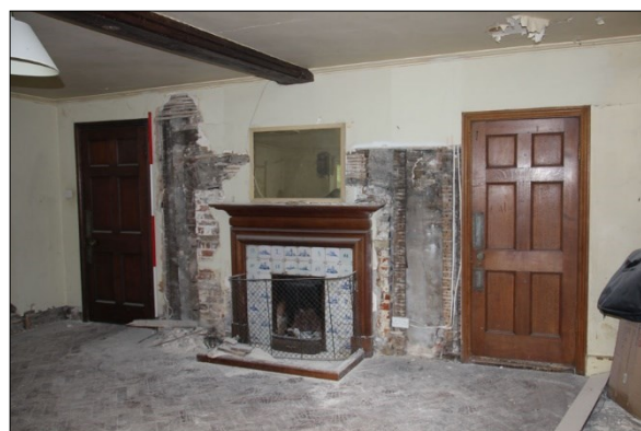
Photo G24: G2: West wall
