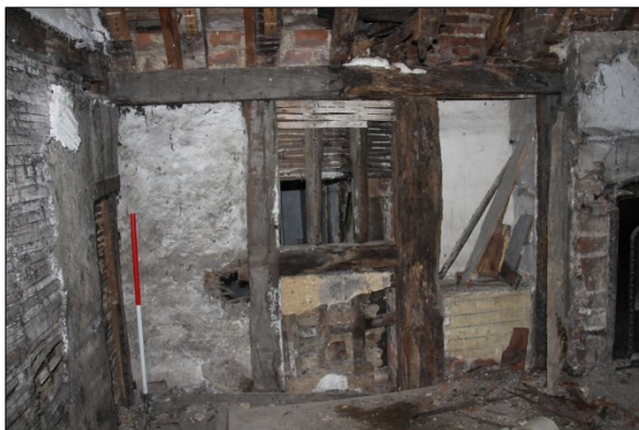
Photo F64: F11: exposed mullion window, wattle and daub on left below window
