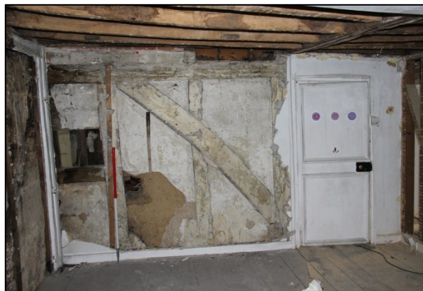
Photo F86: F15: east wall stripped
