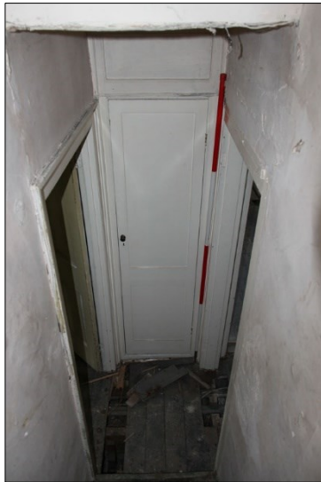
Photo F9: F1: landing between F5 and F6, facing south
