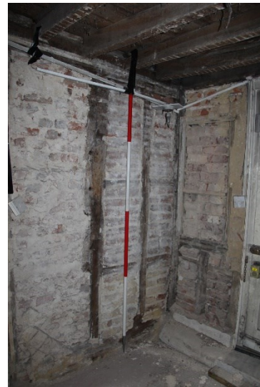
Photo G74: G10: northeast corner
