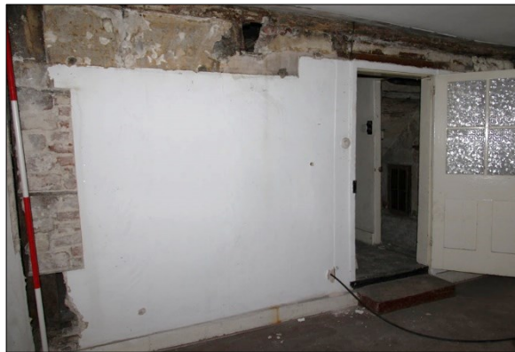
Photo G77: G11: east wall, facing southeast
