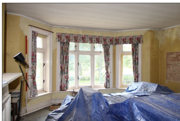
Photo F45: F7: south wall
