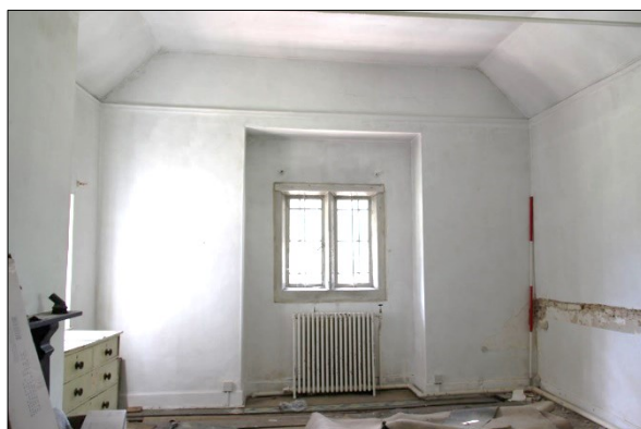
Photo F88: F16: south wall
