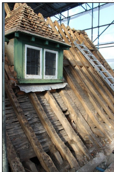
Photo 259: R25: Roof 6, facing northwest
