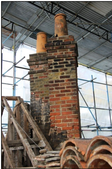
Photo 249: R15: Roof 5, facing northwest
