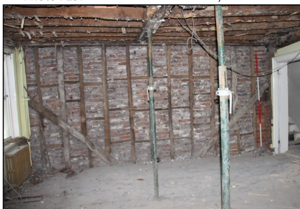
Photo F31: F4: south wall stripped
