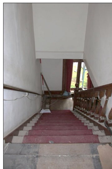
Photo F2: F1: view down staircase, facing north
