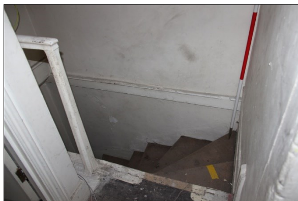
Photo F72: F12: back stair along south wall
