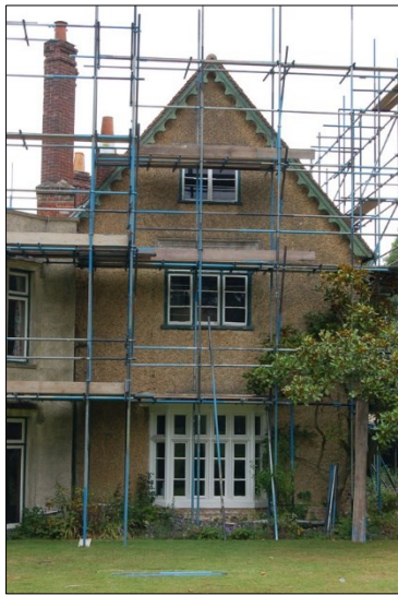
Photo 3: Eastern end of south elevation
