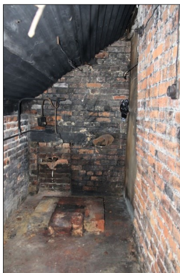
Photo G68: G9: Facing east
