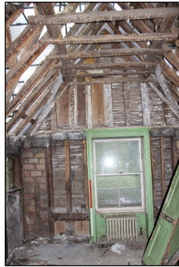
Photo F67: F11: north wall stripped
