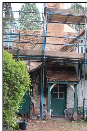
Photo 21: Entrance porch to Northside in northwest corner
