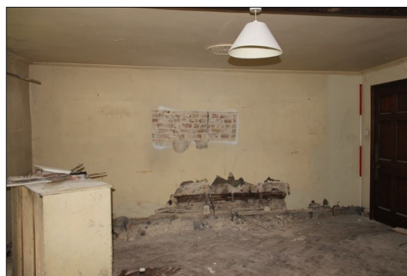
Photo G22: G2: South wall, facing south
