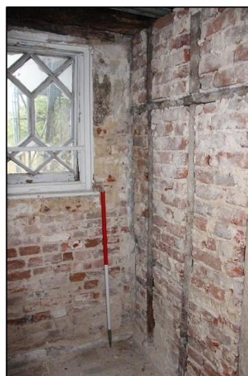
Photo G89: G14: southwest corner
