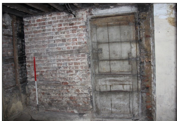
Photo G71: G10: north wall
