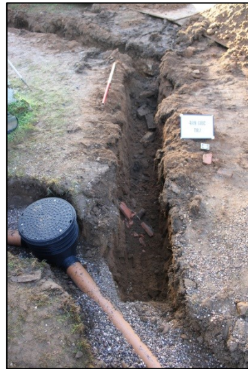
Plate 44: Trench 7, part 1, facing south
