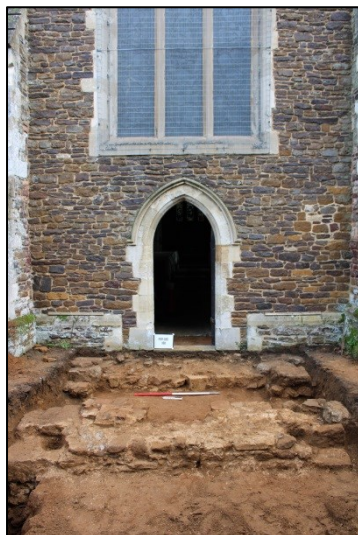
Plate 35: Church foundations [108], facing east
